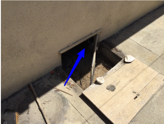
Rear unit crawlspace.
