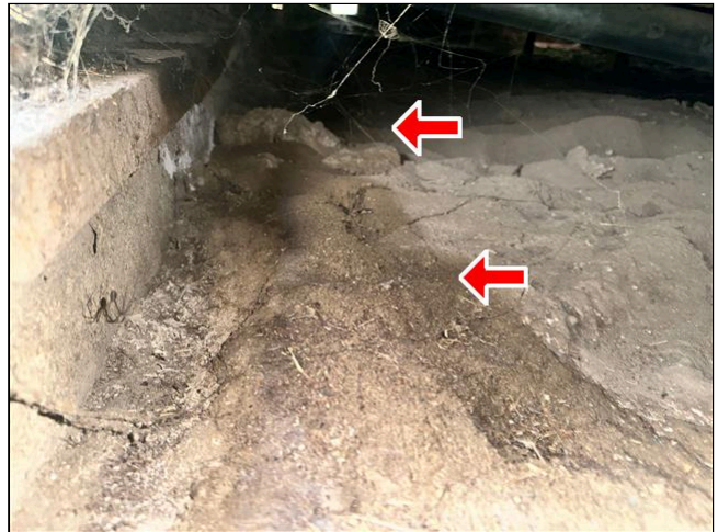
3.0 Item 3 (Picture) Structural Components
