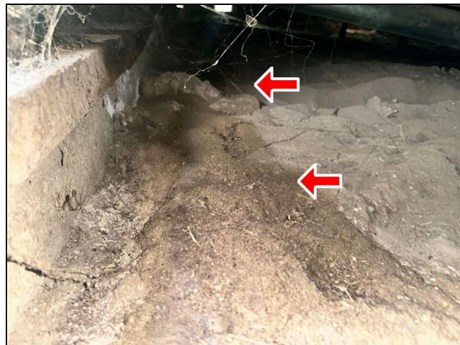
Item 4 - Item 2 (Picture) Structural Components
