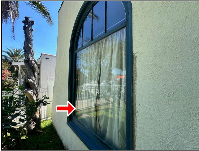
8.3 Item 1 (Picture) Interiors
