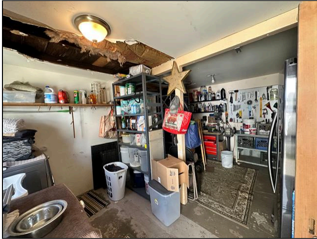
10.4 Item 2 (Picture) Garage
