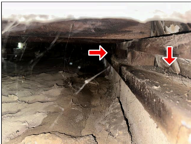
3.0 Item 1 (Picture) Structural Components
