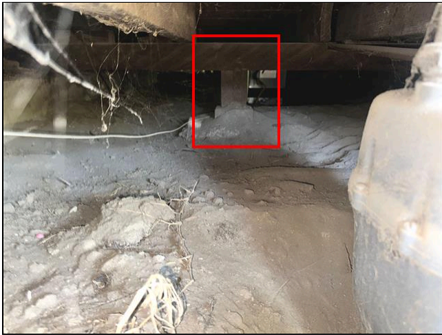
3.2 Item 1 (Picture) Structural Components
