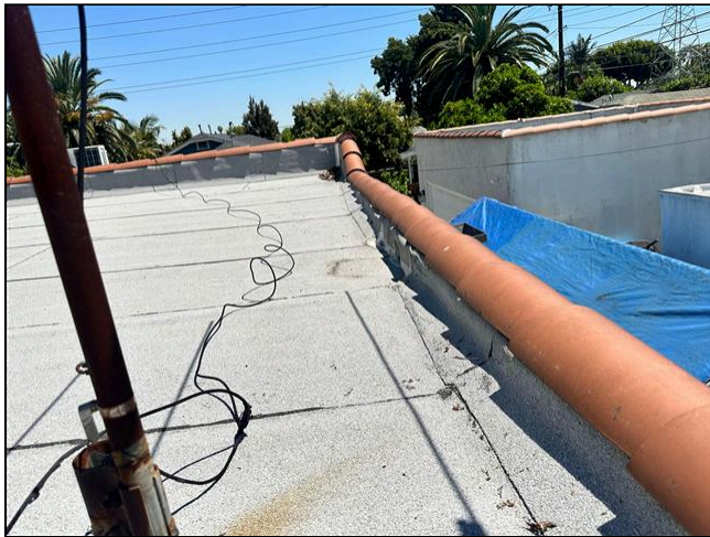
1.0 Item 3 (Picture) Roofing
