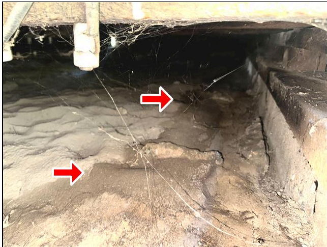
3.0 Item 2 (Picture) Structural Components
