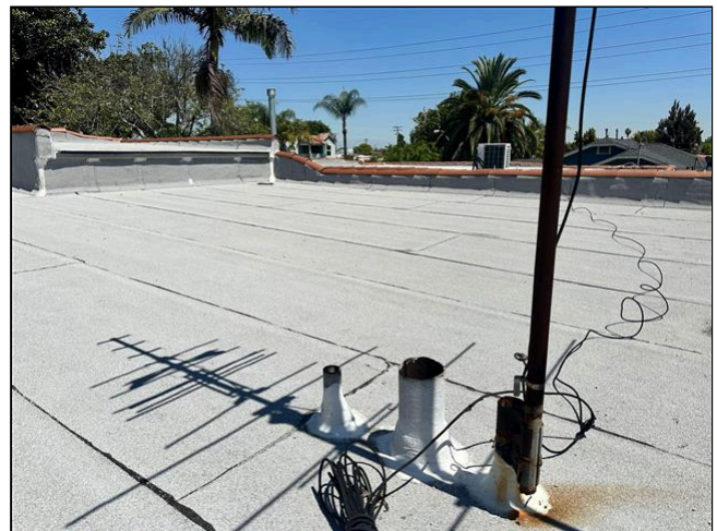
1.0 Item 2 (Picture) Roofing
