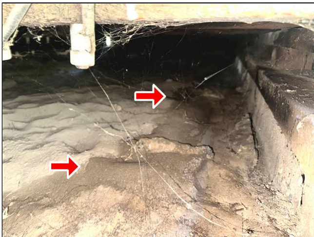
Item 4 - Item 1 (Picture) Structural Components
