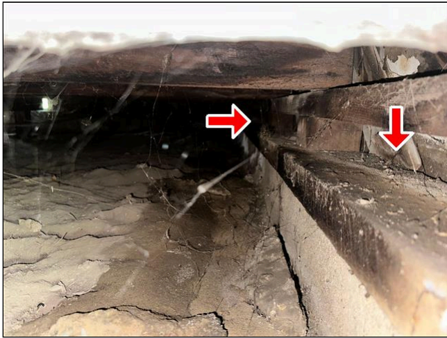
Item 3 - Item 1 (Picture) Structural Components
