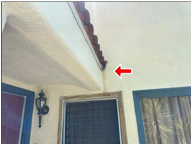
1.1 Item 1 (Picture) Roofing
