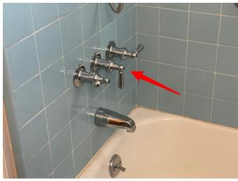
204: The hand sprayer leaks (repairs needed).
