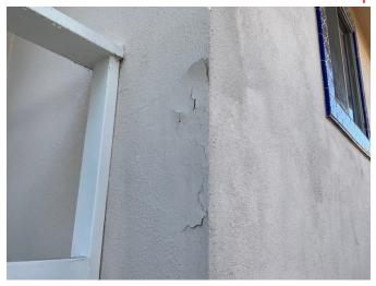
**20:** At some areas of the lower walls, the stucco and paint is cracked, thin, and degraded. This is likely from exposure to moisture in the soils and/or sprinkler overspray. The condition should be monitored but is currently considered cosmetic.
