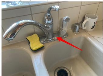
s-147: The sink faucet is leaking into the cabinet below.
