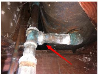
**s-203:** The shower diverter valve in the tub-shower is defective (repair or replacement needed).
