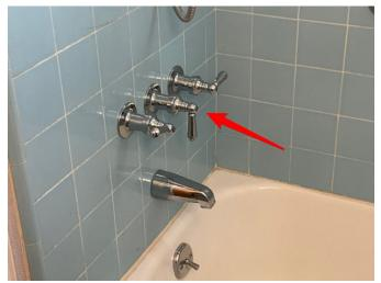
**s-204:** The hand sprayer leaks (repairs needed).
