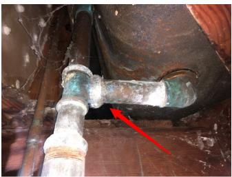
203: The shower diverter valve in the tub-shower is defective (repair or replacement needed).
