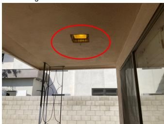
**32:** An approved weather-resistant cover is required at an open junction box located at the rear patio.
