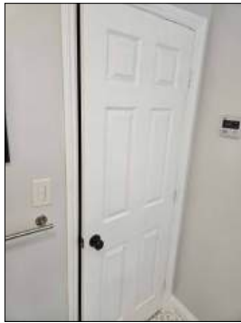
Sticks at jamb - recommend servicing - at master bathroom
