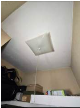
Light fixture did not function / pull chain stuck in position - recommend service - at bedroom closet northeast
