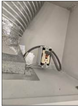
Missing outlet cover above microwave - recommend installation/replacement of all covers for safety
