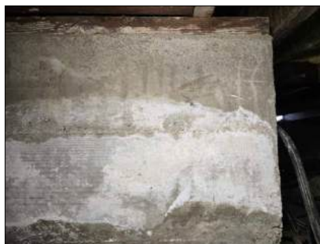
Efflorescence present - indicates past moisture accumulation - monitor for further moisture intrusion
