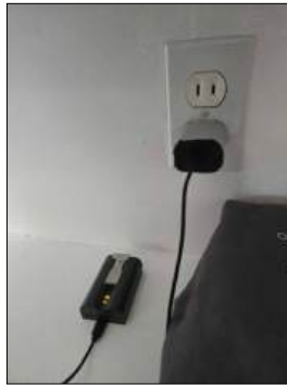
Ungrounded outlets present - typical for the age of the structure - consider upgrading electrical services
