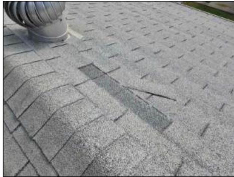
Missing/damaged shingles/tiles in areas - recommend servicing
