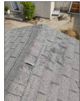
Missing/damaged shingles/tiles at ridge/hip - needs to be serviced
