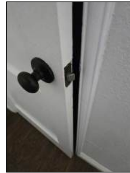
Closet door did not latch properly/hardware insalled backwards - service needed - at bedroom northeast
