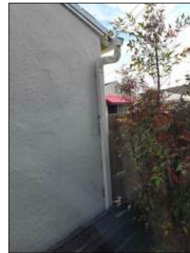
Tree touching against roof / structure - needs to be serviced
