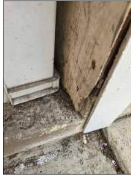
Deteriorated wood observed - recommend servicing
