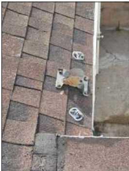
Satellite dish/brackets fastened directly to the roof - screws will need periodic sealant and maintenance to prevent possible damage or moisture intrusion
