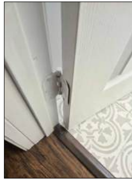
Loose hardware or hinges - needs to be serviced - at master bathroom
