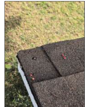
Exposed nails/staples/screws on roofing material - recommend sealing all fastener heads
