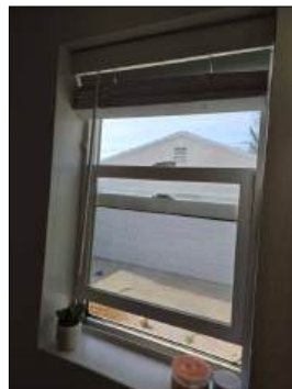
Loose/broken sash springs or cables - possible safety concern - recommend service - at bedroom southeast, master bathroom, living room
