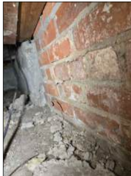
Brick at chimney hearth cracked/chipped/loose - loose/missing mortar - recommend service/further evaluation
