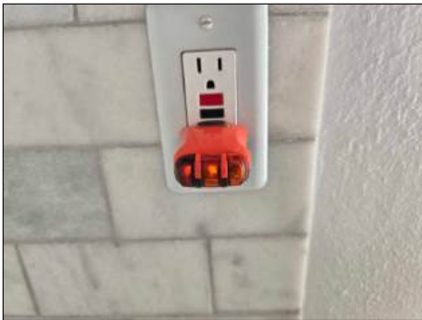
One GFCI outlet hot wired in reverse with neutral - recommend further evaluation by a licensed electrician
