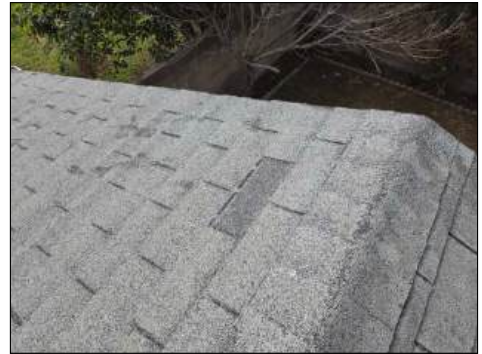
Missing/damaged shingles/tiles in areas - recommend servicing
