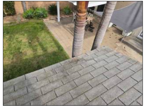
Tree touching against roof / structure - needs to be serviced
