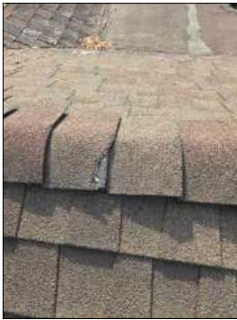
Missing/damaged shingles/tiles at ridge/hip - needs to be serviced
