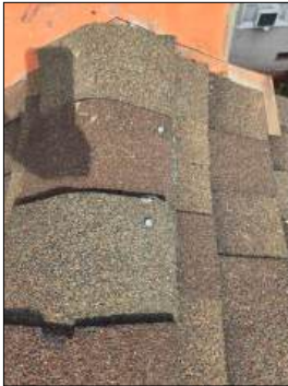
Exposed nails/staples/screws on roofing material - recommend sealing all fastener heads
