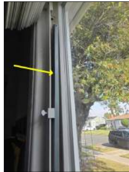
Loose/broken sash springs or cables - possible safety concern - recommend service - at bedroom southeast, master bathroom, living room
