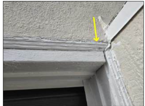
Deteriorated wood at jamb - needs to be serviced
