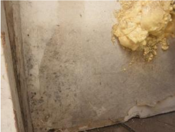
Black mildew like substance on the drywall inside the water heater closet.
