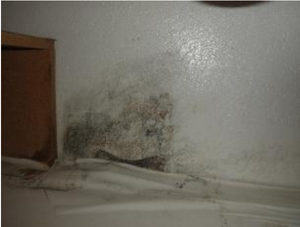
Black mildew like substance under the half bathroom sink.
