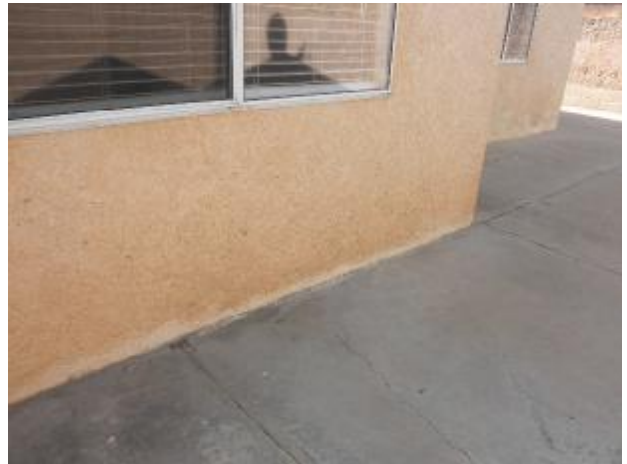
The concrete walkways and patios embed the weep screed at the base of the stucco walls.
