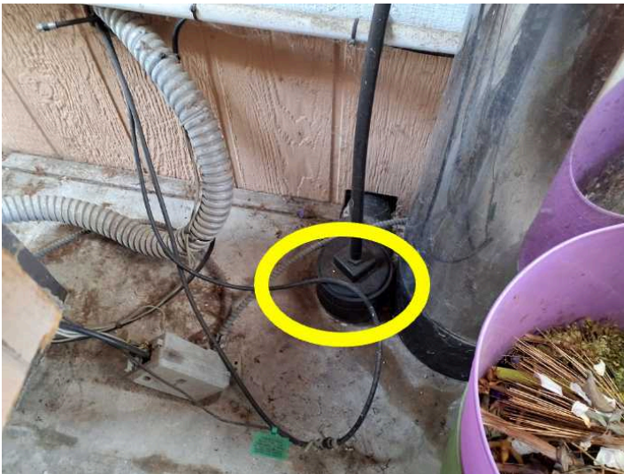
A clean-out is located at the right side.
