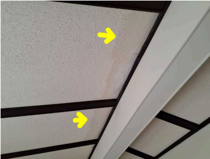
There has been a drywall/plaster repair that should be explained by the seller.
