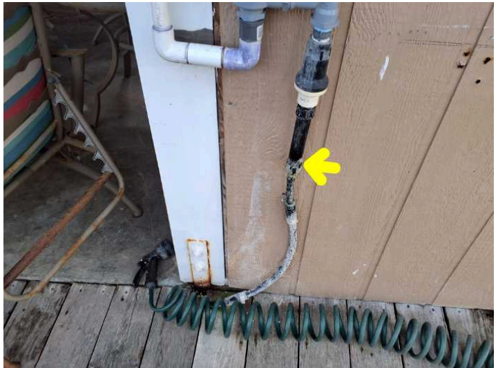
A sprinkler valve, fitting, or pipe located at the right side is leaking and should be repaired by a qualified specialist.
