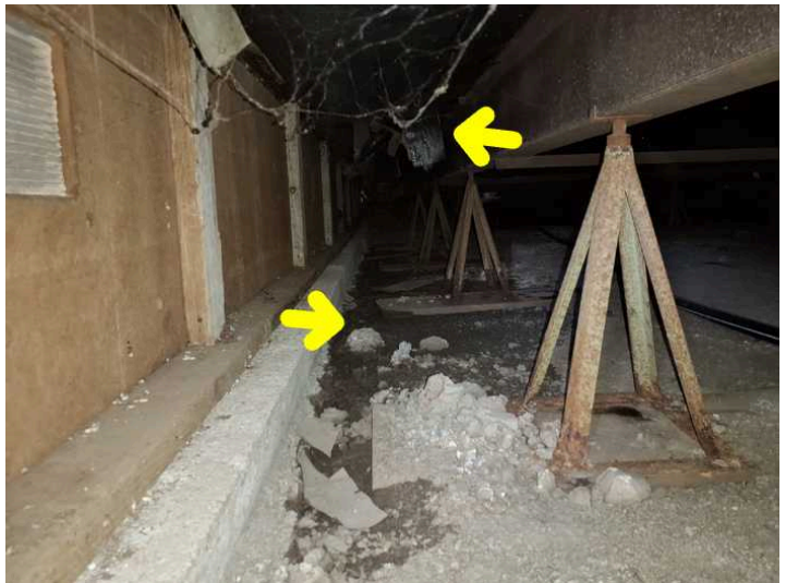
There is a drainpipe leak in the foundation area, below the kitchen, which should be repaired by a qualified tradesperson.
