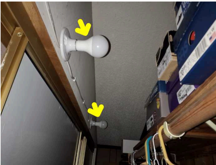
The closet light is missing its globe or cover, which should be installed to improve safety.
