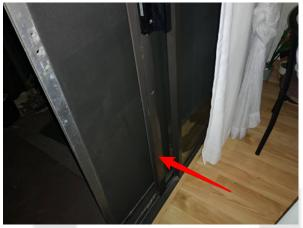
**42:** The sliding screen door is damaged. We recommend it be repaired or replaced.
