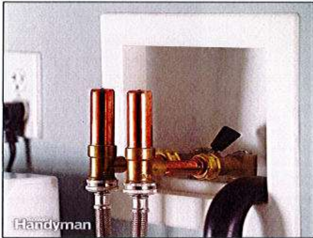
6.5 Item 1 (Picture) HV
