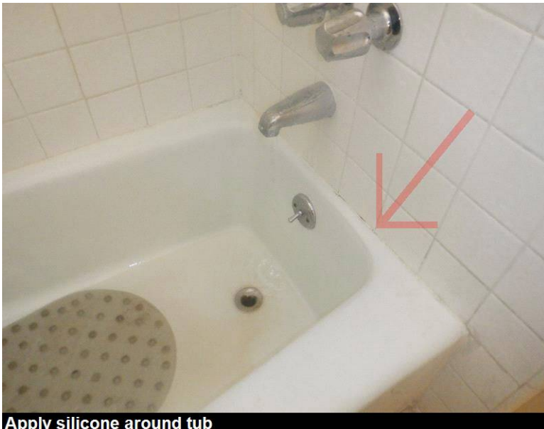
Apply silicone around tub
