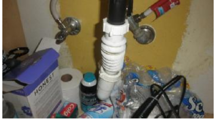
Corrugated piping at the hall bathroom sink.
