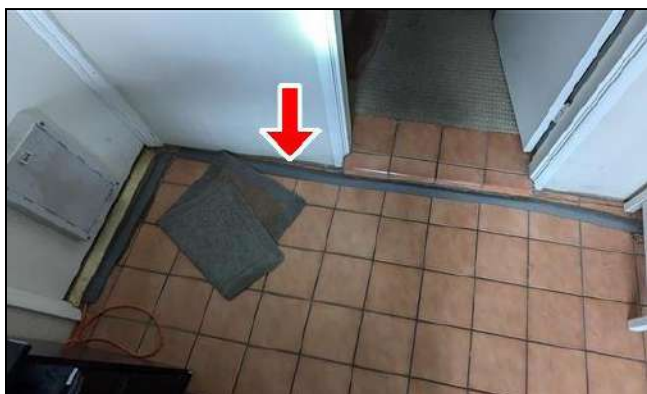
7.4 Item 5 (Picture) Foyer - Cord protectors noted from extension cabling. Suggest adding receptacles/outlets where needed for improved safety.
