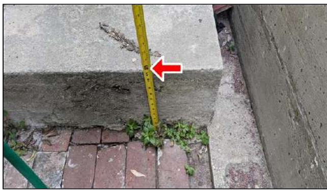
2.3 Item 2 (Picture) Close-up of Item 1 - Riser height at first step is higher than 7.5" maximum
