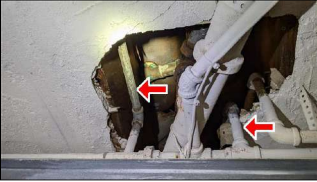
6.0.A Item 3 (Picture) Galvanized supply piping noted, view from Garage
