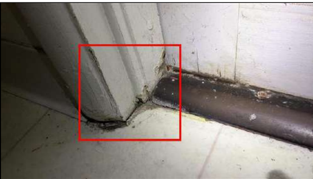
6.4.B Item 3 (Picture) Staining noted at lower portion of Rear entryway door frame
