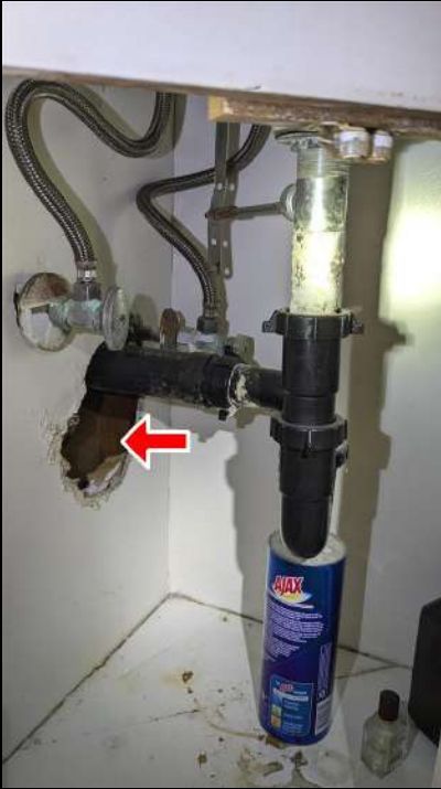
6.0.B Item 5 (Picture) Recommend repairs/sealing at wall penetration.
