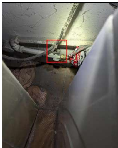
6.4.A Item 5 (Picture) Grease pack valve noted.
