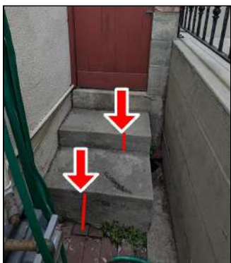
2.3 Item 1 (Picture) Exterior steps are not uniform, which may present a trip hazard
