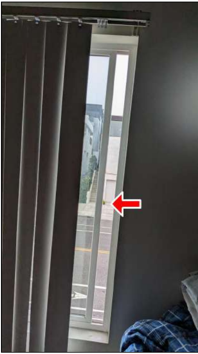
4.4 Item 9 (Picture) SE Bedroom (2nd Floor) - No window screen noted. Suggest adding window screen to prevent insect pest intrusion.
