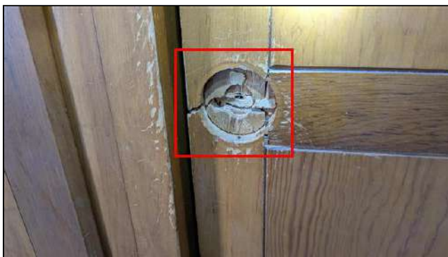
4.5 Item 3 (Picture) SE Bedroom (2nd Floor) - Cracking/wear noted at closet door with missing pull hardware. Suggest repairs.
