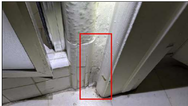
6.4.B Item 4 (Picture) Repairs, possible moisture damage noted by shower stall
