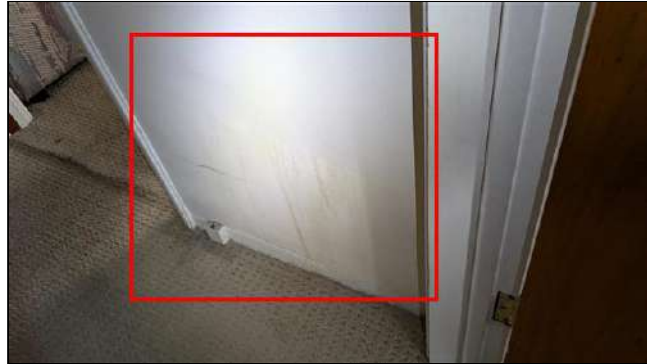
4.0 Item 17 (Picture) 2nd Floor Hallway - Repairs and staining noted at wall
