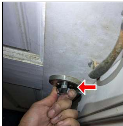
2.2 Item 4 (Picture) Rear Entryway Door - Dead bolt did not turn easily. Recommend adjustments/repairs for smooth operation.
