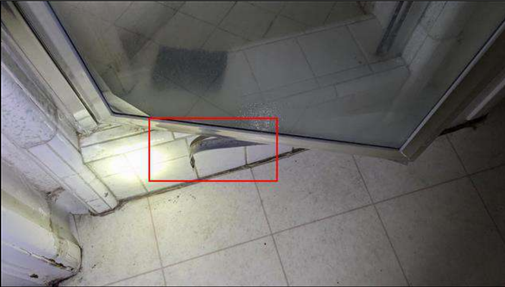
6.2.B Item 4 (Picture) Wear noted at shower door sweep. Recommend replacement to prevent water seepage while bathing
