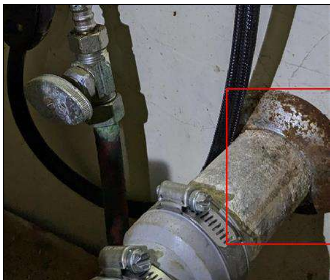
10.0 Item 8 (Picture) Corrosion noted
