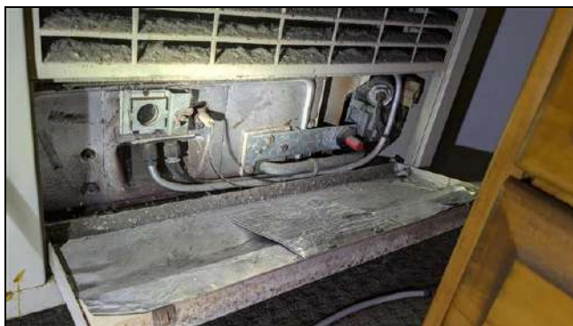
8.1 Item 3 (Picture) First Floor Bedroom - Direct Vent Heating Unit
