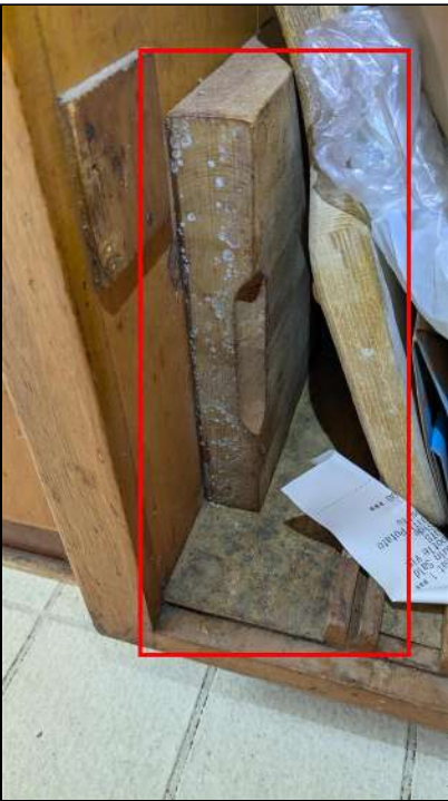
10.6 Item 11 (Picture) Discoloration, possible mold growth noted
