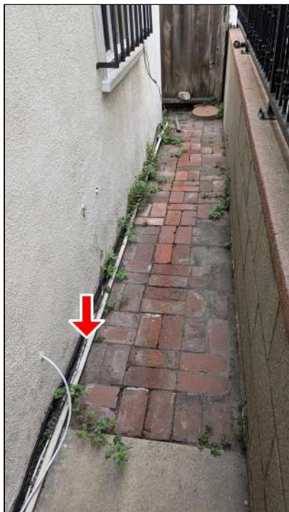
6.5.A Item 2 (Picture) Gas piping noted low, in direct contact with pavement.
