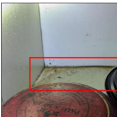
10.6 Item 10 (Picture) Discoloration, possible mold growth noted
