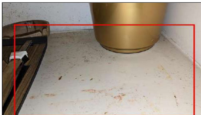
10.6 Item 4 (Picture) Discoloration, possible mold growth noted
