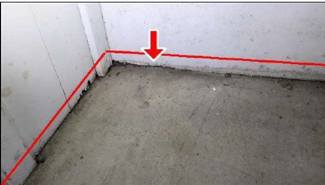
3.2 Item 17 (Picture) Staining/moisture damage noted at lower portions of drywall, rear garage area
