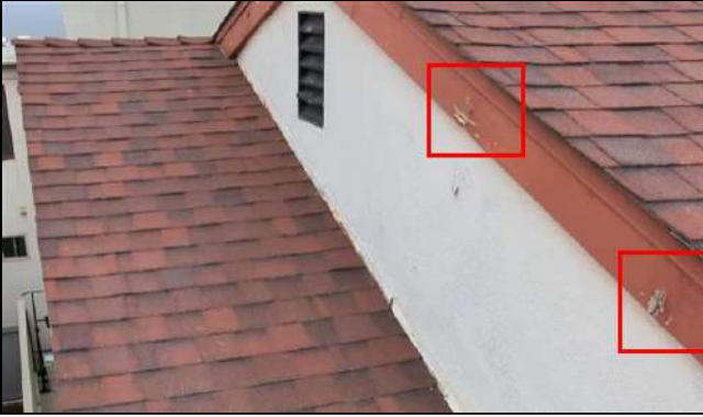
1.4 Item 1 (Picture) Peeled paint/wear noted
