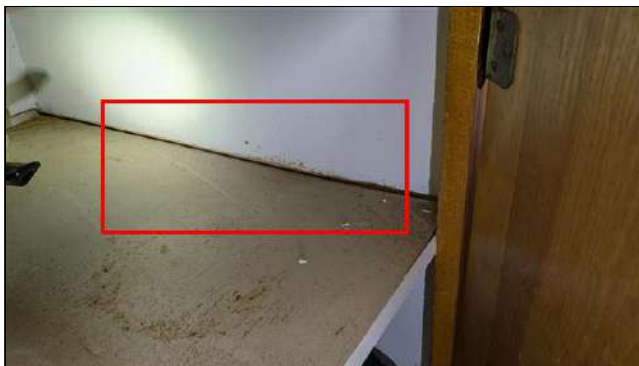
10.6 Item 8 (Picture) Discoloration, possible mold growth noted
