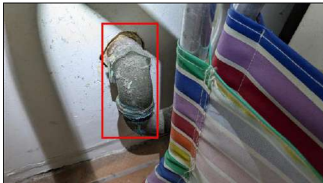
6.4.A Item 2 (Picture) Laundry Room - Wear, corrosion noted at drain piping. Recommend monitoring over time and repairs as needed to prevent leaks
