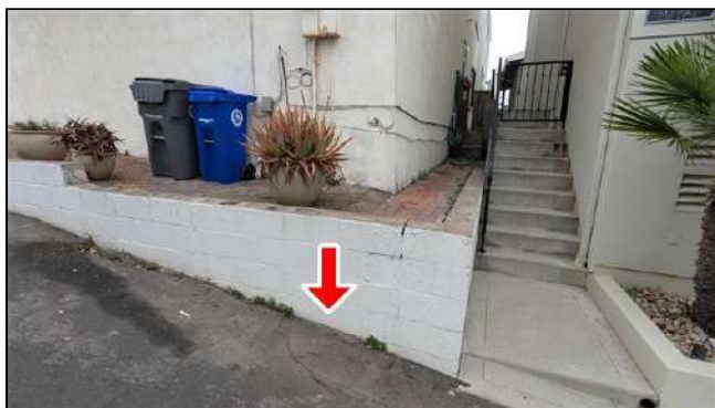
2.5 Item 3 (Picture) No weep holes and no built-in drainage was observed at retaining walls
