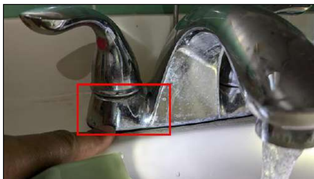
6.0.C Item 2 (Picture) Leak noted at faucet hardware.
