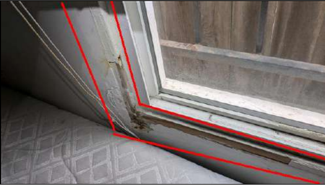
4.4 Item 1 (Picture) First Floor Bedroom - Staining/moisture damage noted at window frame.
