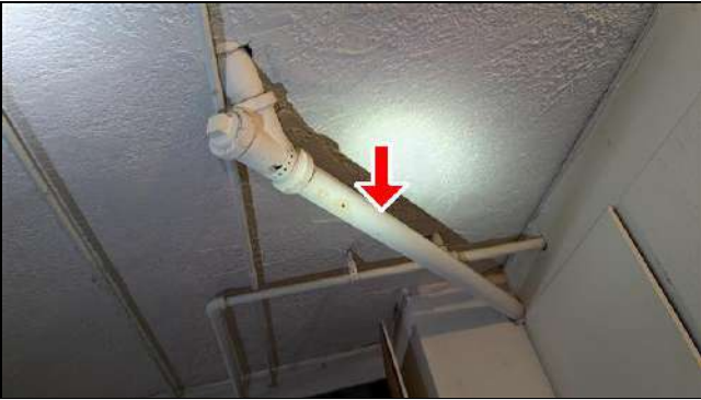
6.1.A Item 7 (Picture) Garage - Older drain piping noted
