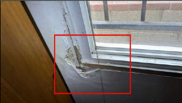
4.4 Item 3 (Picture) First Floor Bedroom - Staining/moisture damage noted at window frame.
