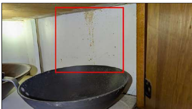
10.6 Item 9 (Picture) Discoloration, possible mold growth noted
