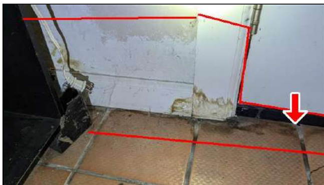
4.0 Item 7 (Picture) Foyer: Repairs noted with staining observed by front entryway door
