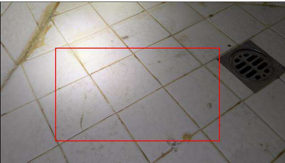
6.2.B Item 10 (Picture) Wear/fissures noted at tiles by drain
