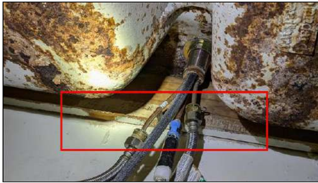
10.0 Item 4 (Picture) Staining noted under countertop behind sink basins
