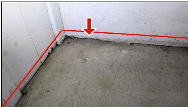
3.1 Item 5 (Picture) Staining/moisture damage noted at lower portion of drywall
