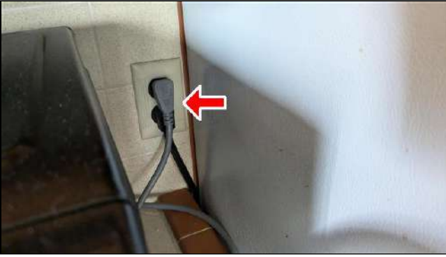
7.3 Item 3 (Picture) Kitchen - Countertop outlets, Not GFCI. The outlets also produced a buzzing sound whenever the garbage disposal was activated.
