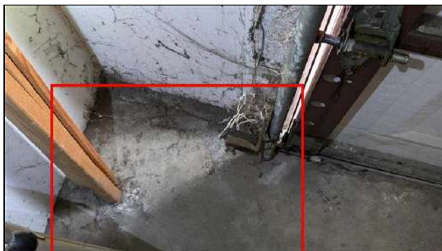
3.1 Item 3 (Picture) Staining/efflorescence noted by vehicle door
