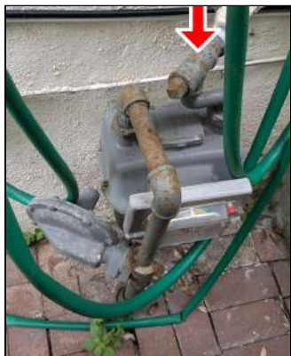
6.5.A Item 1 (Picture) No seismic shut-off valve noted downstream of gas meter
