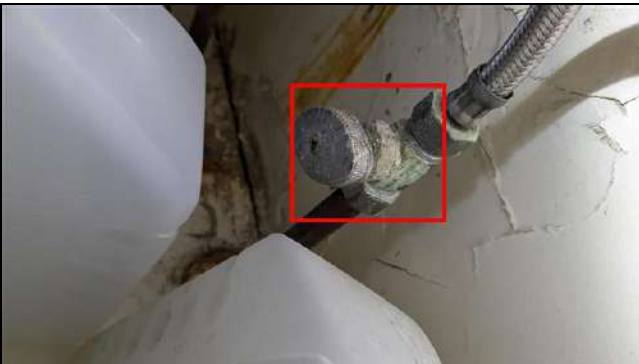
6.0.C Item 6 (Picture) Corrosion noted at angle stop valve
