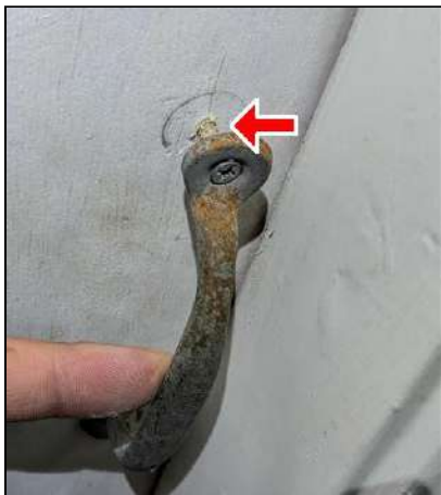
2.2 Item 5 (Picture) Rear Entryway Door - Loose handle noted. Suggest repairs.
