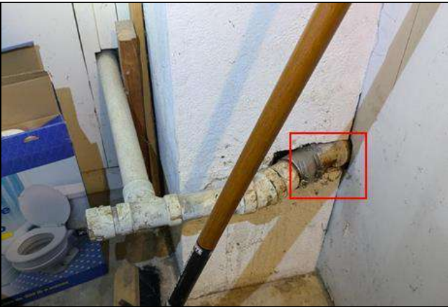
6.1.A Item 8 (Picture) Garage - Corrosion noted at drain piping.
