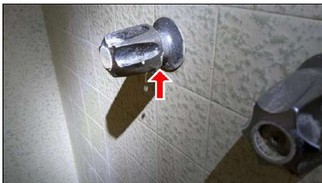
6.2.B Item 16 (Picture) Leaking noted at hot water handle
