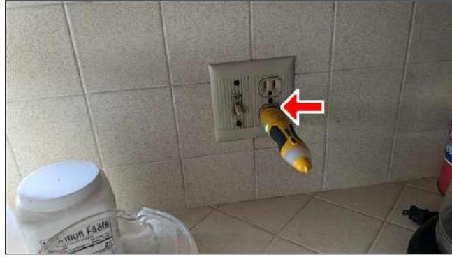
7.3 Item 4 (Picture) Kitchen countertop outlets, Not GFCI
