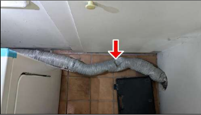
6.4.A Item 6 (Picture) Laundry Room - Flex dryer ducting has kinks. Recommend repairs/replacement to prevent lint clogs
