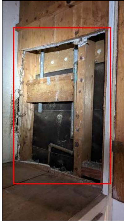
3.2 Item 9 (Picture) Breaches noted at wall within rear cabinet
