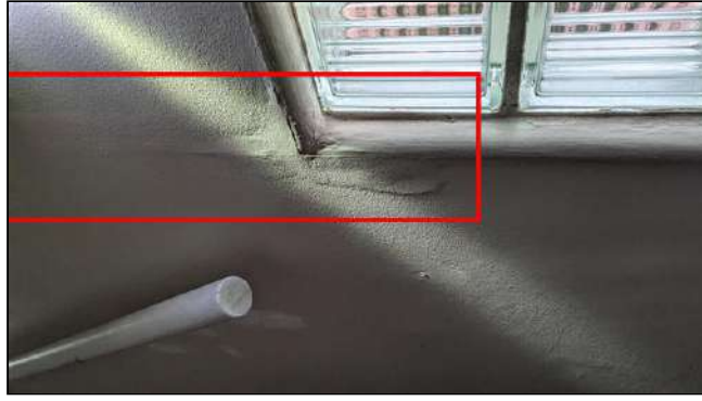
4.0 Item 4 (Picture) Crack/repairs noted by stairway window.
