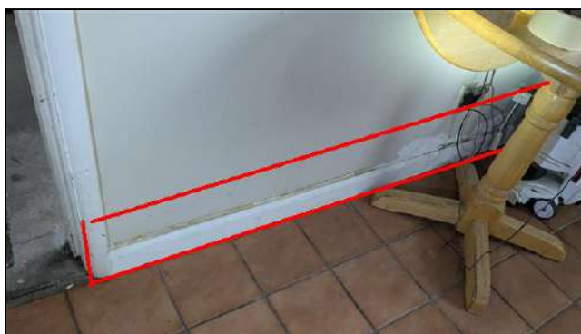
4.0 Item 10 (Picture) Foyer: Area of concern - Repairs and staining noted at lower portion of walls to left of Item 9
