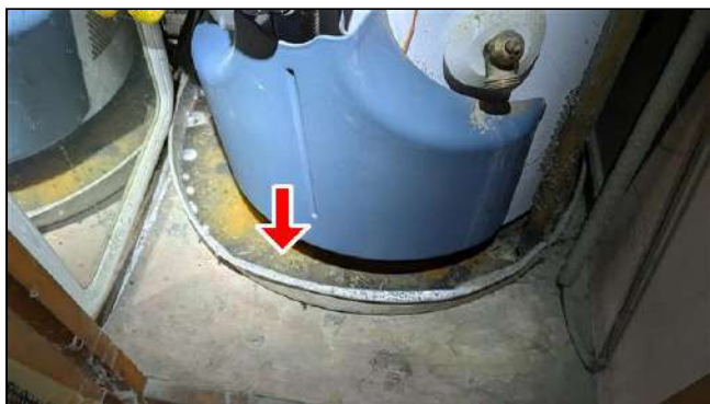
6.6.A Item 3 (Picture) Water noted at overflow pan
