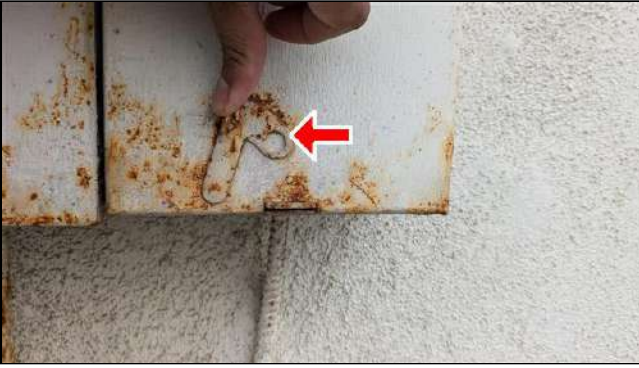
7.2 Item 7 (Picture) Unable to operate latch to secure exterior coverplate due to rust.
