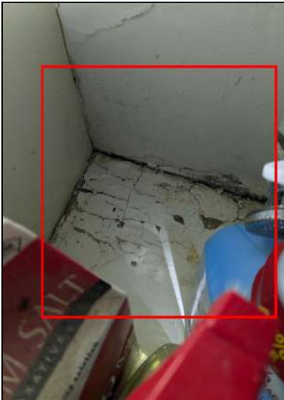
6.0.C Item 7 (Picture) Moisture damage, discoloration, possible mold growth noted.
