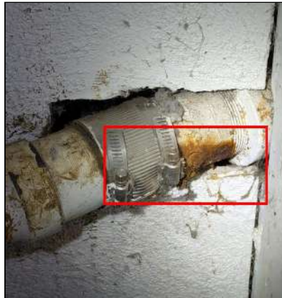
6.1.A Item 9 (Picture) Garage - Corrosion noted at drain piping
