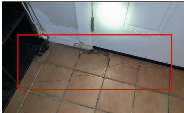
4.1 Item 2 (Picture) Foyer - Cracked tiles noted by front entryway door. Recommend grout repairs/tile replacement as needed to prevent moisture penetration.
