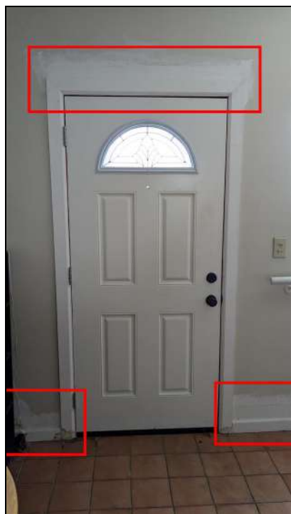
4.0 Item 1 (Picture) Patching/repairs noted by front entryway door
