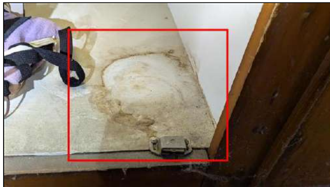
6.6.A Item 9 (Picture) Staining noted below water heater cabinet.
