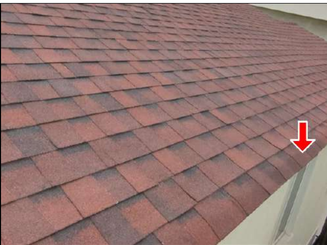
1.0 Item 5 (Picture) Shingles were installed with overhang at W side.
