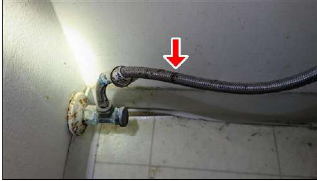
6.1.B Item 2 (Picture) Corrosion noted at steel-braided connector. Recommend repairs/replacement to prevent leaks.
