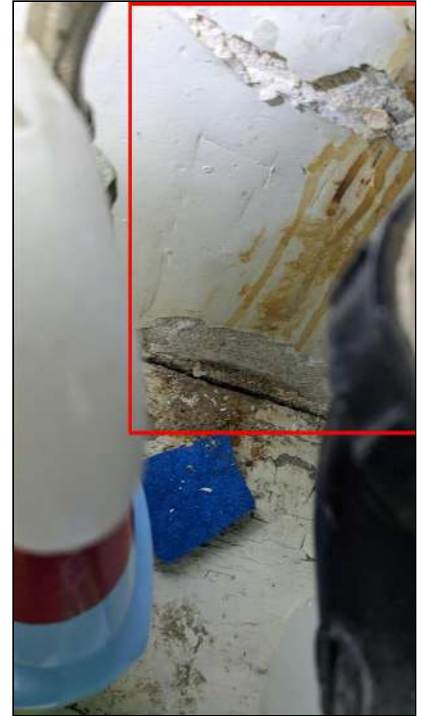
6.0.C Item 5 (Picture) Staining/moisture damage noted
