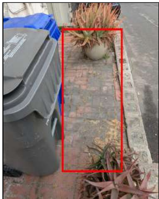
2.6 Item 1 (Picture) Area of drainage concern - No subsurface drainage was observed at walkway
