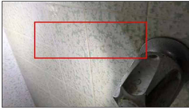
6.2.B Item 8 (Picture) Cracked tiles noted
