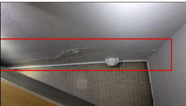
4.0 Item 13 (Picture) First Floor Bedroom - Blistering noted at lower portion of wall
