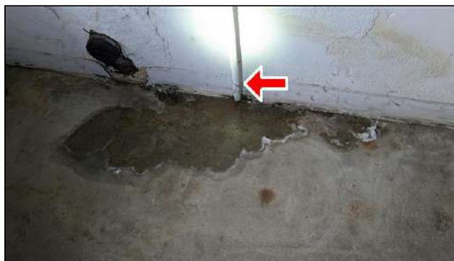
6.6.A Item 4 (Picture) Water noted at garage area. Recommend repairs to extend overflow drain piping to terminate at exterior to prevent water damage at interior building materials
