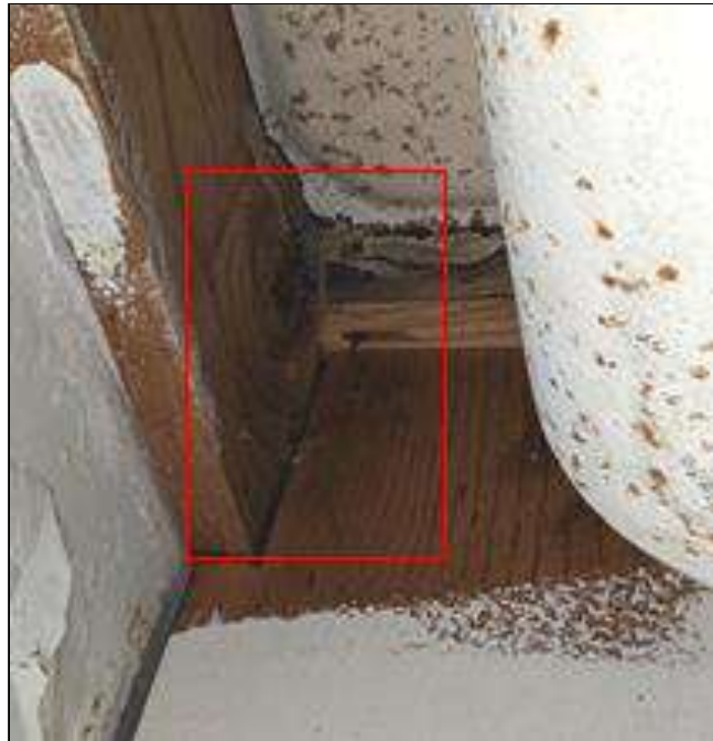
10.0 Item 6 (Picture) Staining noted under countertop behind sink basins
