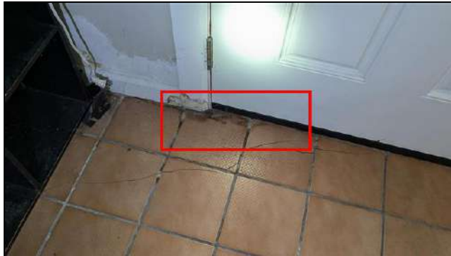
2.2 Item 2 (Picture) Staining noted by front entryway door
