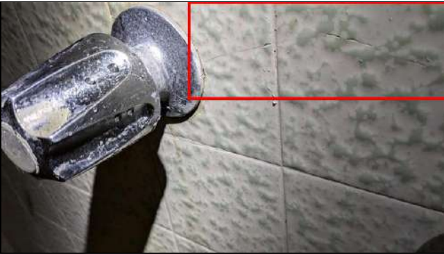
6.2.B Item 9 (Picture) Cracked tiles noted.
