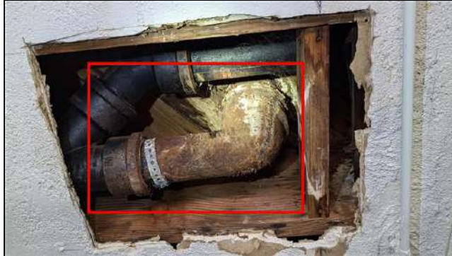
6.1.A Item 4 (Picture) Older/worn, cast-iron drain-waste piping noted under Shared Bathroom (2nd Floor), view from Garage. Signs of leaking were observed.
