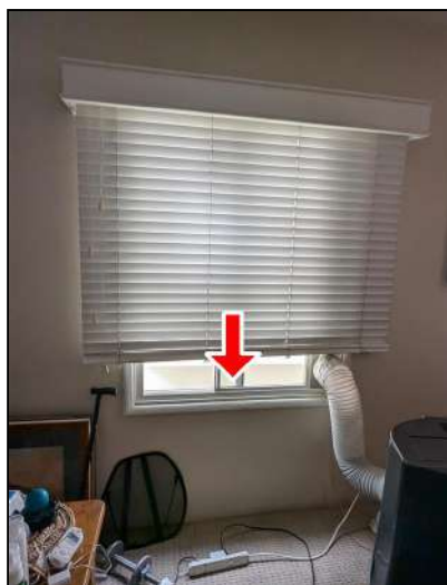
4.4 Item 12 (Picture) Living Room (2nd Floor) - Openable window has sill height less than 42"
