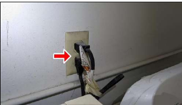
7.3 Item 1 (Picture) Laundry area outlets, Not GFCI
