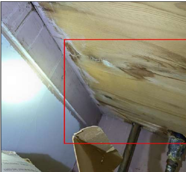
6.6.A Item 8 (Picture) Staining noted under platform
