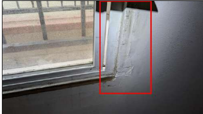
4.4 Item 4 (Picture) First Floor Bedroom - Staining/moisture damage noted at window frame.
