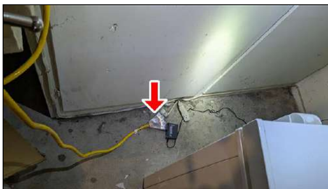
7.4 Item 4 (Picture) Garage - Extension cord cabling noted in garage area. Suggest further evaluation and repairs (i.e. adding outlets/ receptacles at garage) as needed for improved functionality/accessibility.
