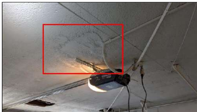
3.2 Item 4 (Picture) Patching/repairs noted.
