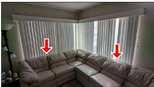
4.4 Item 11 (Picture) Living Room (2nd Floor) - Openable windows have sill heights less than 42"
