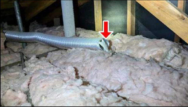
9.2 Item 1 (Picture) Shared Bathroom (2nd Floor) exhaust vent ducting terminates in attic area
