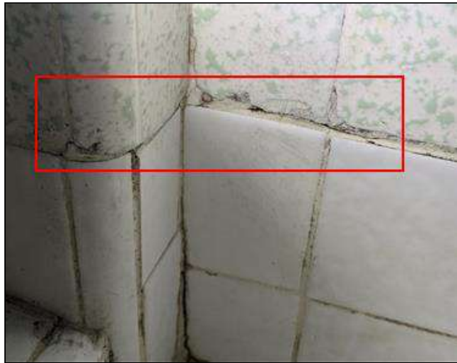
6.2.B Item 12 (Picture) Cracking/wear noted at grout
