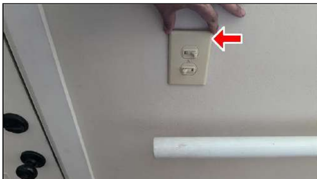
7.3 Item 8 (Picture) Foyer - Loose light switch noted. Recommend repairs.
