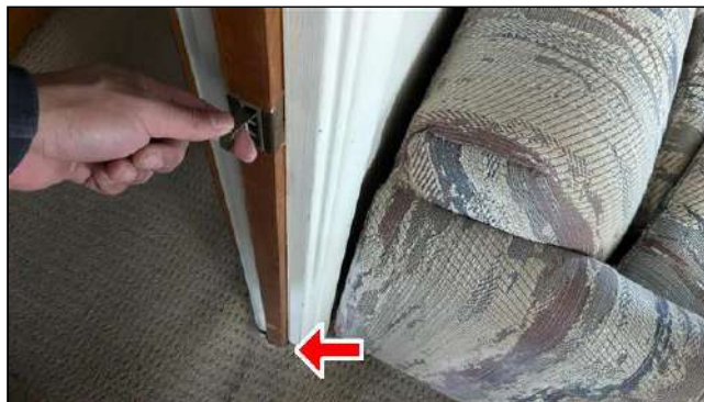
4.5 Item 2 (Picture) Pocket door at 2nd Floor hallway area does not open easily and snags on carpet. Suggest repairs.
