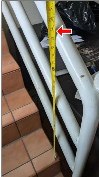
4.3 Item 2 (Picture) Hand railing is less than 34-36" high
