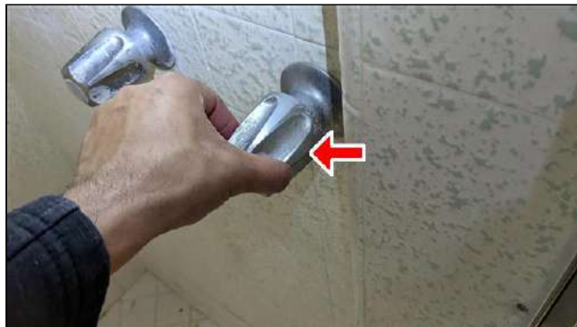
6.2.B Item 15 (Picture) Cold water handle was stiff and did not turn on.
