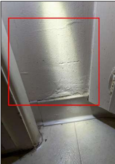
6.4.B Item 5 (Picture) Blistering/repairs noted.
