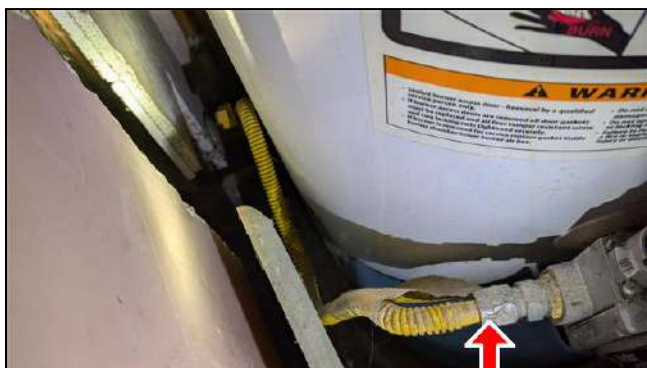
6.8.A Item 1 (Picture) No sediment trap noted.
