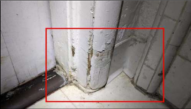
6.4.B Item 1 (Picture) Staining/moisture damage noted at lower portion of wall by shower stall and rear entryway door.
