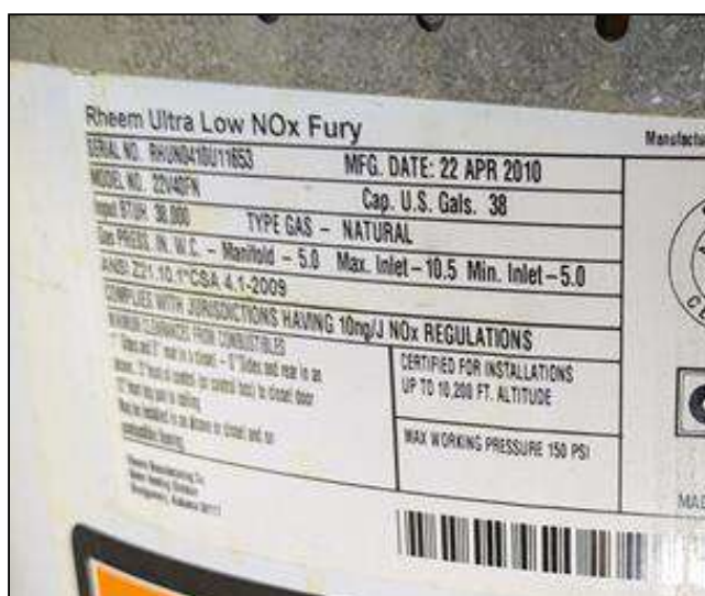
6.6.A Item 2 (Picture) Water Heater is older than 10 years
