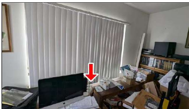
4.4 Item 14 (Picture) NE Bedroom (2nd Floor) - Openable window has sill height less than 42"
