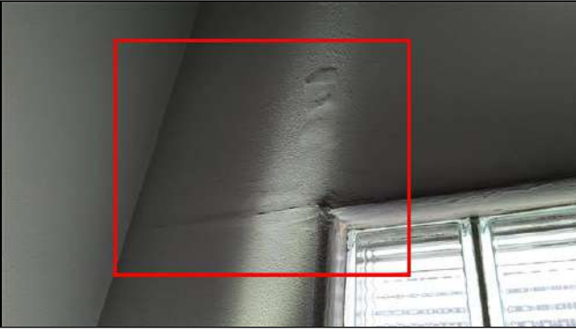
4.0 Item 3 (Picture) Crack/repairs noted by stairway window.
