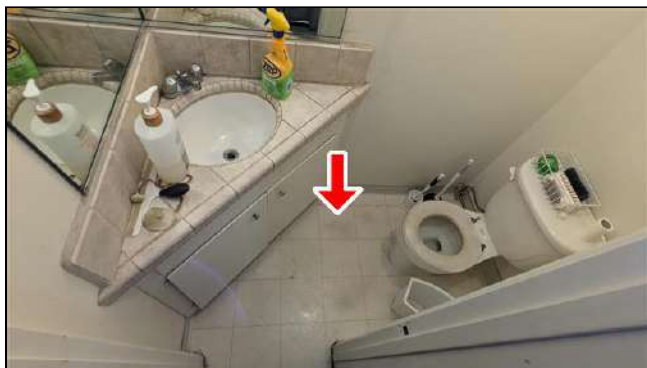
6.3.B Item 1 (Picture) Rolled vinyl flooring noted. Unable to determine age. Note that older vinyl flooring from before 1984 may contain asbestos in the flooring materials and/ or the adhesive.
