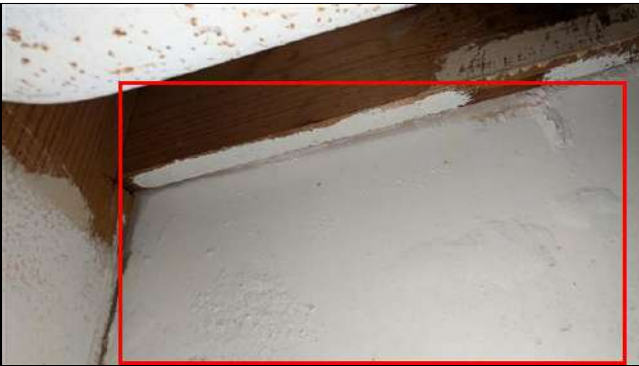
10.0 Item 5 (Picture) Blistering, possible moisture damage noted.
