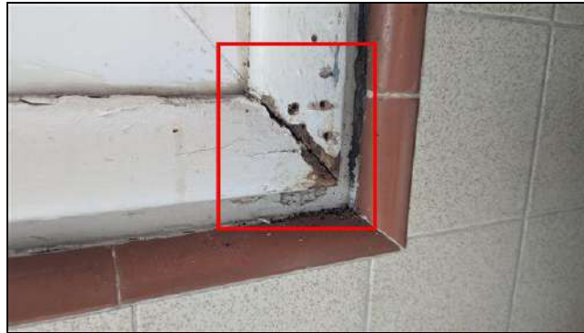
4.4 Item 8 (Picture) Kitchen - Wear, possible wood damage noted at window frame
