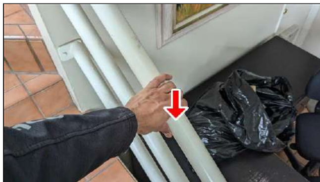
4.3 Item 4 (Picture) Hand railing is loose. Recommend repairs.
