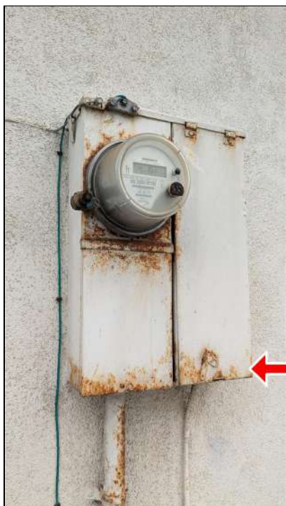
7.2 Item 1 (Picture) Rust noted at main electrical panel enclosure
