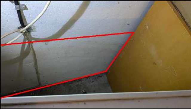
3.2 Item 14 (Picture) Garage - Staining noted at lower portion of garage wall to right of Item 13
