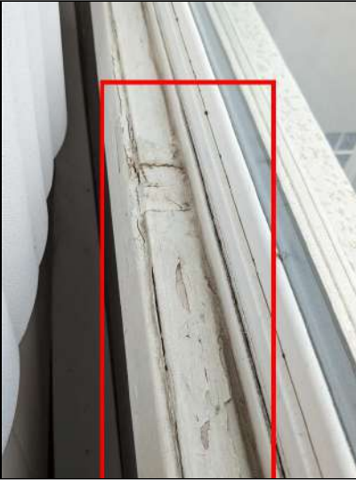
4.4 Item 5 (Picture) Living Room (2nd Floor) - Staining, possible wood damage noted, S
