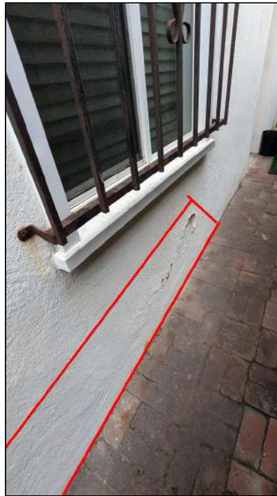
2.0 Item 4 (Picture) Peeling/wear noted at lower portion of stucco siding. No weep screed was present.
