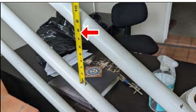
4.3 Item 3 (Picture) Space between rails is greater than 4" sphere
