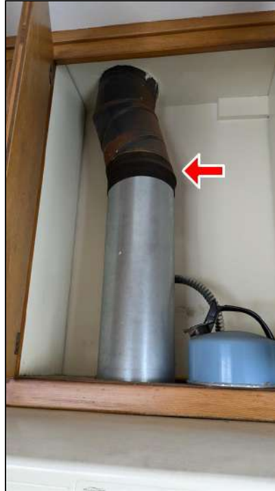
10.5 Item 2 (Picture) View of ducting above rangehood ventilator. Ducting joints should be sealed with properly-rated, UL-listed tape (typically Aluminum-backed and rated for high temperature/humidity)
