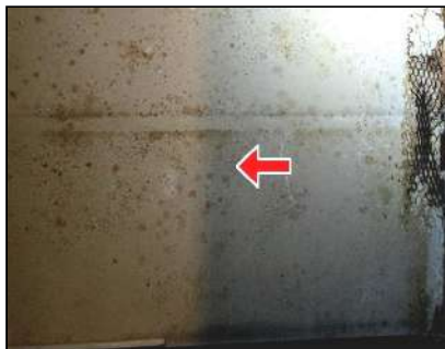
3.2 Item 20 (Picture) Close-up of discoloration, possible mold growth from Item 19
