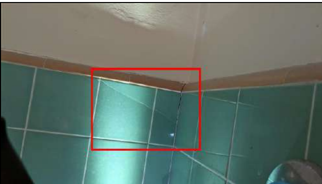
6.2.C Item 5 (Picture) Cracked tiles noted
