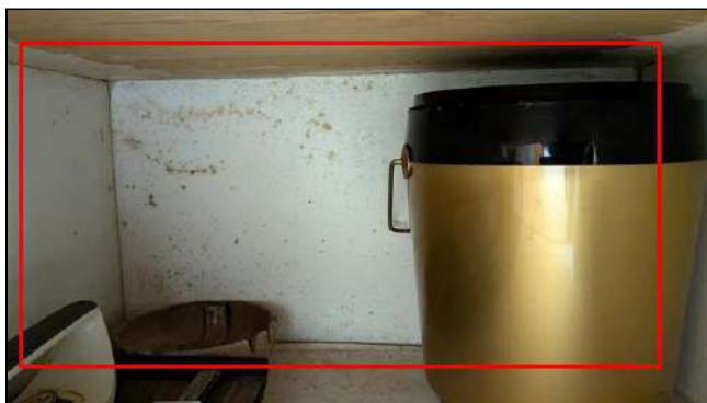
10.6 Item 3 (Picture) Discoloration, possible mold growth noted
