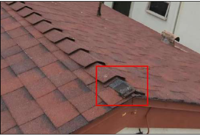
1.0 Item 3 (Picture) Missing ridge cap shingle noted. Recommend repairs.
