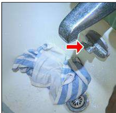
6.2.C Item 8 (Picture) Drain stopper did not work properly. Suggest repairs.
