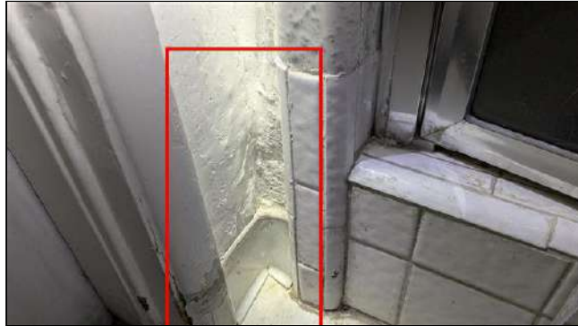
6.4.B Item 2 (Picture) Moisture damage/blistering noted at wall above Item 1
