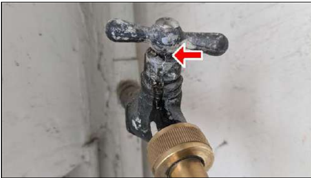
6.3.A Item 1 (Picture) Garage - Leak noted at hose bib
