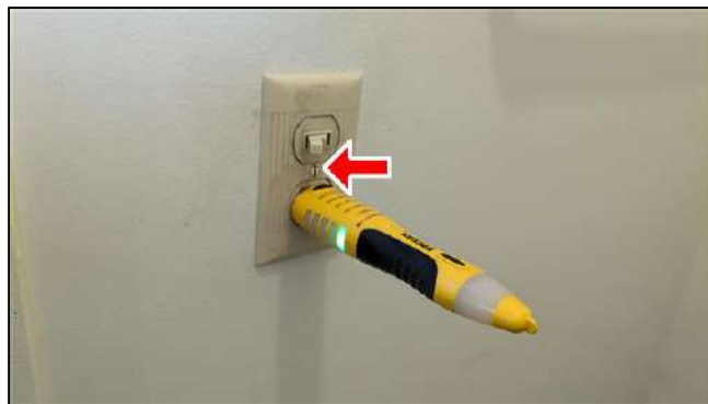
7.3 Item 2 (Picture) En Suite Bathroom - Outlets, Not GFCI
