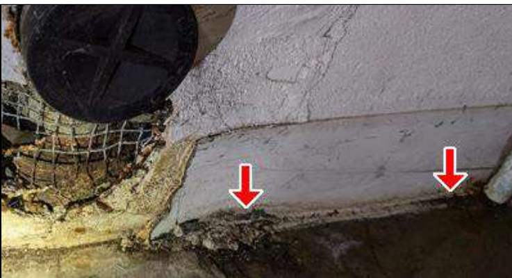
3.2 Item 12 (Picture) Close-up of area of concern - Discoloration, possible mold growth noted.
