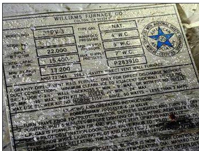
8.1 Item 2 (Picture) First Floor Bedroom - Direct Vent Heating Unit
