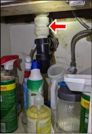
6.0.C Item 3 (Picture) Flexible drain piping noted under sink
