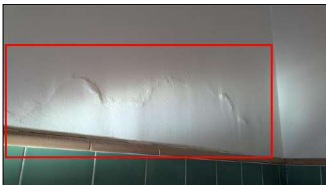
6.4.C Item 1 (Picture) Blistering noted at wall above bathtub enclosure
