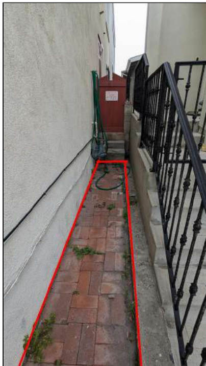
2.6 Item 2 (Picture) Area of drainage concern noted, rear. No subsurface drains were present. Evidence of ponding also noted
