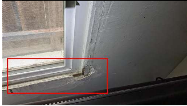
4.4 Item 2 (Picture) First Floor Bedroom - Staining/moisture damage noted at window frame.
