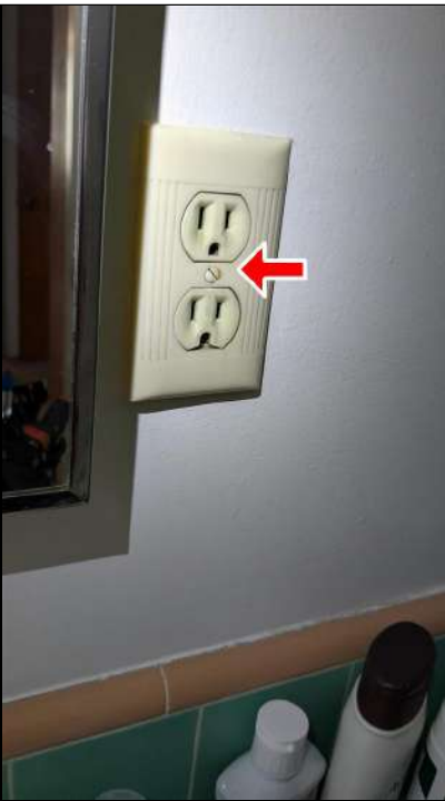
7.3 Item 7 (Picture) Shared Bathroom (2nd Floor) outlets, Not GFCI
