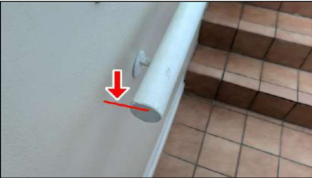
4.3 Item 1 (Picture) Per current building standards, the ends of hand railings should return to wall for safety.
