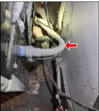
6.4.A Item 3 (Picture) Steel-braided hoses are suggested at laundry area on washing machine
