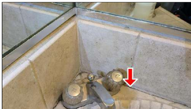
6.0.B Item 2 (Picture) MAINTENANCE TIP: Recommend caulking where countertop meets backsplash to prevent water seepage behind cabinet
