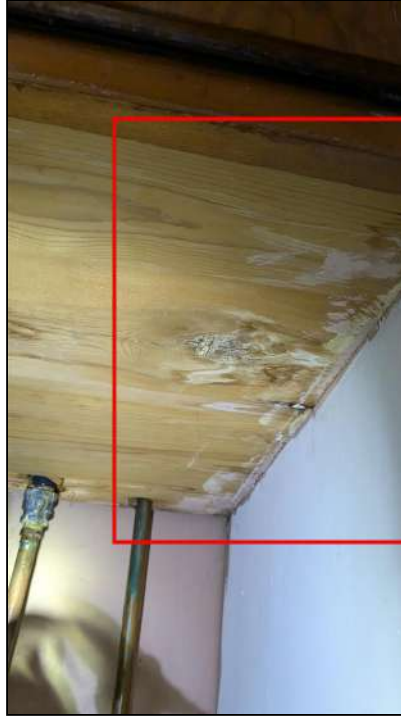
6.6.A Item 7 (Picture) Staining noted under platform
