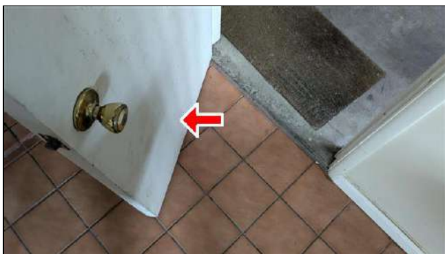
3.2 Item 1 (Picture) Door that admits to garage is not solid. Recommend repairs/replacement with a door that is fire-rated
