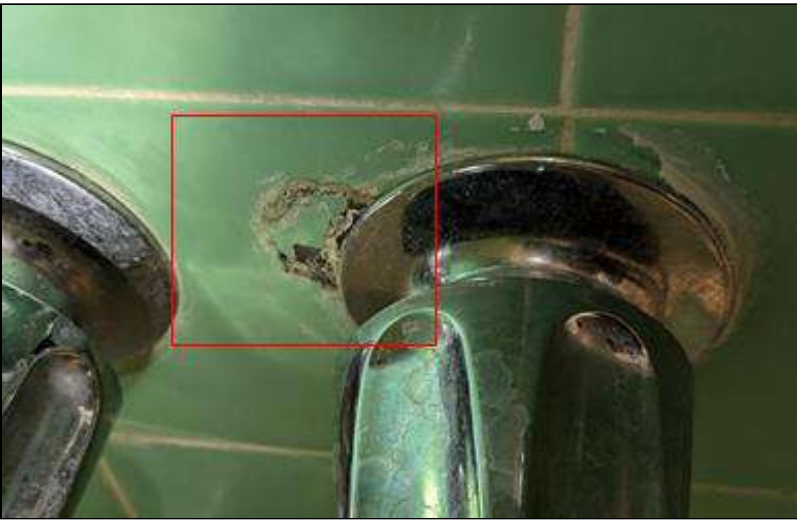
6.2.C Item 4 (Picture) Wear/damage noted at tile. Recommend grout repairs/tile replacement as needed to prevent moisture penetration
