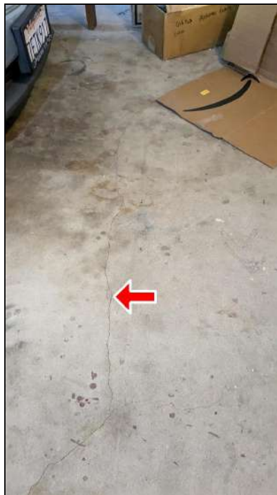
3.1 Item 2 (Picture) Cracking noted
