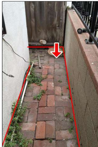
2.6 Item 3 (Picture) Area of drainage concern - Evidence of ponding noted, rear area
