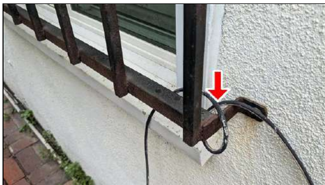
7.4 Item 1 (Picture) Loose cable noted at exterior, rear
