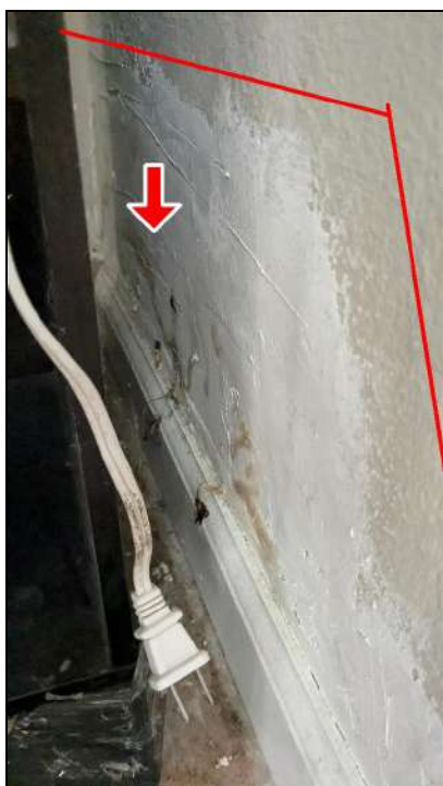
4.0 Item 9 (Picture) Foyer: Repairs noted at wall with staining observed to left of Item 7
