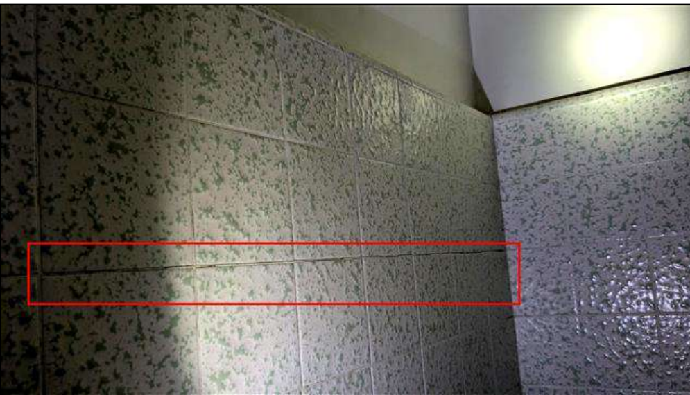
6.2.B Item 6 (Picture) Cracking noted at grout
