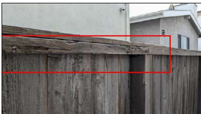
2.5 Item 6 (Picture) Wear, wood damage noted at fencing
