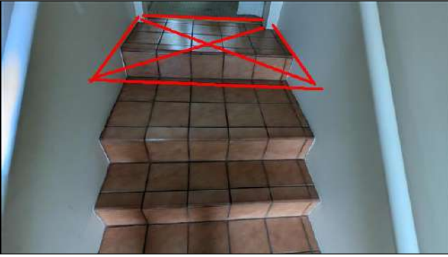
4.2 Item 3 (Picture) Unconventional installation noted. No landing was present at top of stairway
