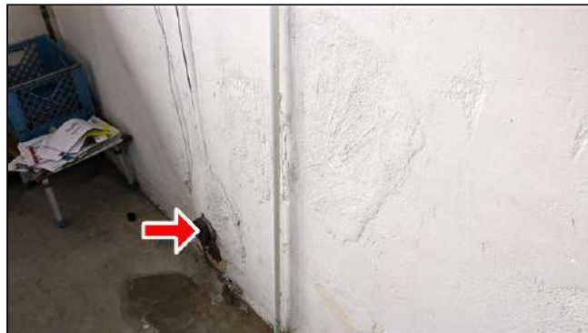
6.1.A Item 2 (Picture) Garage - Location of clean-out
