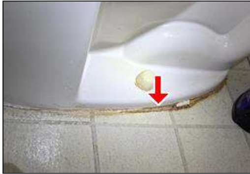
6.1.C Item 2 (Picture) Staining noted at base of toilet
