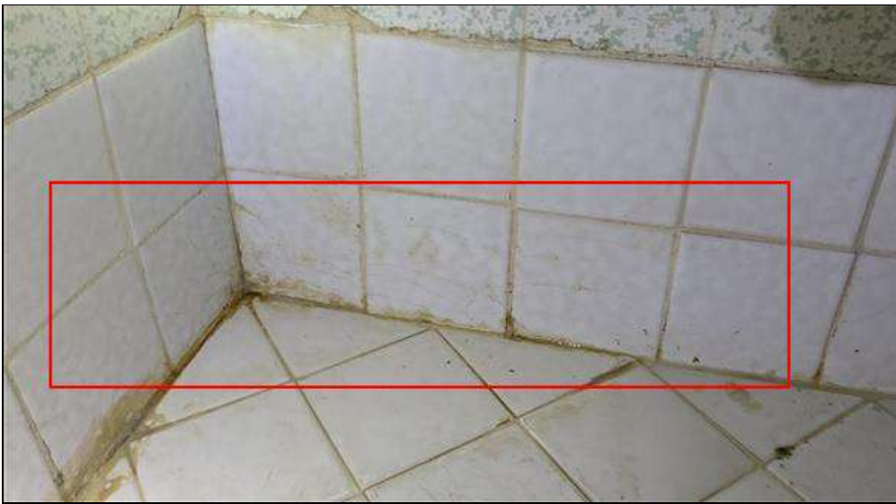
6.2.B Item 13 (Picture) Fissures/wear noted at lower tiles
