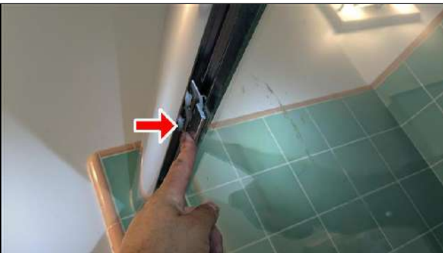
6.2.C Item 7 (Picture) Sliding glass door does not open/close easily and appears off track.
