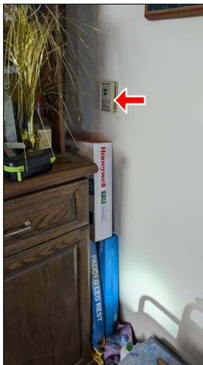
8.1 Item 7 (Picture) Thermostat for 2nd Floor Heating Unit - Wall Furnace
