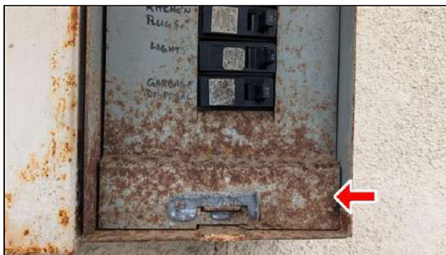
7.2 Item 3 (Picture) Rust noted at dead front (interior coverplate)
