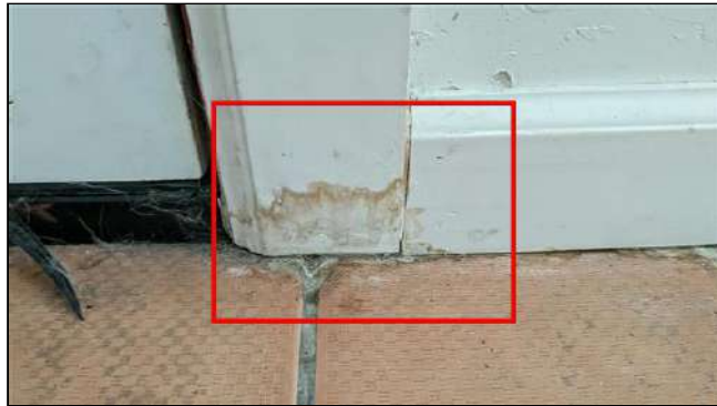
4.0 Item 6 (Picture) Foyer: Close-up of staining from Item 5
