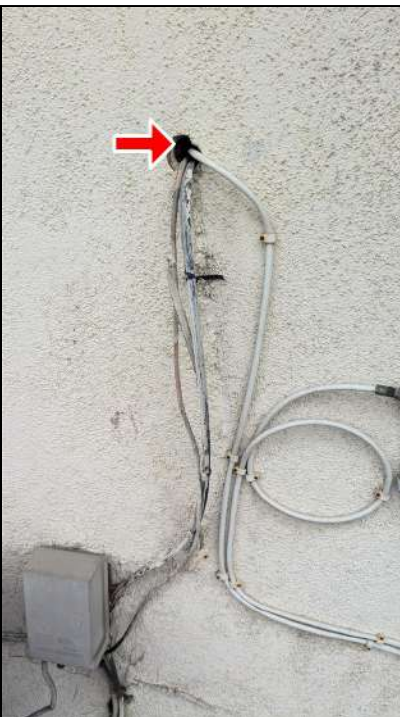
2.0 Item 5 (Picture) Gap noted at N siding. Recommend sealing/repairs to prevent moisture penetration and insect pest intrusion.
