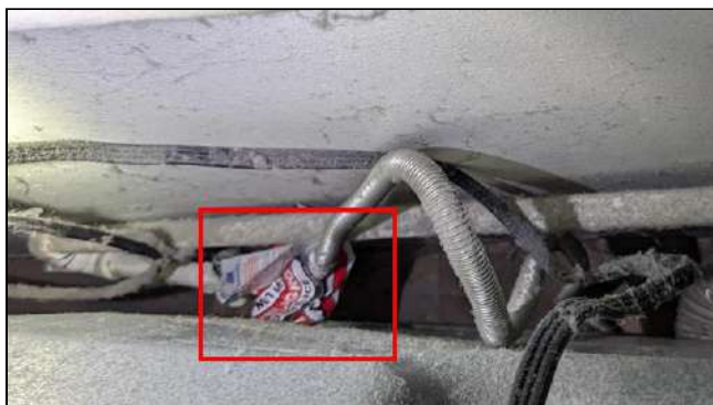
6.4.A Item 4 (Picture) Red Tag noted at gas line by dryer in Laundry Room,
