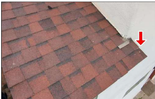
1.1 Item 1 (Picture) No kick-out flashings were present at front area
