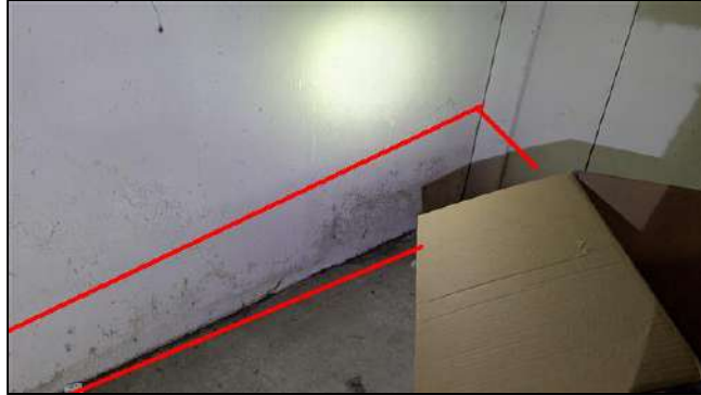
3.2 Item 16 (Picture) Area of concern at back of rear cabinet with discoloration, possible mold growth
