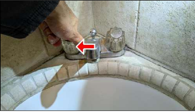
6.0.B Item 3 (Picture) Hot water handle did not work properly when tested
