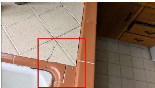
10.7 Item 1 (Picture) Cracked tiles and worn grout noted at countertop.
