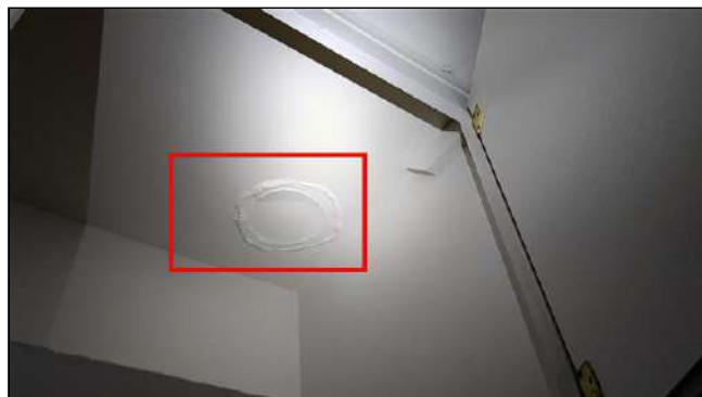
4.0 Item 14 (Picture) First Floor Bedroom - Blistering/repairs noted at closet ceiling
