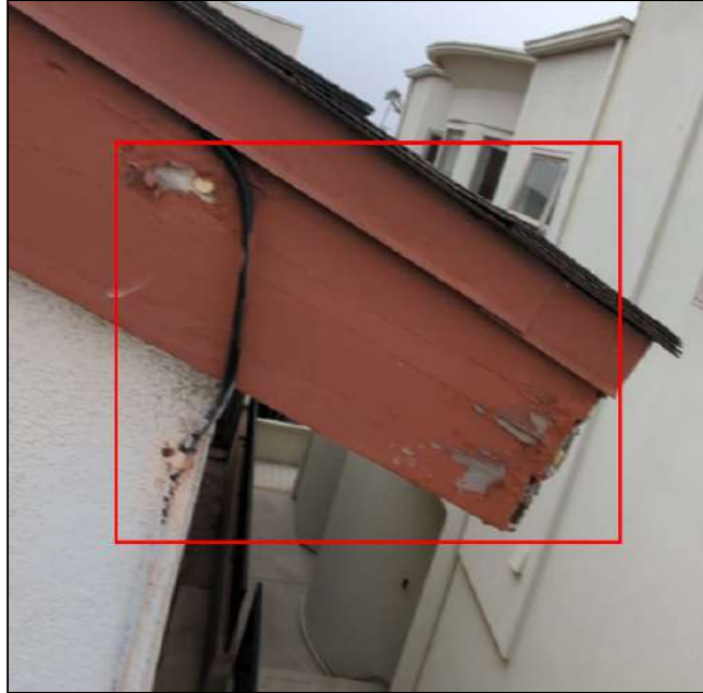
1.4 Item 2 (Picture) Peeled paint/wear noted
