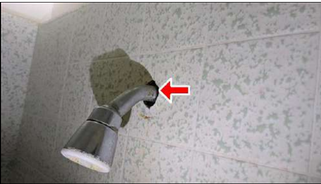
6.2.B Item 5 (Picture) No escutcheon noted. Recommend repairs.
