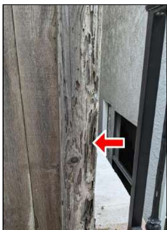
2.5 Item 4 (Picture) Wear, wood damage noted at fencing
