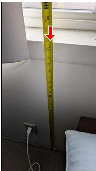
4.4 Item 13 (Picture) SE Bedroom (2nd Floor) - Openable window has sill height less than 42"
