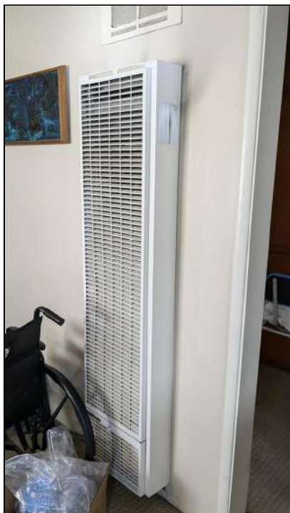
8.1 Item 4 (Picture) 2nd Floor Heating Unit - Wall Furnace
