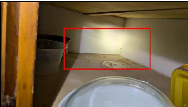
10.6 Item 12 (Picture) Discoloration, possible mold growth noted
