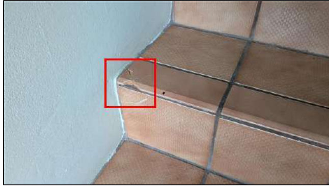
4.2 Item 4 (Picture) Cracked tiles noted at steps. Recommend grout repairs/tile replacement as needed.
