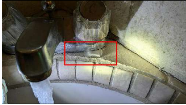
6.0.B Item 4 (Picture) Leaking noted at faucet fixture.
