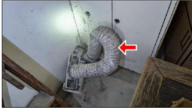
6.4.A Item 7 (Picture) Flex dryer ducting noted in garage.
