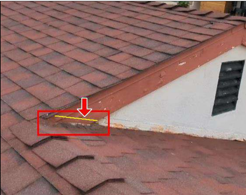
1.4 Item 3 (Picture) Fascia board should have 1" clearance from roof covering
