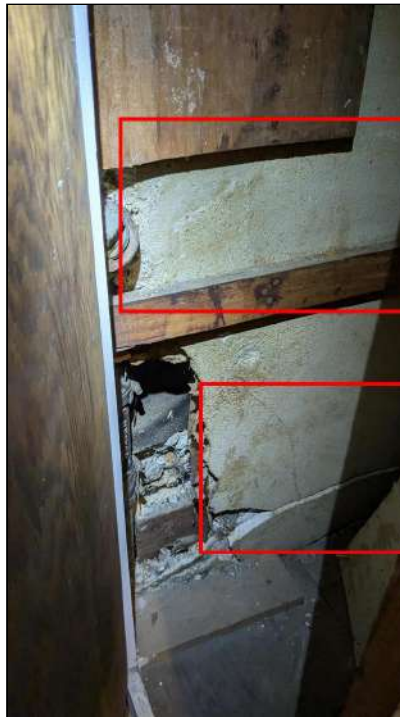
3.2 Item 18 (Picture) Staining/discoloration, possible mold growth noted at back of cabinet.
