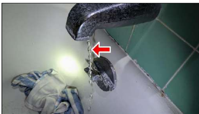
6.2.C Item 3 (Picture) Shower diverter did not work properly
