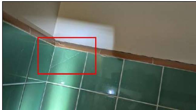
6.2.C Item 6 (Picture) Cracked tiles noted
