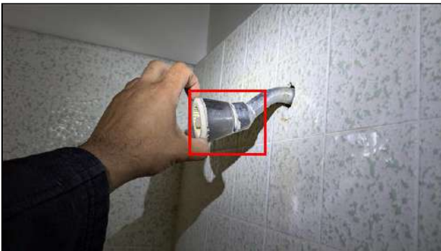
6.2.B Item 14 (Picture) Shower head detached. Recommend hardware replacement.
