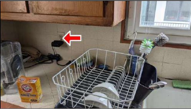
7.3 Item 5 (Picture) Kitchen countertop outlets, Not GFCI
