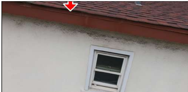
1.2 Item 1 (Picture) No rain gutters noted
