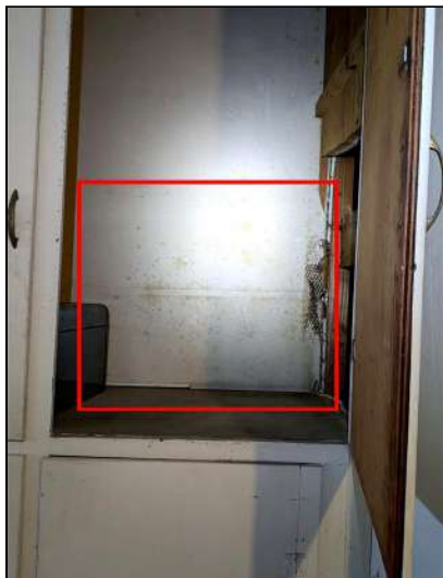
3.2 Item 19 (Picture) Garage - Discoloration, possible mold growth noted at back of cabinet
