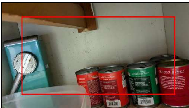
10.6 Item 5 (Picture) Discoloration, possible mold growth noted
