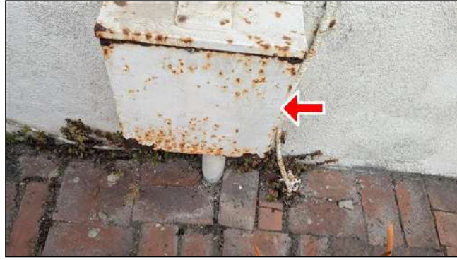
7.2 Item 8 (Picture) Wear, rust noted at enclosure near main panel. Recommend repairs/replacement with NEMA 4-rated box for lasting performance and to protect the interior components from wear
