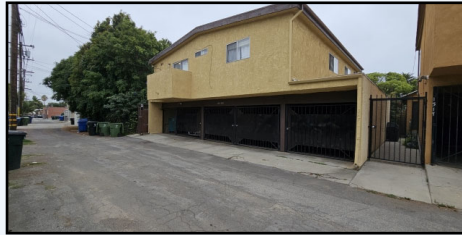
Carport access from alley
