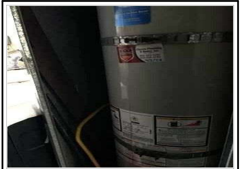
Water heater double strapped
