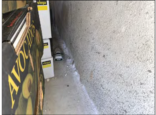
3.0 Item 6(Picture) Structural Components
