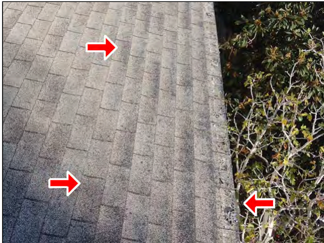
Item 1 - Item 1(Picture) Roofing
