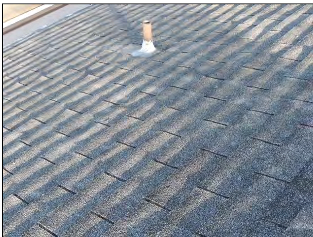
1.0 Item 7(Picture) Roofing
