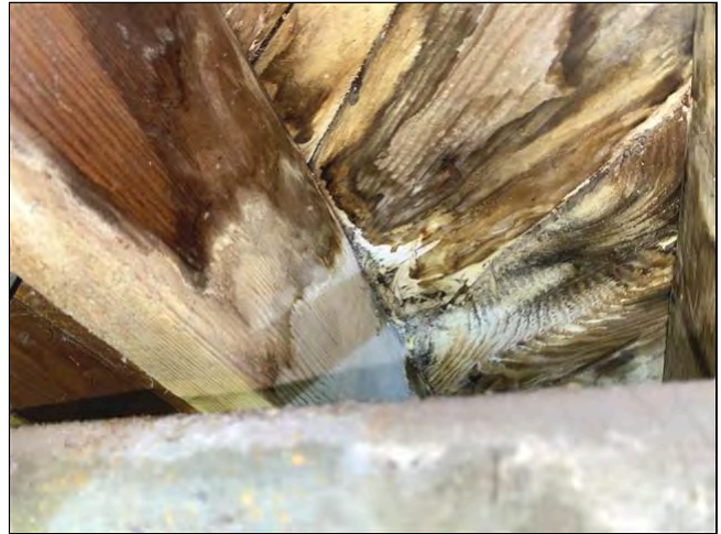
3.2 Item 2(Picture) Structural Components
