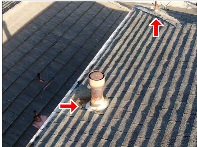
Item 3 - Item 2(Picture) Roofing
