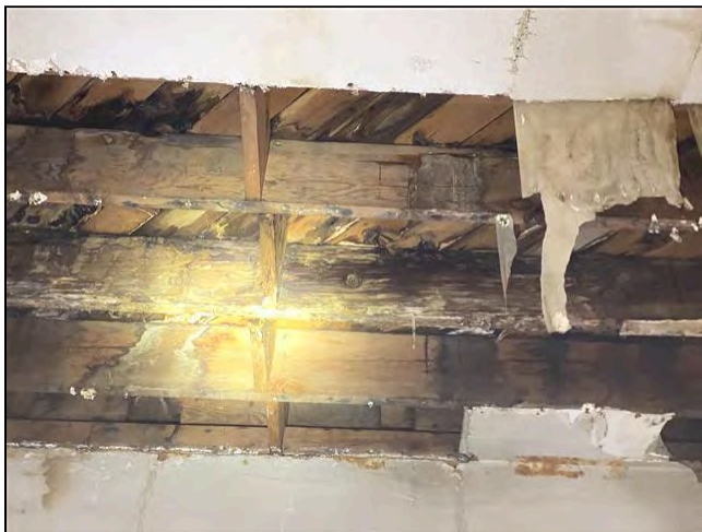
3.5 Item 5(Picture) Structural Components
