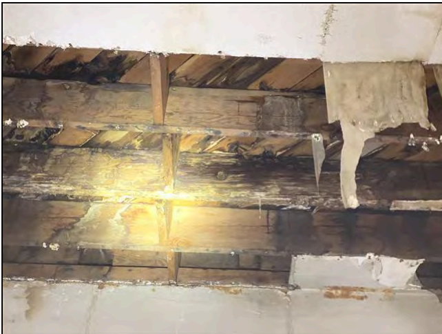
Item 18 - Item 5(Picture) Structural Components
