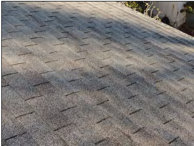
Item 1 - Item 5(Picture) Roofing
