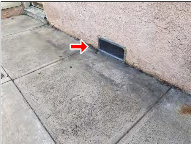
Item 13 - Item 1(Picture) Exterior Exterior Closet
