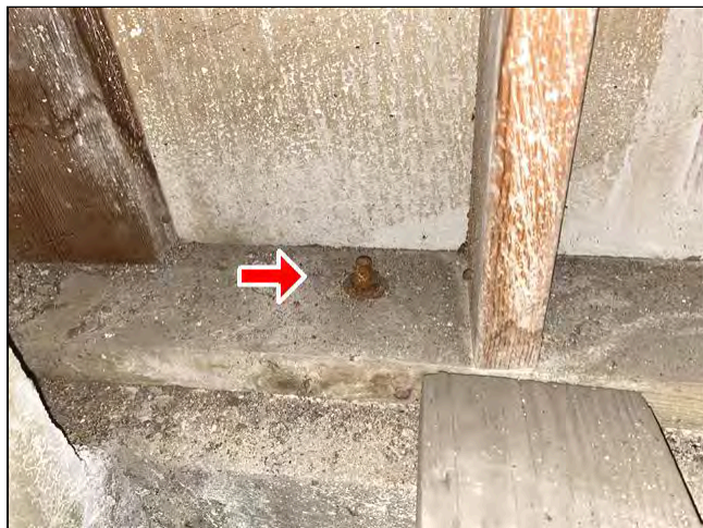
3.0 Item 8(Picture) Structural Components
