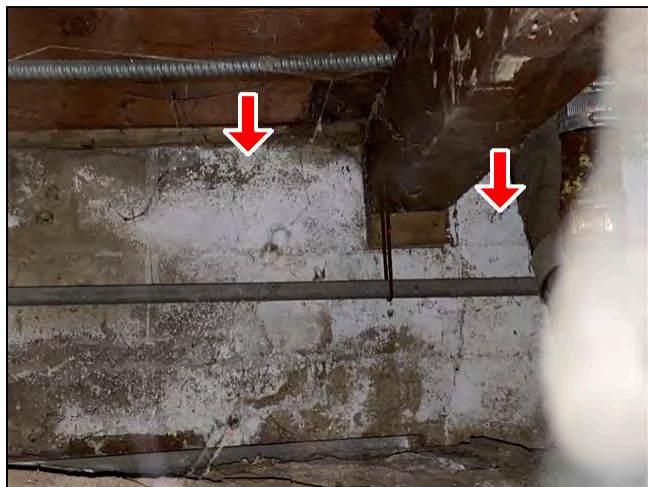
3.0 Item 4(Picture) Structural Components
