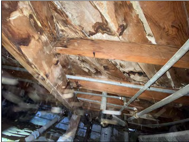
3.2 Item 1(Picture) Structural Components
