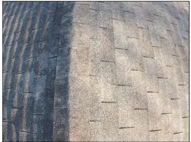
1.0 Item 4(Picture) Roofing
