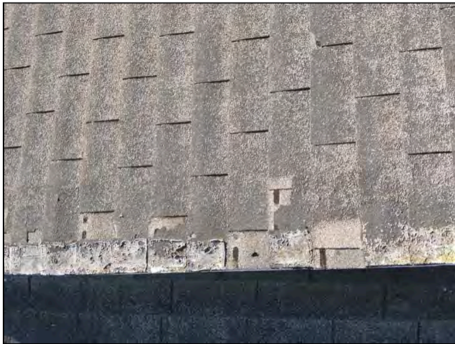
1.0 Item 3(Picture) Roofing
