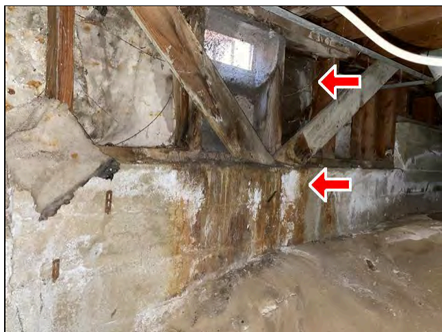
3.0 Item 9(Picture) Structural Components
