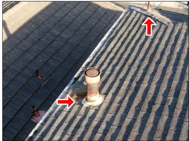
1.1 Item 2(Picture) Roofing
