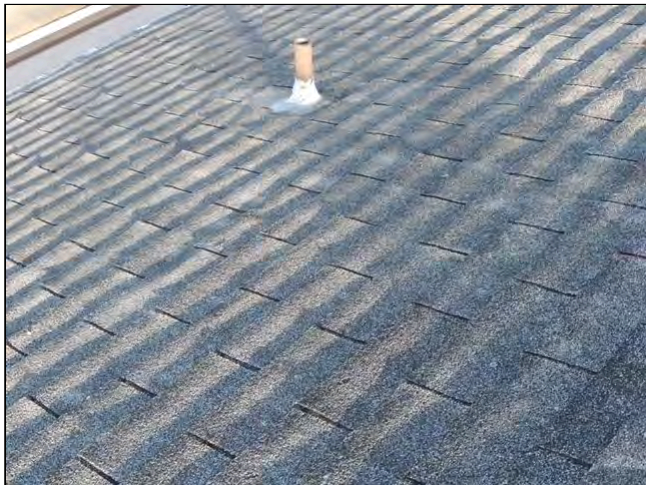
Item 1 - Item 7(Picture) Roofing
