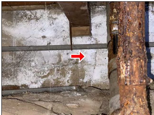
3.0 Item 3(Picture) Structural Components
