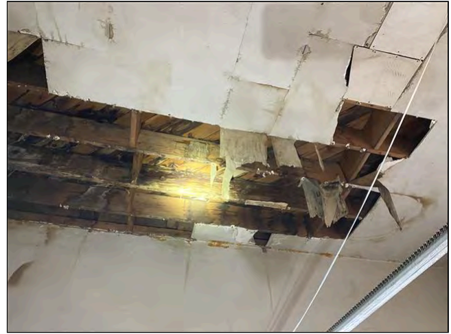
3.5 Item 2(Picture) Structural Components
