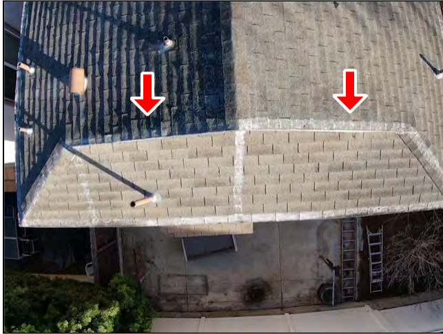
1.0 Item 8(Picture) Roofing
