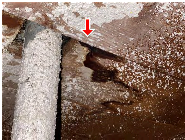
3.5 Item 8(Picture) Structural Components
