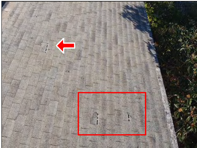
Item 1 - Item 6(Picture) Roofing
