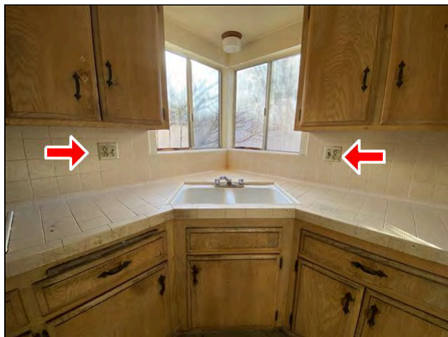
Item 36 - Item 1(Picture) Electrical System
