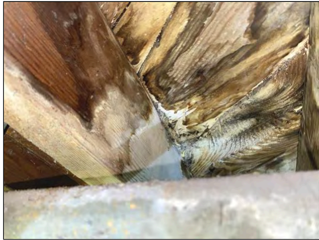
Item 16 - Item 2(Picture) Structural Components
