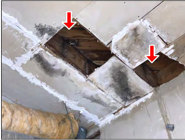
3.5 Item 1(Picture) Structural Components
