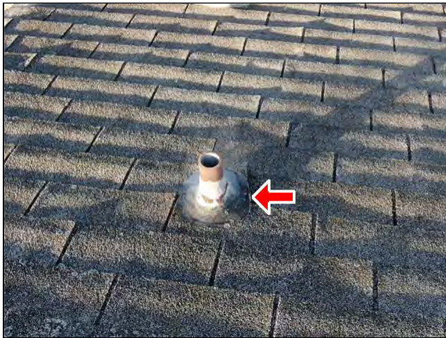
1.1 Item 1(Picture) Roofing
