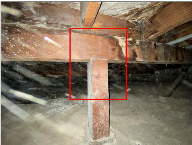
Item 17 - Item 1(Picture) Structural Components
