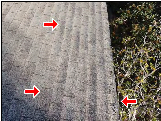
1.0 Item 1(Picture) Roofing
