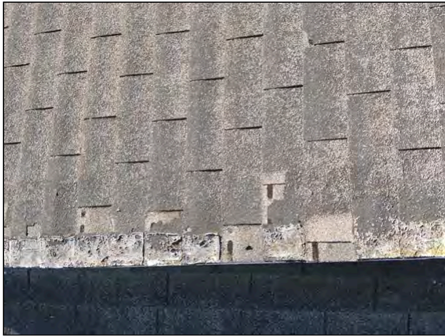
Item 1 - Item 3(Picture) Roofing
