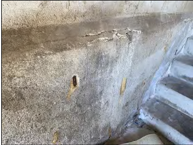
3.0 Item 5(Picture) Structural Components
