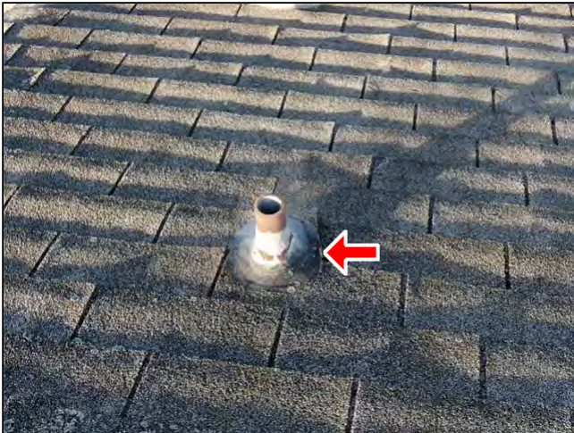
Item 3 - Item 1(Picture) Roofing
