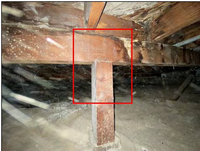
3.2 Item 3(Picture) Structural Components
