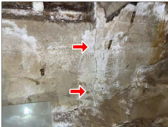
3.0 Item 2(Picture) Structural Components
