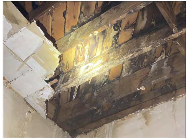
3.5 Item 4(Picture) Structural Components
