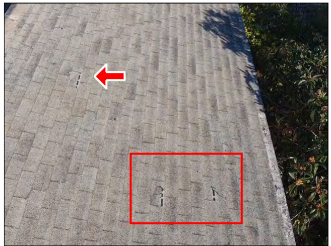
1.0 Item 6(Picture) Roofing
