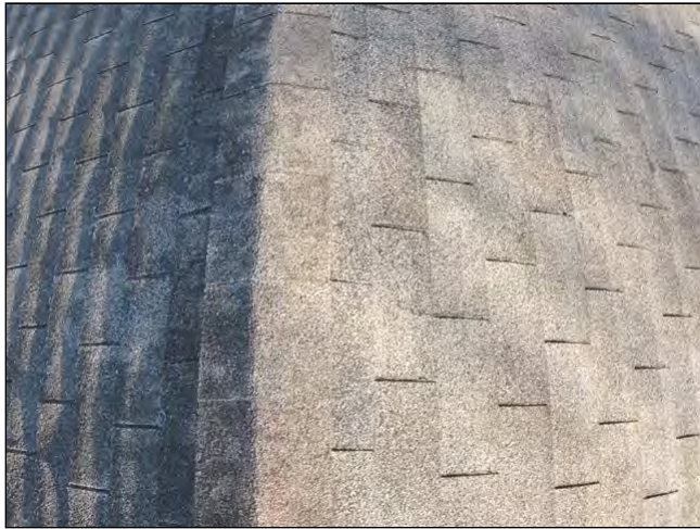
Item 1 - Item 4(Picture) Roofing
