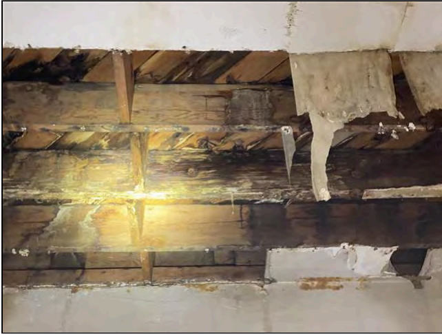
Item 18 - Item 3(Picture) Structural Components
