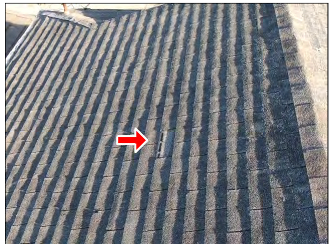
1.0 Item 2(Picture) Roofing
