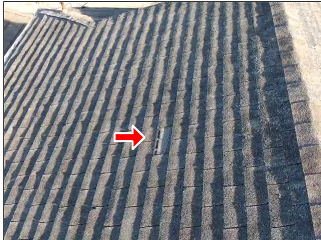
Item 1 - Item 2(Picture) Roofing
