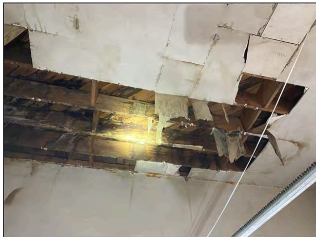
Item 18 - Item 2(Picture) Structural Components
