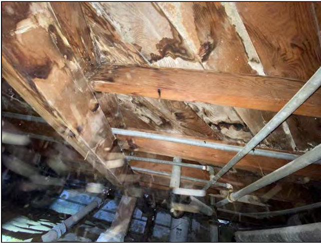
Item 16 - Item 1(Picture) Structural Components
