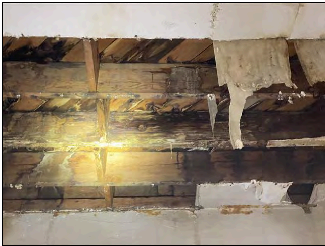
3.5 Item 3(Picture) Structural Components
