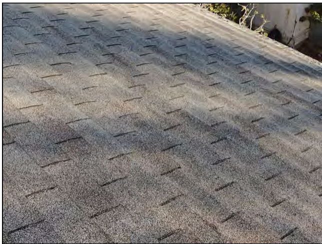
1.0 Item 5(Picture) Roofing
