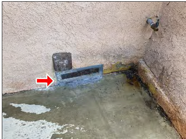
Item 13 - Item 2(Picture) Exterior
