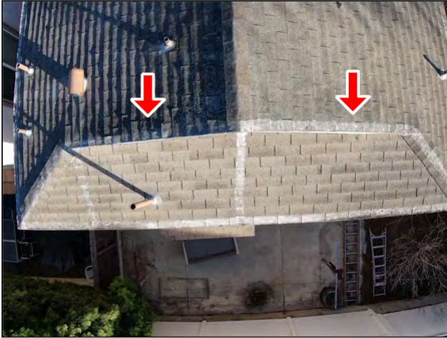
Item 2 - Item 1(Picture) Roofing
