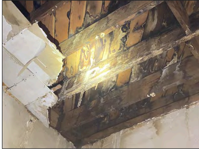
Item 18 - Item 4(Picture) Structural Components
