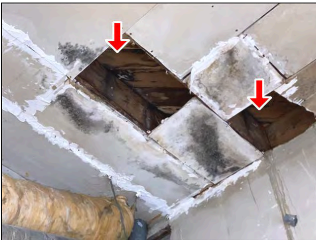
Item 18 - Item 1(Picture) Structural Components
