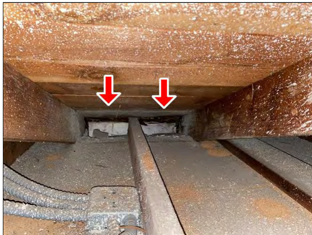
3.5 Item 7(Picture) Structural Components
