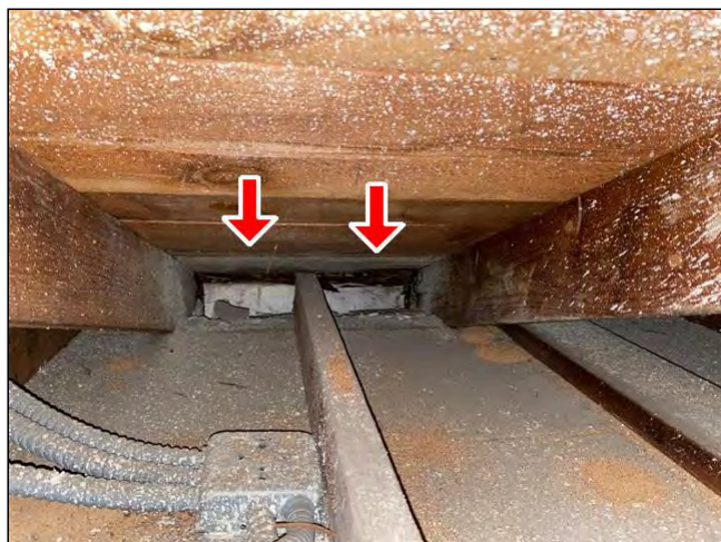
Item 19 - Item 2(Picture) Structural Components
