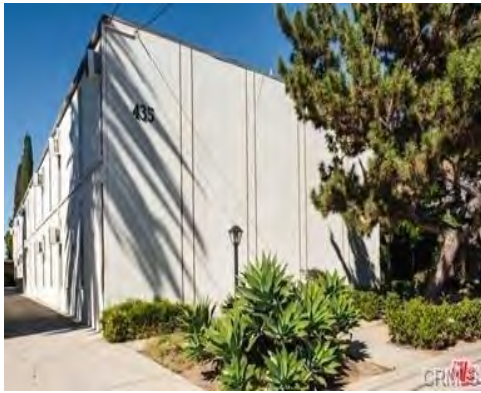
Hudson Units 435 Hudson Avenue Pasadena, CA 91101
