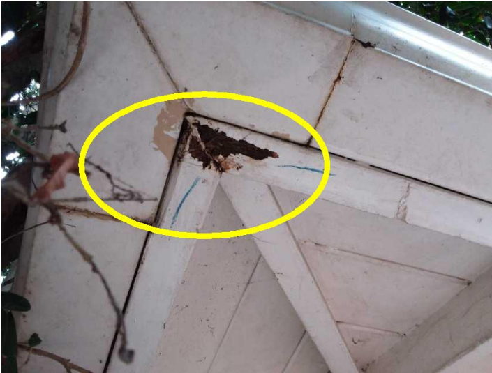
There is damage to the wood trim that should be evaluated by a termite inspector.
