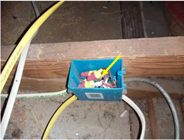
There are open electrical junction boxes, which should be sealed to contain any arcing or sparking that might occur.
