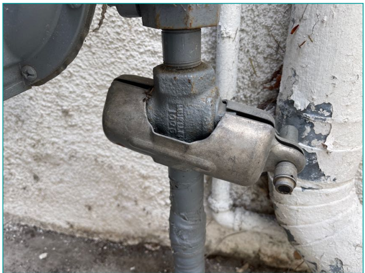
Main gas valve locked out by Gas Co.
