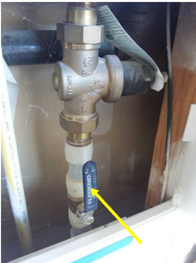
The main water shut-off valve is located inside the garage.
