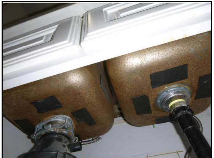
View of rust under sink.
