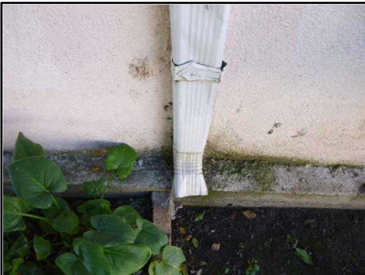
View of downspout.
