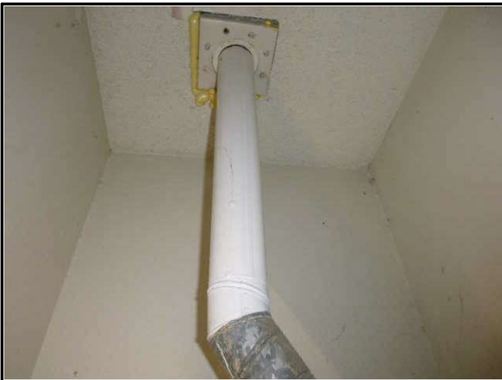
View of partly painted ventilation pipe.
