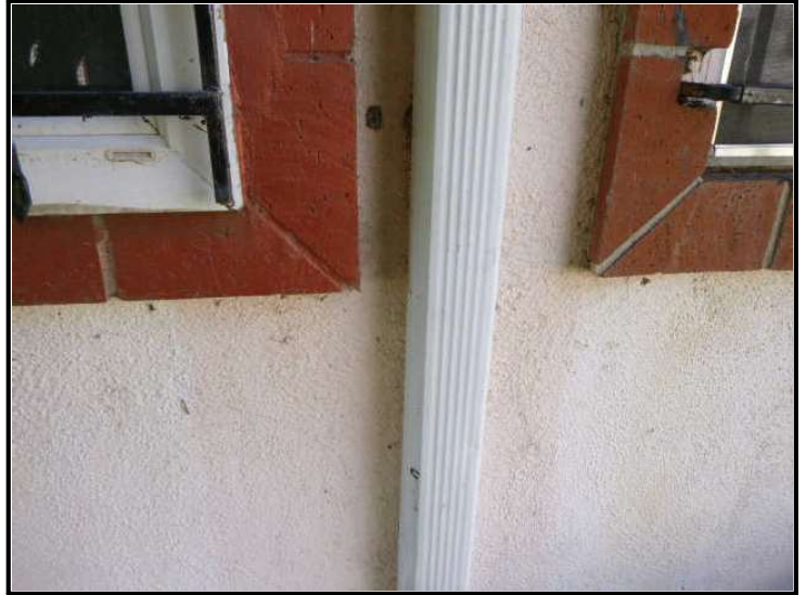
View of downspout.
