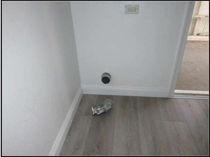
View of laundry area in living room.
