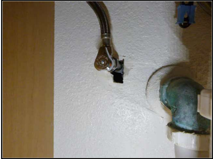
View of cutout at wall under sink in bathroom #1.
