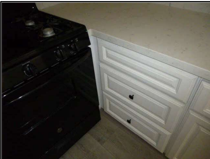
View of missing drawer handle, in contact with stove/oven, proper clearance advisable.
