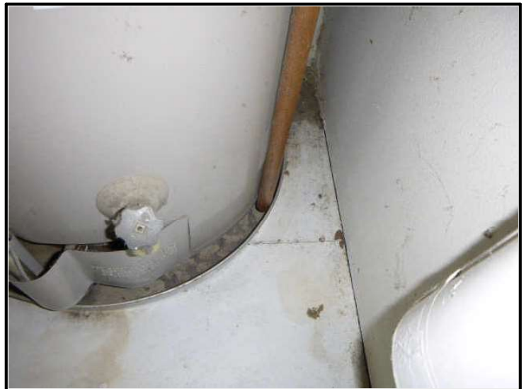
View of pan drain, unable to determine if extends to exterior.
