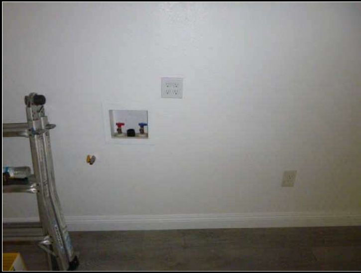
View of laundry area in living room.
