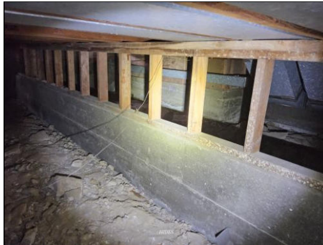
General View of the Foundation
