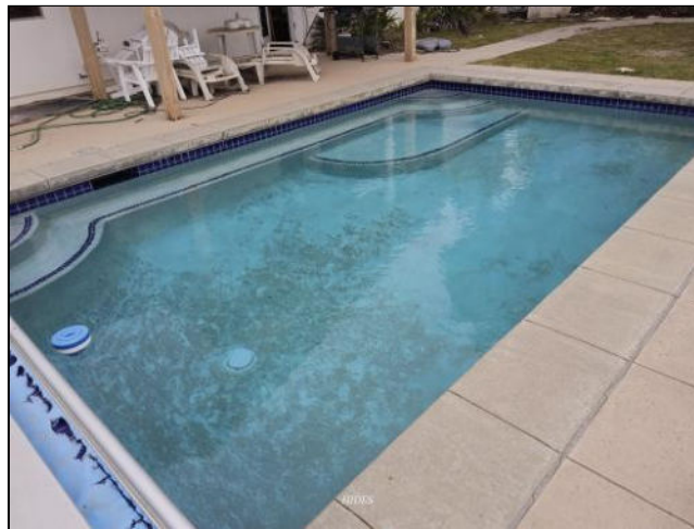
General View of the Pool and Surrounding Deck Area
