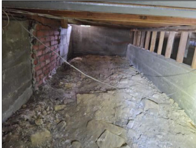
General View of the Foundation
