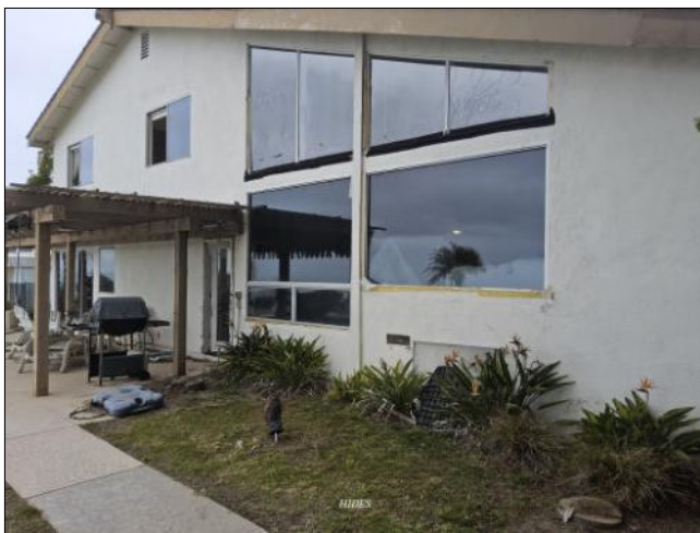
General View of the Rear Exterior of Home
