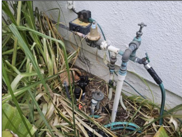
General View of the Main Water Supply Line
