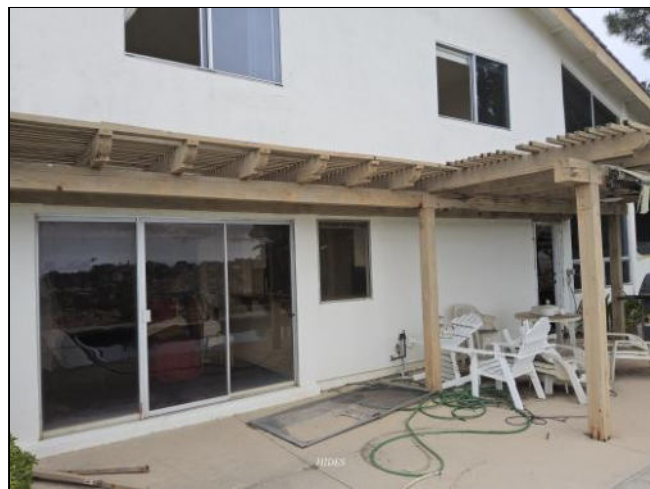
General View of the Rear Exterior of Home
