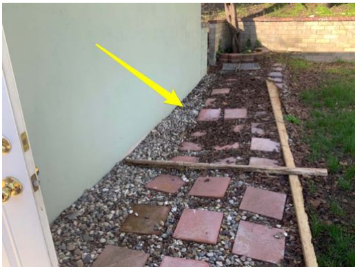
Example at the garage
