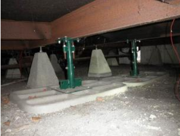
Example of the permanent foundation jacks.
