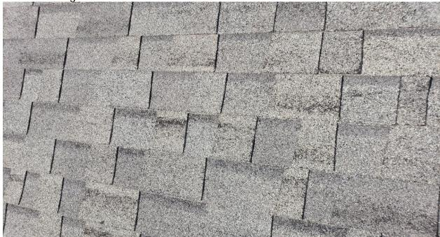
The field shingles around the solar panels also show granular loss. A lot of this can be attributed to the foot traffic from the installation of the solar panels. Some spots are worn more than others.
