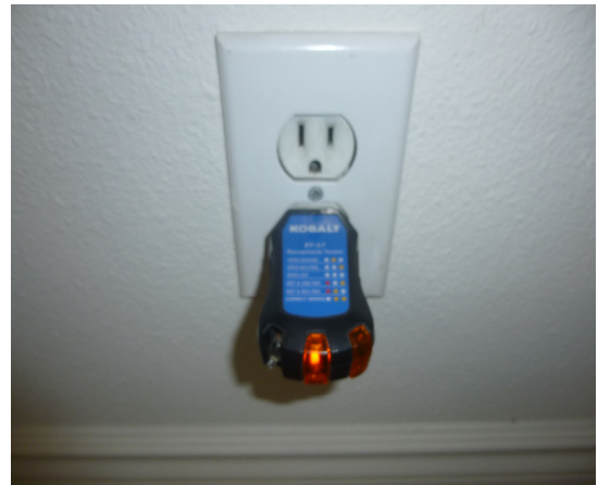
OPEN GROUND ON ALL WALL OUTLETS IN EVERY ROOM THROUGH OUT HOUSE/OUTLET ARE NOT GROUNDED BY TODAY'S STANDARDS RECOMMEND FURTHER EVALUATION
