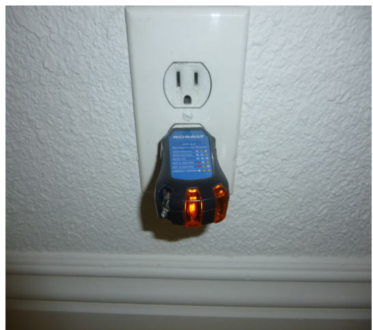
OPEN GROUND ON ALL WALL OUTLETS IN EVERY ROOM THROUGH OUT HOUSE/OUTLET ARE NOT GROUNDED BY TODAY'S STANDARDS RECOMMEND FURTHER EVALUATION
