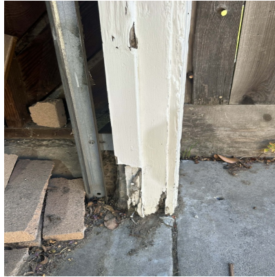
3b Fungus infection right side garage door frame
