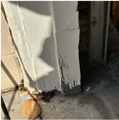
3c Fungus infection left garage door frame
