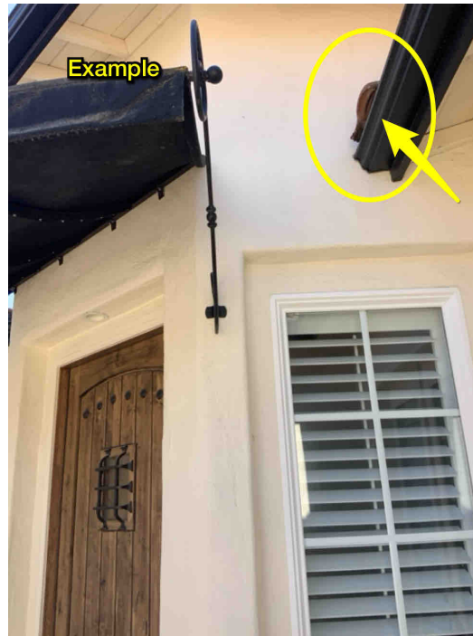
Above the front entry door area
