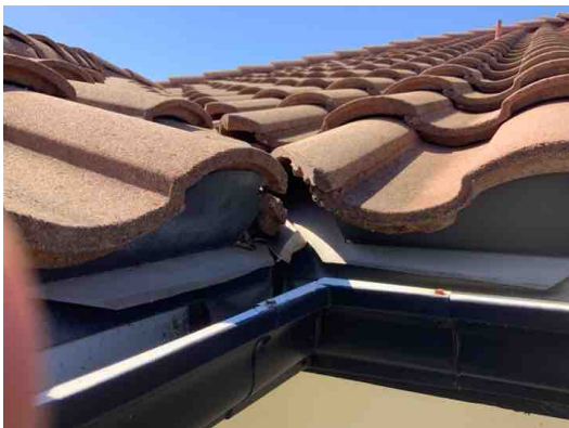
Tiles are lifted and separated
