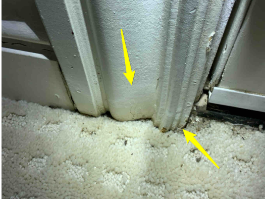
Some water damage at the door trim
