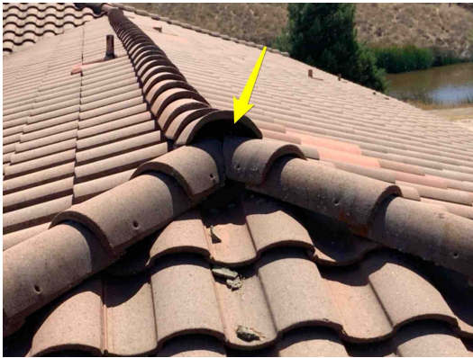
Areas should be filled with mortar
