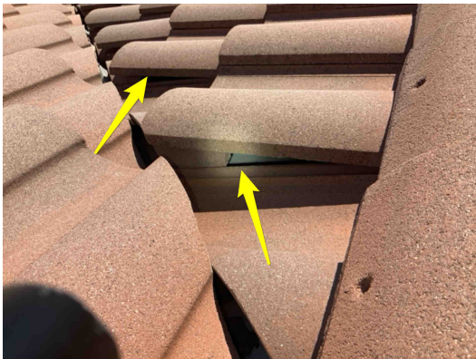
Tiles are lifted and separated
