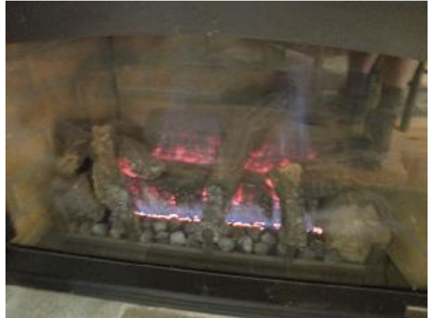
Fireplace was working during the time of inspection.
