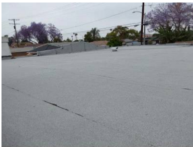
ROOF COVERING OVERVIEW
