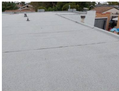
ROOF COVERING OVERVIEW
