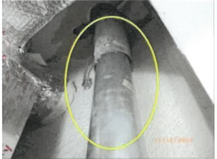
HS-7 Single wall furnace flue pipe
