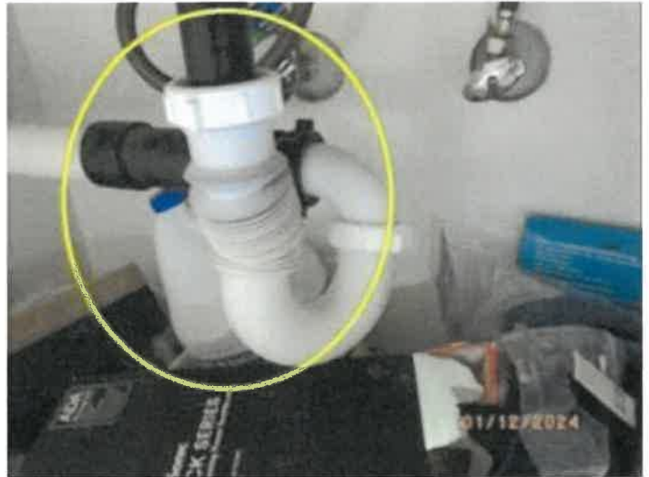
P-5 Flexible drain line at bath sink
