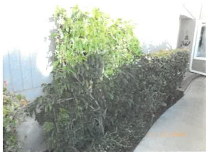
ES-1 Vegetation in contact with stucco at side of townhouse
