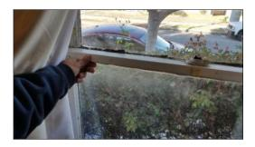
• **Description:** One or more windows that were built to open did not open or were difficult to operate at the time of inspection. Conditions may pose a safety concern if this window(s) is the only access of escape in the event of fire or other emergencies. It is recommended to have a qualified contractor repair conditions as necessary.
