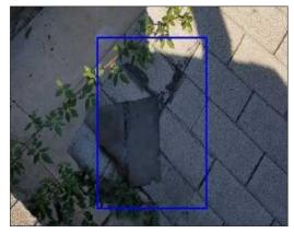
• **Description:** Composition shingles are damaged in one or more areas of the roof. Conditions will lead to further deterioration and possibly leaks if not attended. It is recommended to have a qualified roofing contractor repair affected areas as necessary
