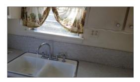
• **Description:** No ground fault circuit interrupter (GFCI) electric receptacles were found within 6? feet of sink in bathroom. Conditions pose a safety hazard due to the risk of shock. It is recommended to have a qualified electrical contractor install GFCI receptacles as needed.
