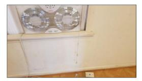
• **Description:** One or more hairline cracks were observed in one or more interior wall areas. Conditions do not appear to pose a structural concern, but the client may have a qualified contractor patch cracks as needed for aesthetic reasons.
