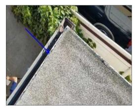
• **Description:** Roof surface gaps were found at seams in one or more areas. These may result in leaks now or in the near future. A qualified roofing contractor should evaluate and repair affected areas as needed.
