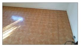
• **Description:** At the time of inspection, vinyl flooring material was missing, deteriorated or damaged in one or more areas of the interior rooms. It is recommended to have a qualified contractor evaluate conditions and make repairs to flooring as necessary.
