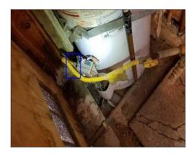
• **Description:** Not drip leg was observed on the water heater gas supply line. The purpose of drip legs is to trap oil, scale, water condensation and/or debris from the gas supply lines before they reach and damage the water heater components. It is recommended to have a qualified contractor evaluate and repair conditions as necessary.
