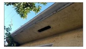
• **Description:** Soffit vents are damaged or deteriorated in one or more areas. It is recommended to have a qualified contractor evaluate and repair affected areas as necessary.
