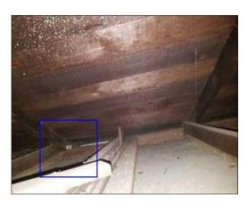
• **Description:** At the time of inspection live "knob and tube" wiring was found in the home. This type of wiring is ungrounded and it is considered unsafe by today's
