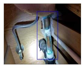
• **Comment:** Corrosion was observed on one or more facet handles, base, etc. It is recommended to have a qualified plumber evaluate conditions and repair or replace as necessary.
