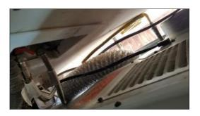
• **Comment:** Inspector found a mylar (foil) duct for dryer. Foil ducts are substandard and consider unsafe by today's standards. It is recommended to replace duct soon.
