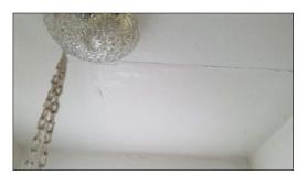
• **Description:** Minor cracks were fond on bathroom walls. Conditions do not appear to pose a structural concern, but the client may have a qualified painting contractor seal, prep and paint walls as needed.
