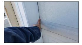
• **Description:** Garage vehicle door is missing weather strip. It is recommended to install weather strip as needed to prevent vermin and water intrusion.
