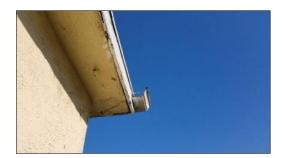
• **Description:** Gutter missing end-caps in one or more areas. It is recommended to have a qualified contractor install end-caps as needed.
