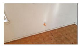
• **Description:** One or more open ground, three pronged electric receptacles were found at the time of inspection. Conditions pose a safety concern due to the risk of shock. A qualified electrical contractor should repair conditions or replace receptacles as necessary.
