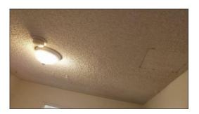
• **Description:** This property was built prior to 1979 and some ceiling area have "popcorn" textured surfaces which may have been installed prior to 1979> This material may contain asbestos, which is a known carcinogen and poses a health hazard. The client may have a qualified lab test a sample of the ceiling material and determine if it does contain asbestos.
