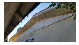
• Description: Paint is failing in one or more areas. It is recommended to have a qualified painter prep, prime, and paint wood as necessary to prevent water damage.
