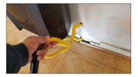
• **Comment:** The gas line for the former wall heater was out in the open and not capped recommend capping or if no longer in use removal by qualified contractor.
