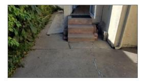
• **Description:** Sidewalk or patios slopes toward the structure, this condition will allow water to accumulate along the structure's foundation. Having a qualified contractor evaluate and correct areas to divert water away from the structure's foundation is recommended.
