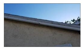
• Description: Paint is failing on one or more areas. It is recommended to have a licensed painter prep, prime, and paint wood as necessary to prevent water damage.
