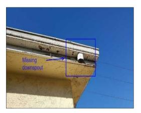
• **Description:** Termination to one or more downspouts is inadequate and may allow water to run toward the structure's foundation. It is recommended to have a qualified contractor repair or replace sections as needed.
