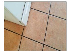
Description: Tiles appeared to be damaged and/or deteriorated at the time of inspection. It is recommended to have a qualified contractor evaluate and repair or replace tiles as necessary.
