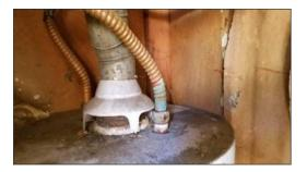
• **Description:** Corrosion was found in one or multiple areas of the plumbing lines and/or fittings. It is recommended to have a qualified contractor evaluate and repair condition as needed.
