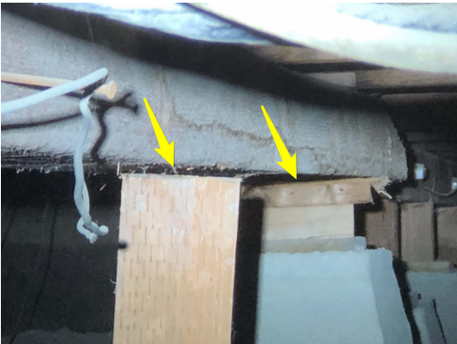
Piers are not making contact with the girder
