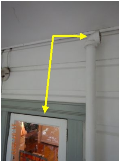
Window and open plumbing vent
