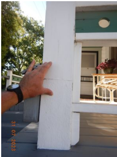
Splice in posts
