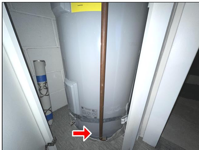
5.2 Item 1(Picture) Plumbing System
