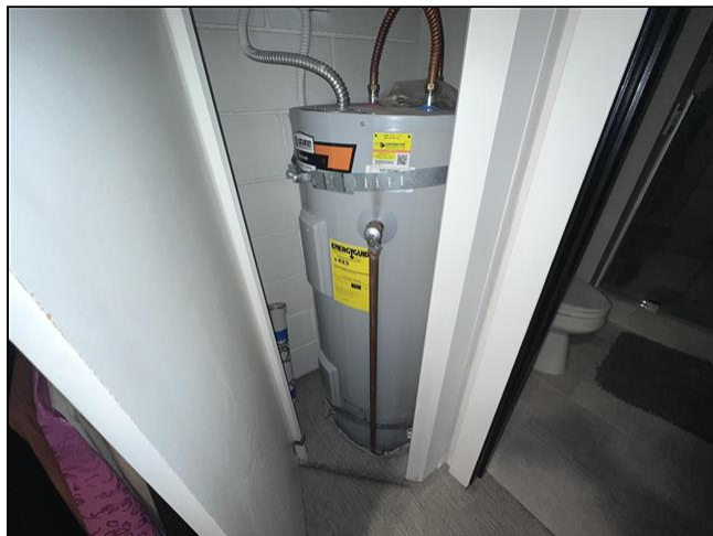
5.2 Item 2(Picture) Plumbing System
