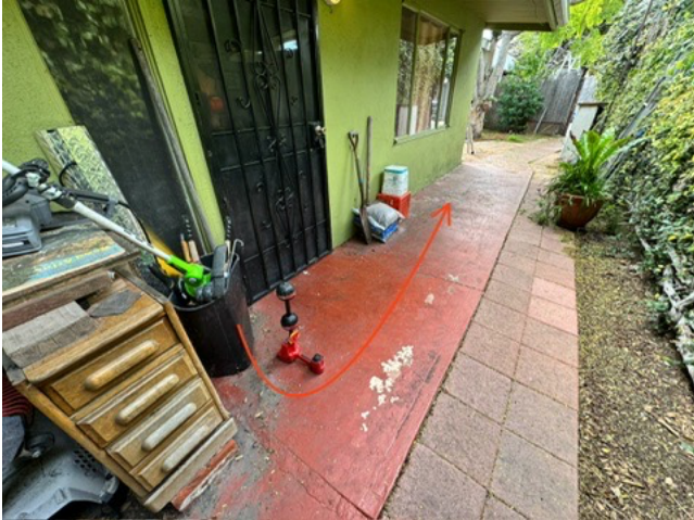
Path of sewer line. 2' deep under tool.
