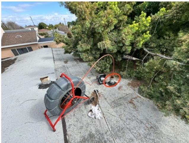
4" roof vent used for inspection.
