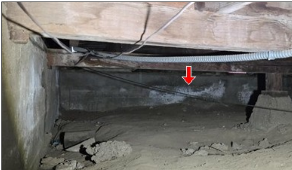
11.0 Item 1(Picture) Efflorescence, crawlspace
