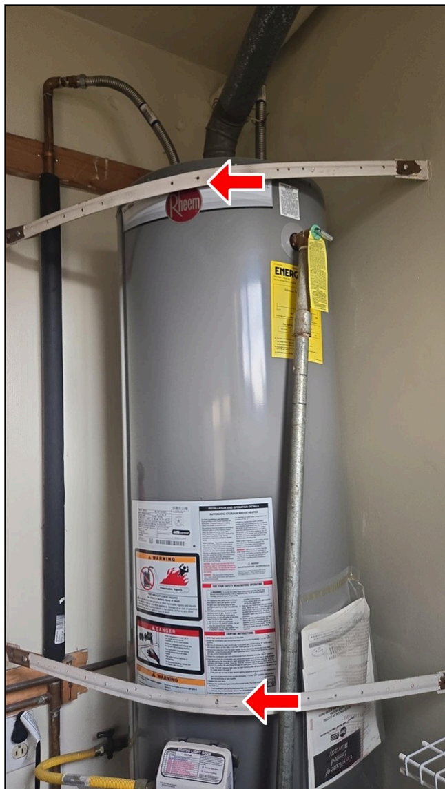
6.2 Item 4(Picture) Water heater, earthquake seismic straps
