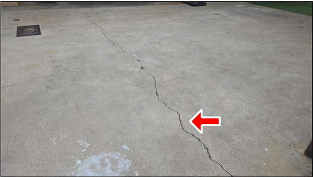
1.6 Item 2(Picture) Driveway settlement cracks
