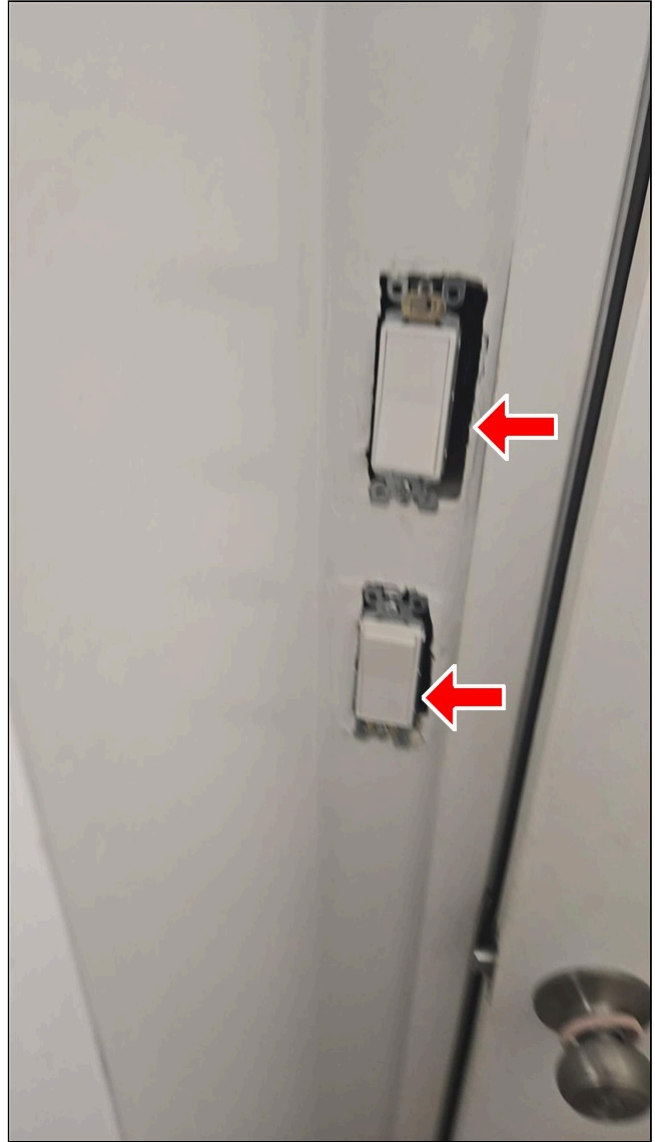
5.4 Item 2(Picture) Unit B switches, missing covers
