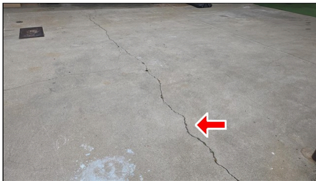
1.6 Item 2(Picture) Driveway settlement cracks
