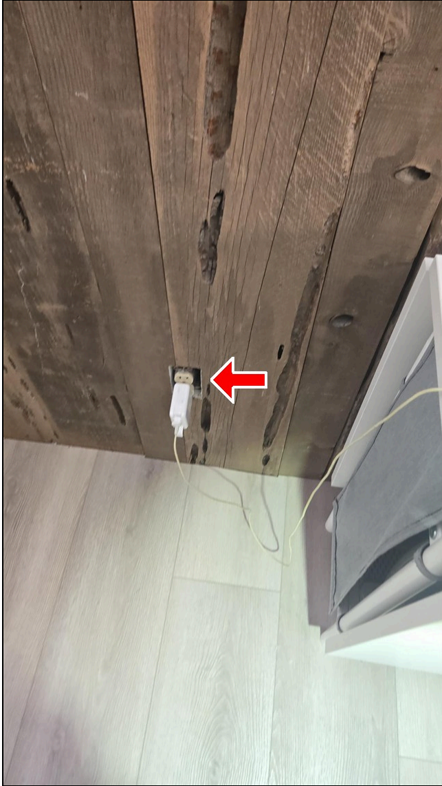
5.4 Item 1(Picture) Unit B living room outlet, missing cover
