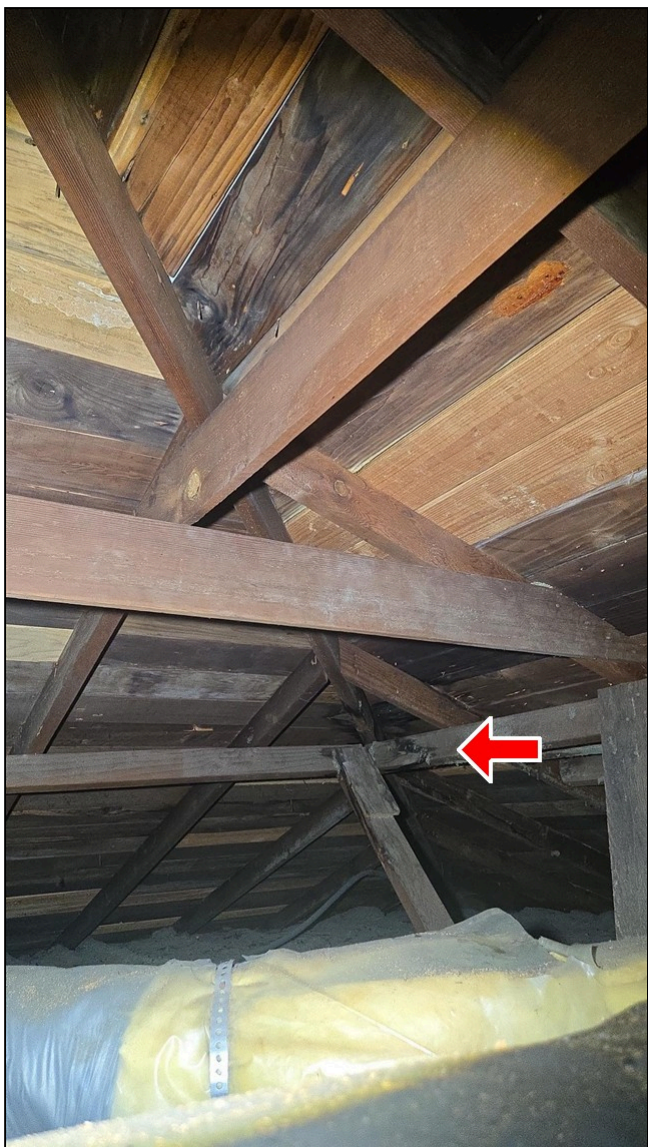
2.4 Item 2(Picture) Water stains, unit A attic
