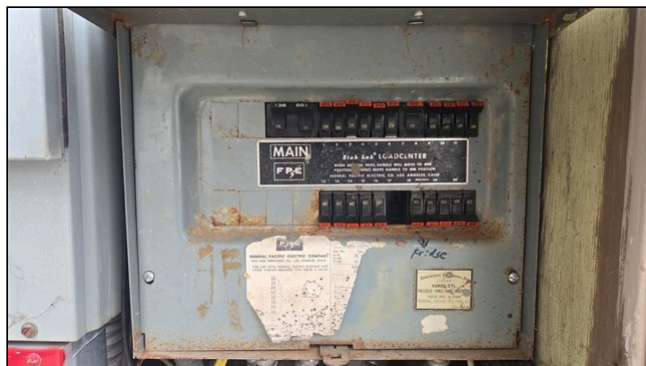
5.2 Item 1(Picture) Missing labels, unit A main distribution panel
