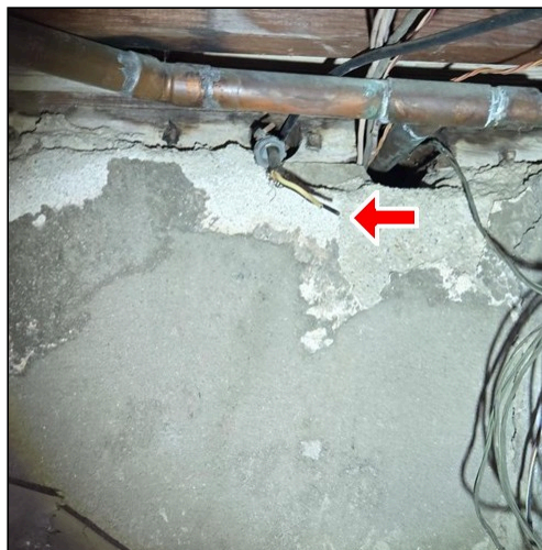
5.4 Item 3(Picture) Exposed wiring, crawlspace
