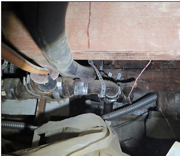
6.3 Item 3(Picture) Copper/galvanized water supply lines
