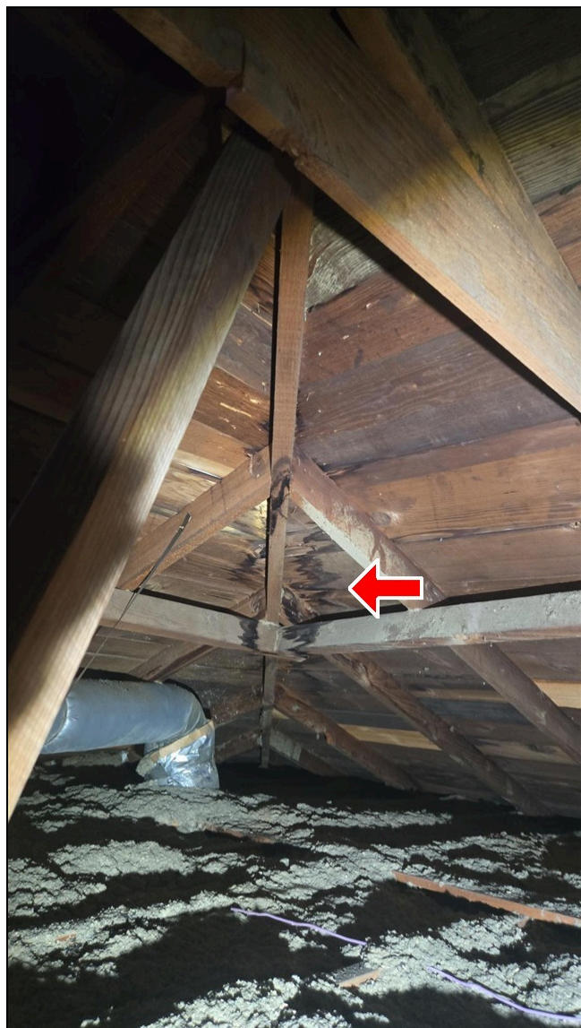
2.4 Item 1(Picture) Water stains, unit A attic
