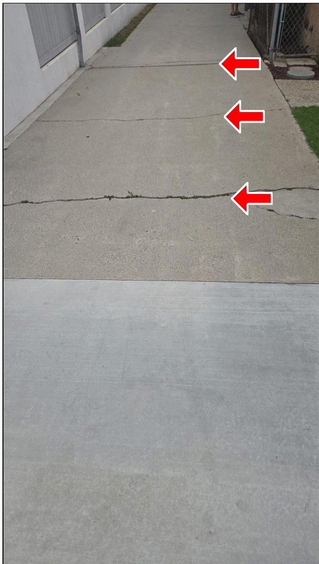
1.6 Item 1(Picture) Driveway settlement cracks
