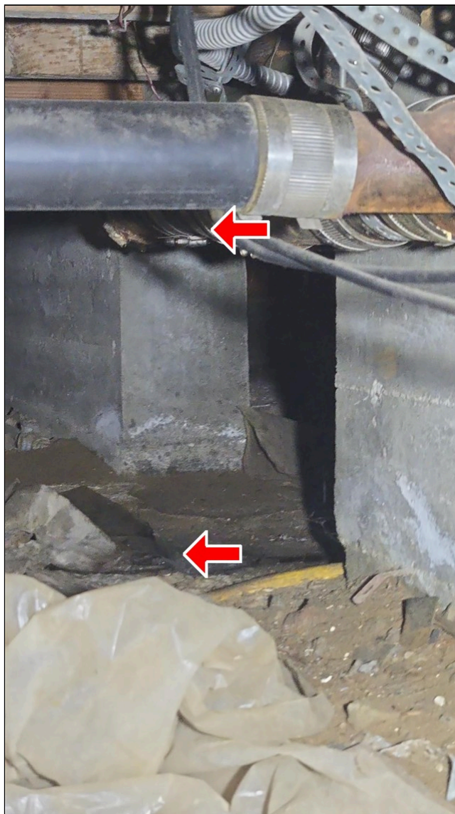
6.5 Item 3(Picture) Active leaking, crawlspace
