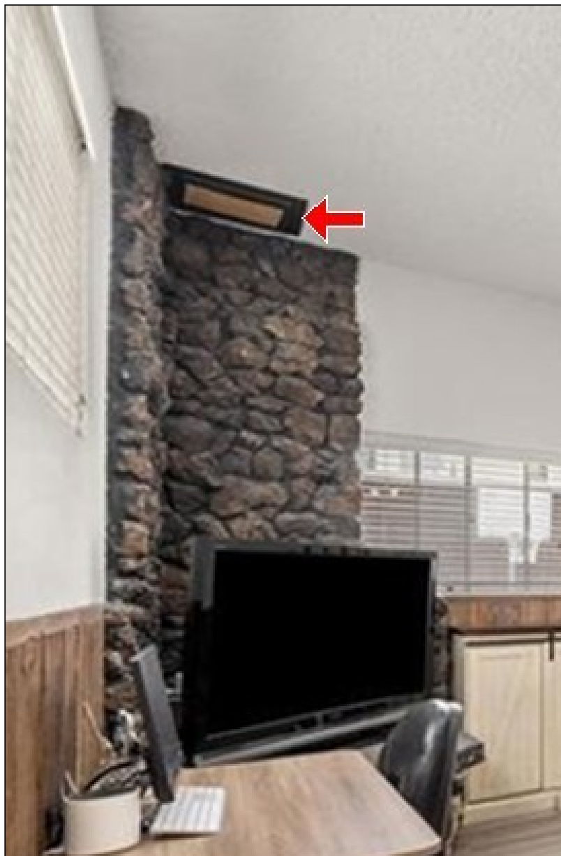
8.2 Item 1(Picture) Flue opening, unit B
