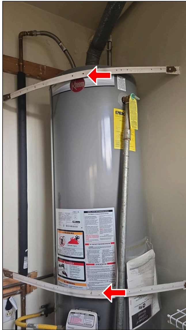
6.2 Item 4(Picture) Water heater, earthquake seismic straps
