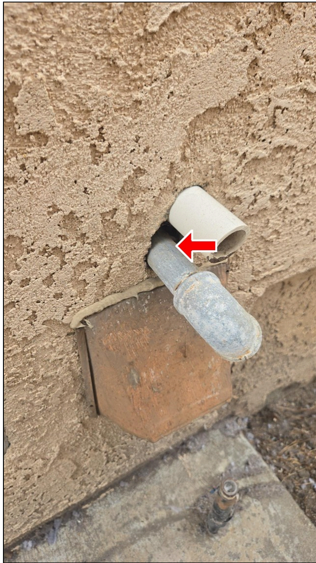
1.0 Item 2(Picture) Gaps, east exterior siding
