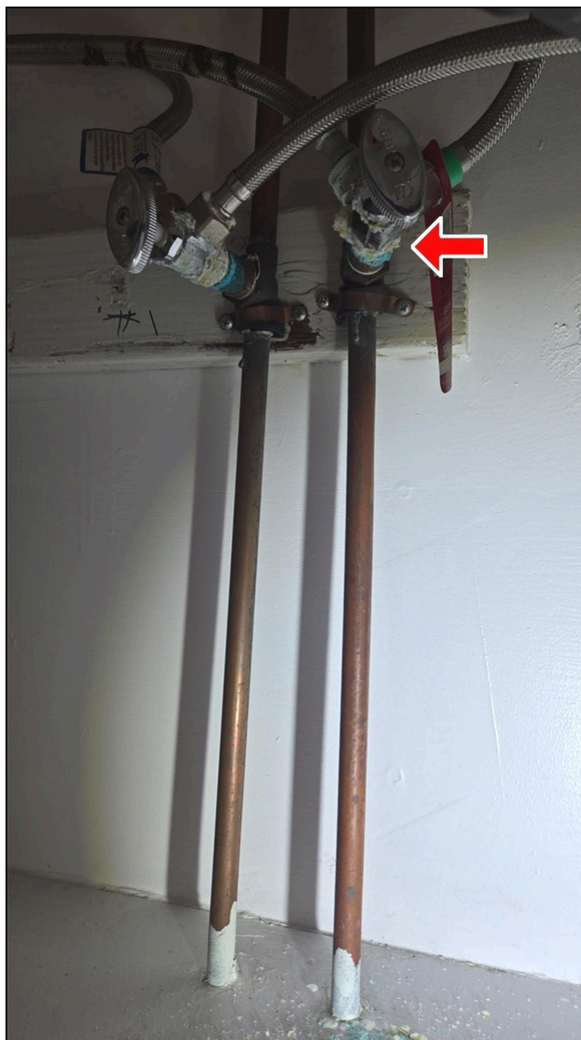
6.3 Item 1(Picture) Corrosion, unit A hall bathroom water supply shut off valves
