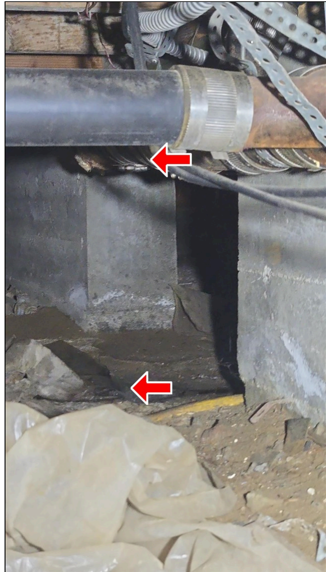
6.5 Item 3(Picture) Active leaking, crawlspace
