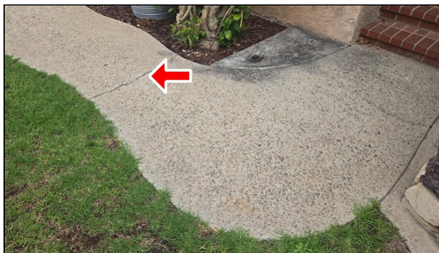
1.6 Item 3(Picture) Settlement cracks, front entry, unit A
