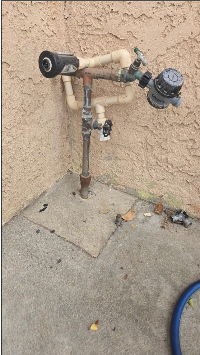
6.0 Item 3(Picture) Additional main water shut off, Unit B
