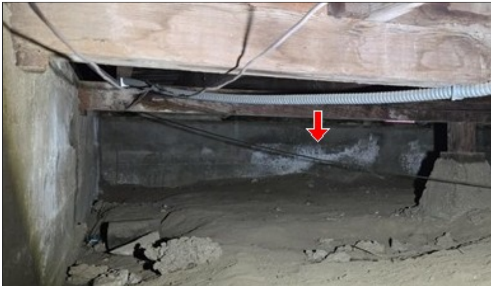
11.0 Item 1(Picture) Efflorescence, crawlspace
