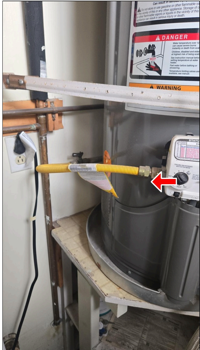
6.6 Item 2(Picture) Water heater gas line
