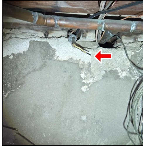
5.4 Item 3(Picture) Exposed wiring, crawlspace
