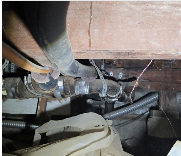
6.3 Item 3(Picture) Copper/galvanized water supply lines
