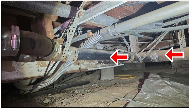
6.5 Item 2(Picture) Cast iron drain lines/ABS repairs, crawlspace
