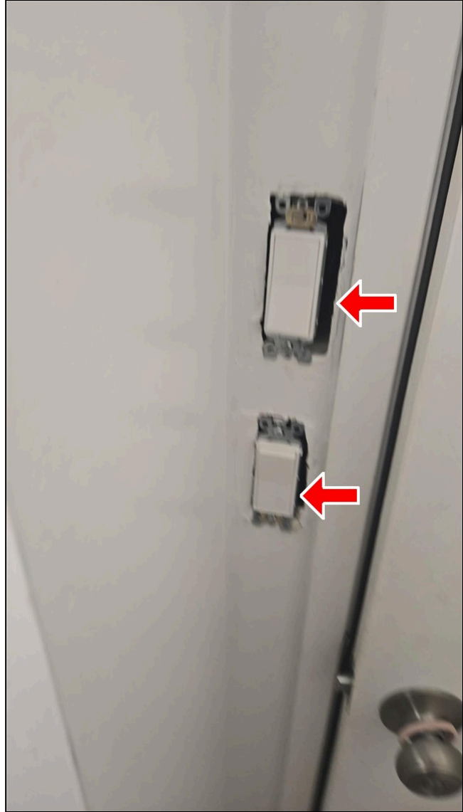
5.4 Item 2(Picture) Unit B switches, missing covers
