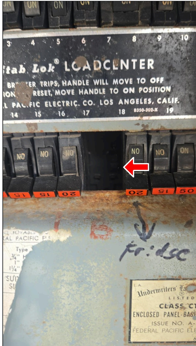
5.2 Item 2(Picture) Missing circuit breakers, unit A main distribution panel
