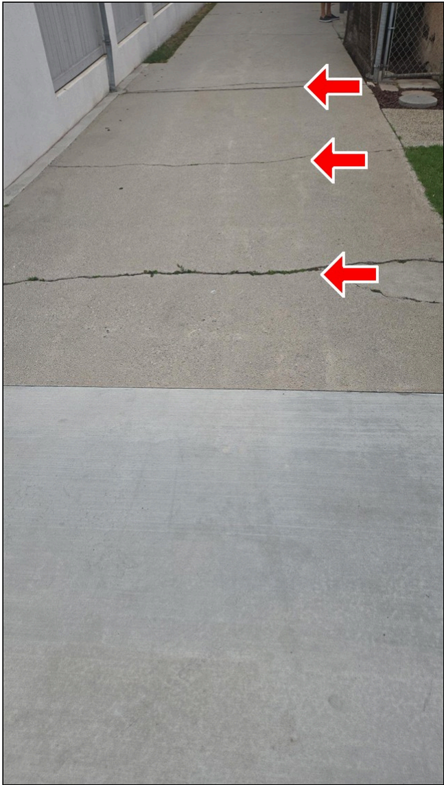
1.6 Item 1(Picture) Driveway settlement cracks
