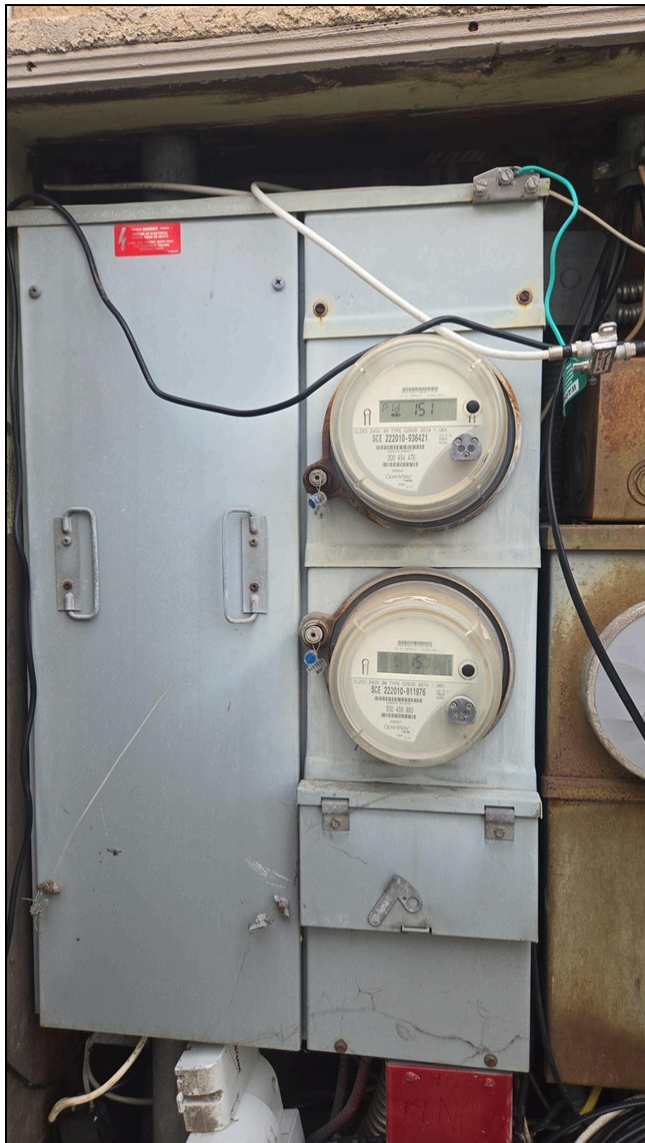
5.1 Item 1(Picture) Electric meter and main shut off (unit A and unit B)
