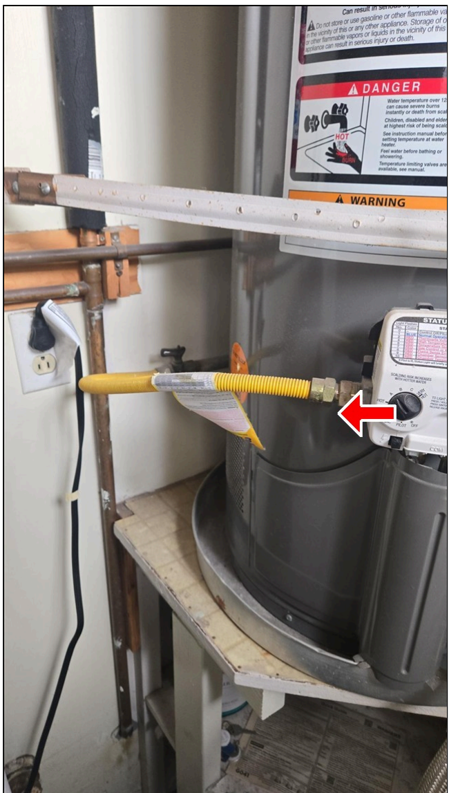
6.6 Item 2(Picture) Water heater gas line
