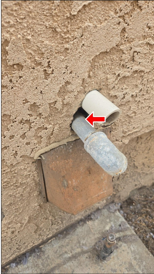
1.0 Item 2(Picture) Gaps, east exterior siding
