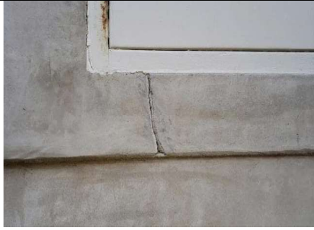
Surface Cracks
