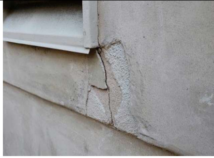
Surface Cracks
