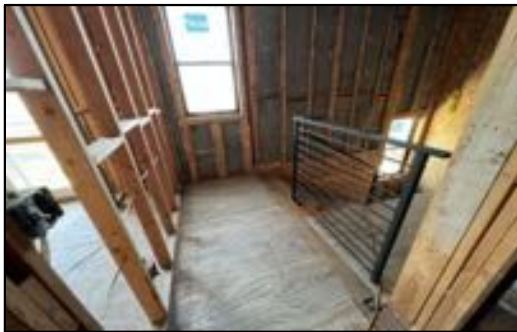
3rd Floor Landing
