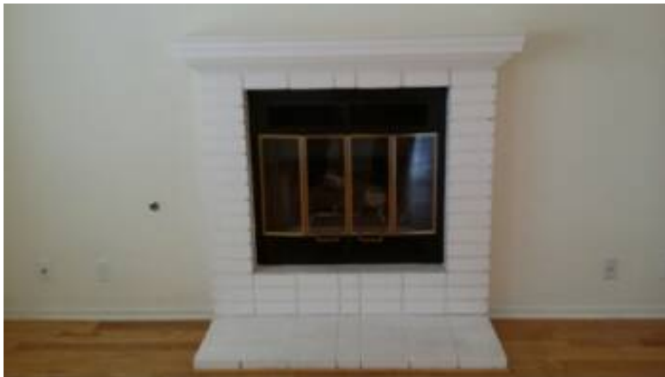
The fireplace is in acceptable condition.
