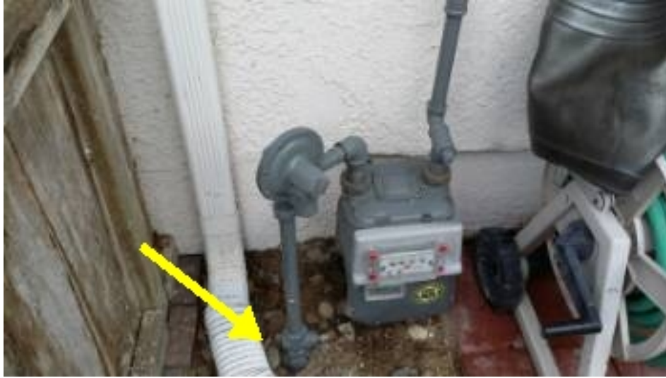
The gas main shut-off is located on right side of the home, unit or building.
