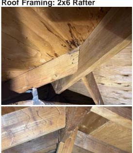
4. Sheathing: OSB - Stains were visible on the roof structure in one or more areas. These areas were dry at the time of the inspection. A past leak may have caused the stains. Recommend asking the property owner(s) about past leaks. The client(s) should monitor these areas in the future, especially after heavy rains, to determine if active leaks exist. If leaks are found, a qualified roofing contractor should evaluate and repair.
