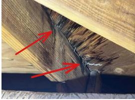
9. Main Attic Bathroom Fan Venting: Electric fan - Bathroom improperly vents into attic and may cause moisture damage to the insulation. The services of a qualified contractor is recommended to evaluate and estimate repairs.
