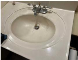
11. Taucets/Traps: Delta fixtures with a PVC trap - Rusty faulty drain stopper. A licensed plumber is recommended to evaluate and estimate repairs.
