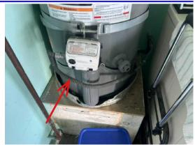
11. Garage Water Heater Flue Pipe: Double wall - Metal vents that are too close to wood or combustionable materials may cause the wood to burst into flames. Single wall vents should have a minimum of 6 inches of clearance and double wall, sometimes called a vent, should have 1 inch minimum clearance. A qualified air conditioning contractor is recommended to evaluate and estimate repairs.
