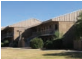
Davis AFB pinhole leaks copper
