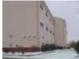
Fort Knox potable water corrosion prevention
