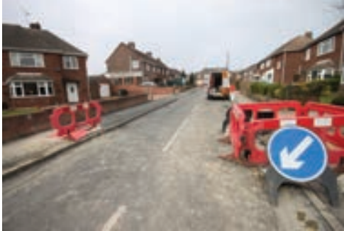
Lead Service Lines - No Road Closure
