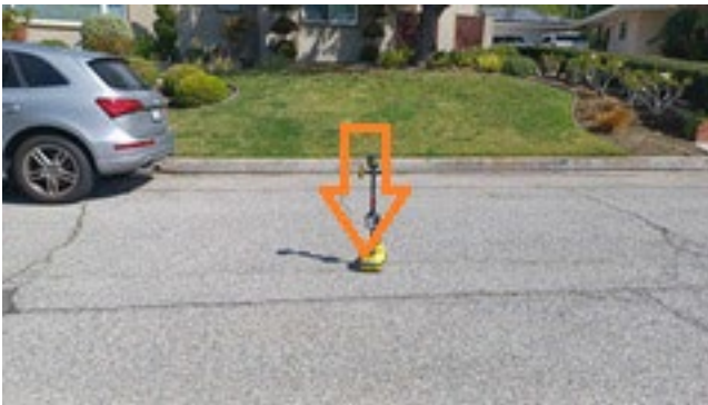
The sewer line connecting to the city sewer about 10 feet deep
