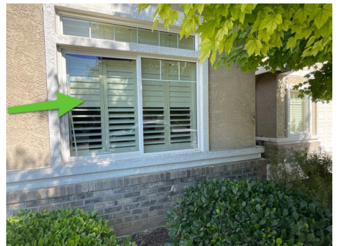
Front Wall - Left Of Entry Door
