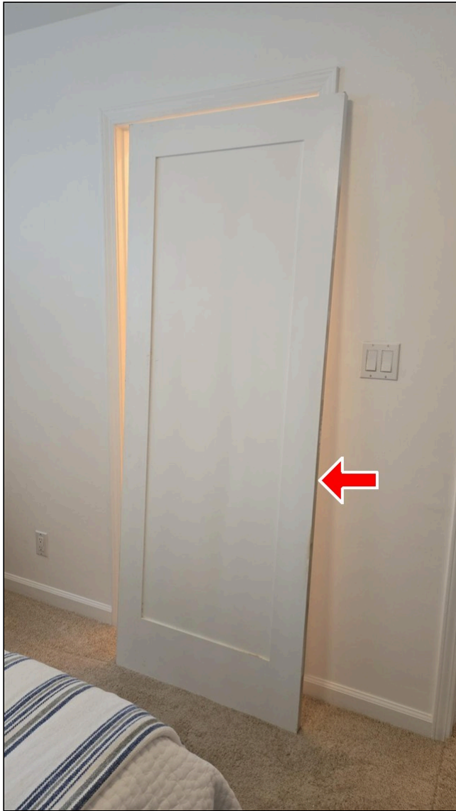
3.6 Item 3 (Picture) Lower level bedroom closet door
