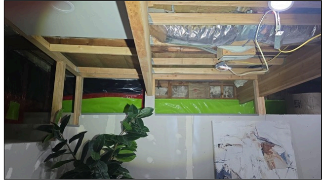
9.0 Item 2 (Picture) Foundation wall, west
