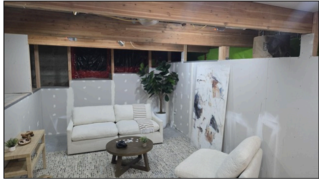
3.1 Item 4 (Picture) Basement walls, unfinished
