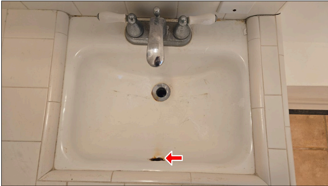
5.5 Item 1 (Picture) Lower level hall bathroom sink
