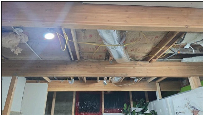
3.0 Item 1 (Picture) Unfinished ceiling, basement
