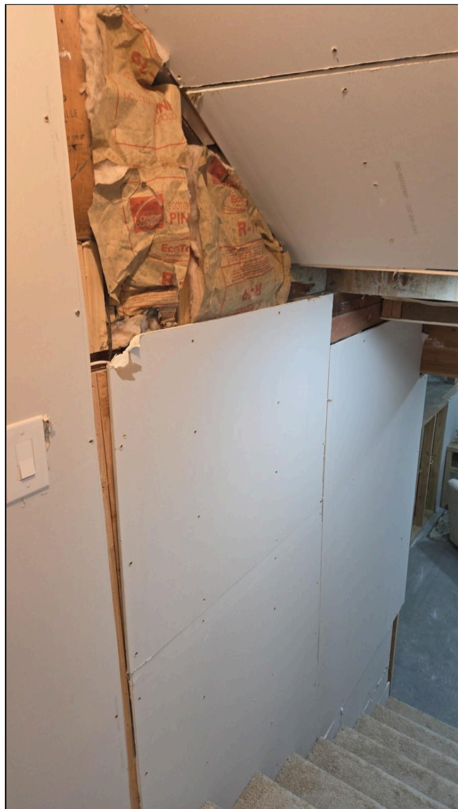
3.1 Item 1 (Picture) Basement walls, unfinished
