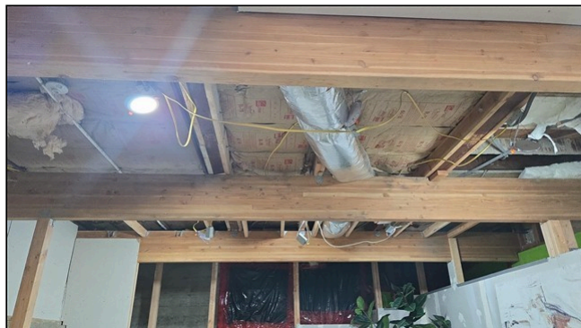
3.0 Item 1 (Picture) Unfinished ceiling, basement
