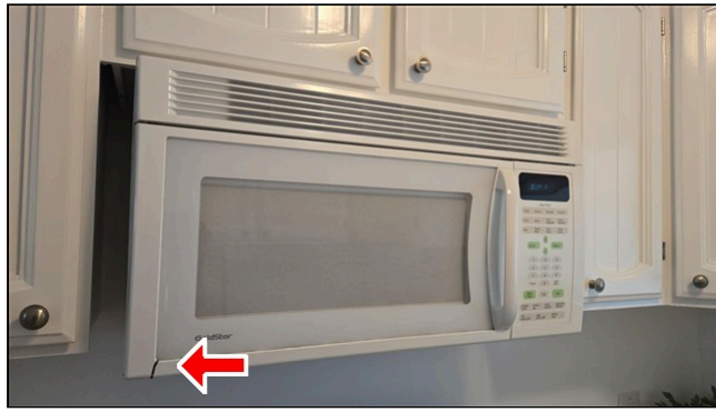
6.5 Item 1 (Picture) Built in microwave
