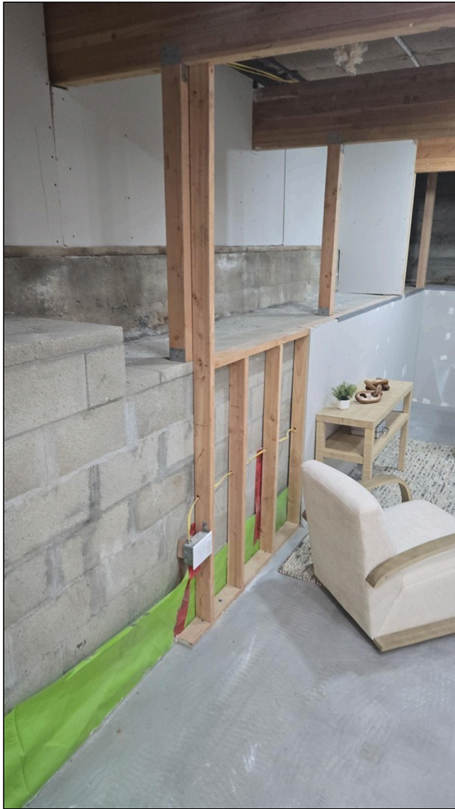
3.1 Item 3 (Picture) Basement walls, unfinished
