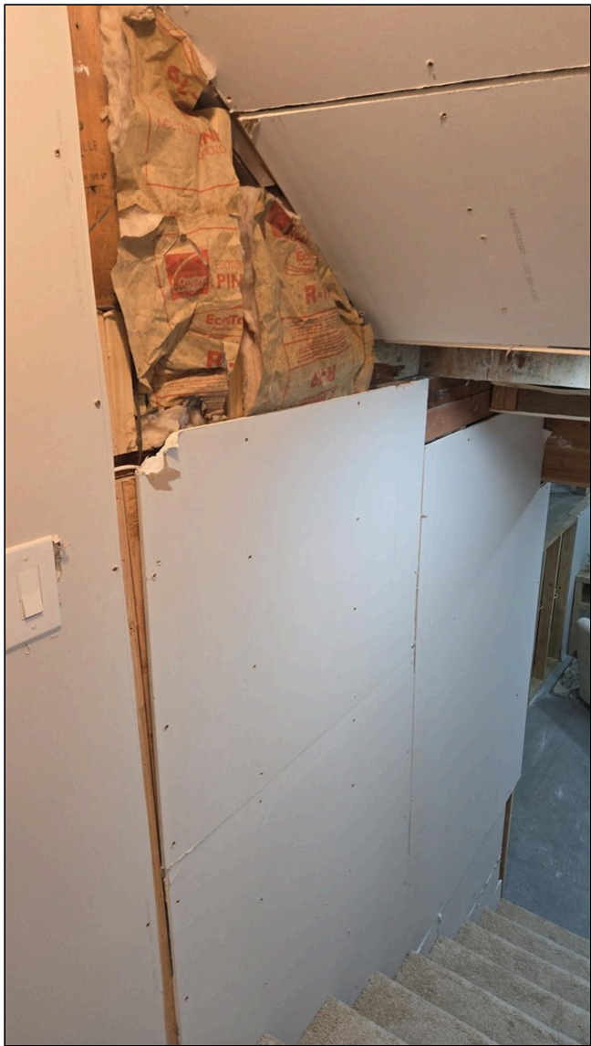
3.1 Item 1 (Picture) Basement walls, unfinished
