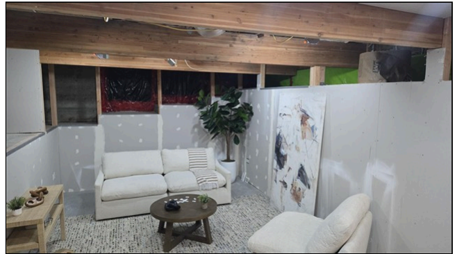
3.1 Item 4 (Picture) Basement walls, unfinished
