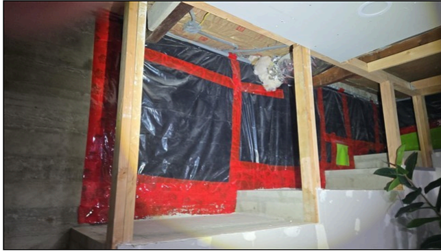
9.0 Item 1 (Picture) Foundation wall, south
