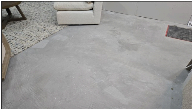
3.2 Item 4 (Picture) Basement, unfinished flooring
