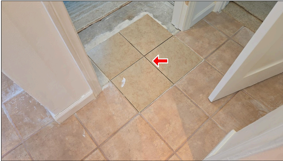
3.2 Item 3 (Picture) Lower level floor tile
