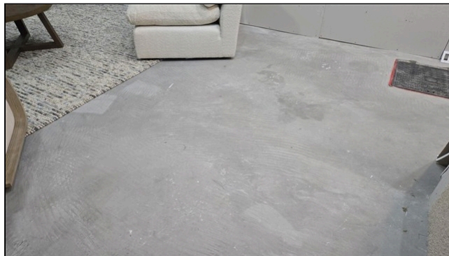
3.2 Item 4 (Picture) Basement, unfinished flooring
