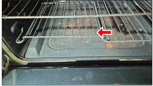
6.1 Item 2 (Picture) Oven panel, rust and deterioration
