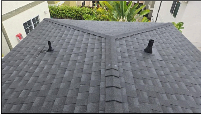
2.0 Item 3 (Picture) Roof covering
