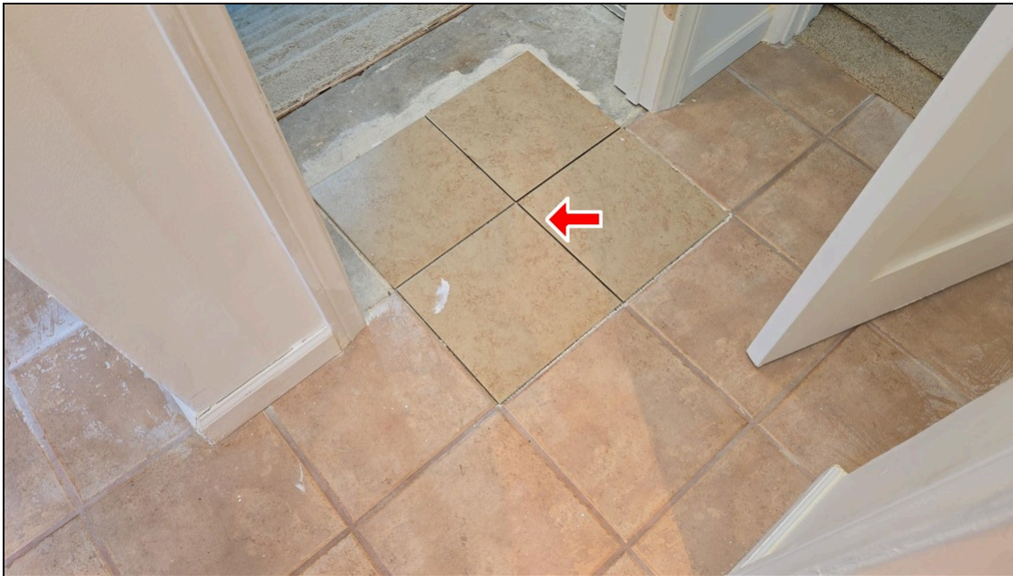
3.2 Item 3 (Picture) Lower level floor tile
