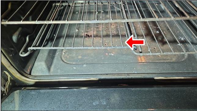
6.1 Item 2 (Picture) Oven panel, rust and deterioration
