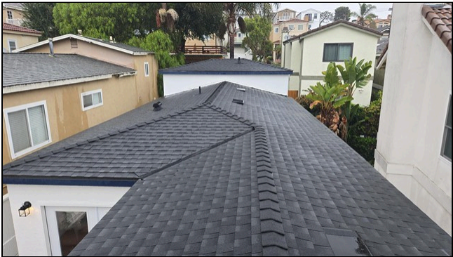
2.0 Item 1 (Picture) Roof covering
