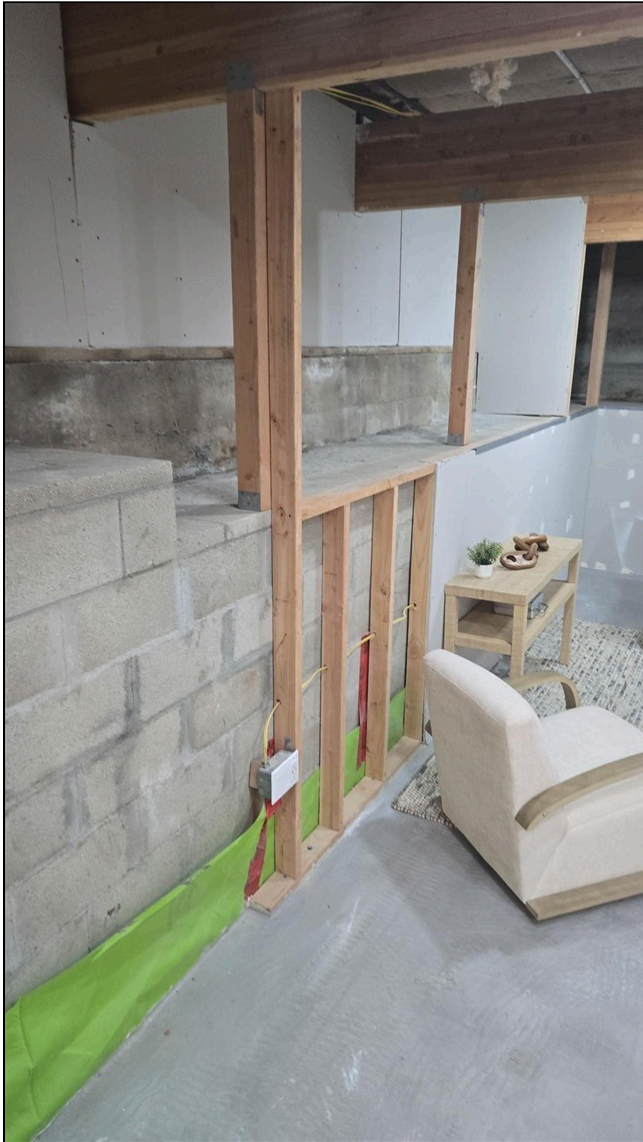
3.1 Item 3 (Picture) Basement walls, unfinished
