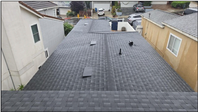
2.0 Item 2 (Picture) Roof covering
