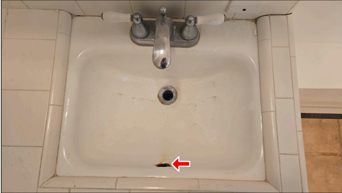
5.5 Item 1 (Picture) Lower level hall bathroom sink
