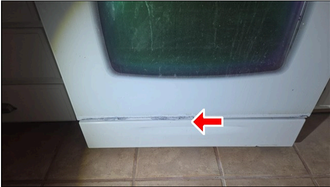
6.1 Item 1 (Picture) Oven door, rust and deterioration
