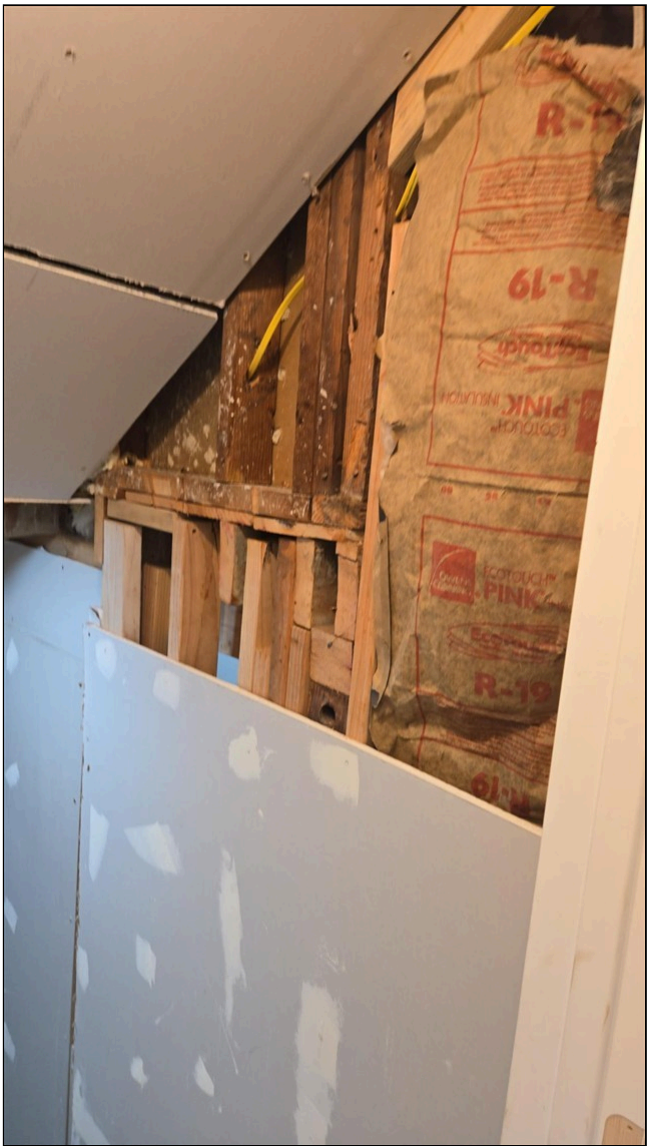
3.1 Item 2 (Picture) Basement walls, unfinished
