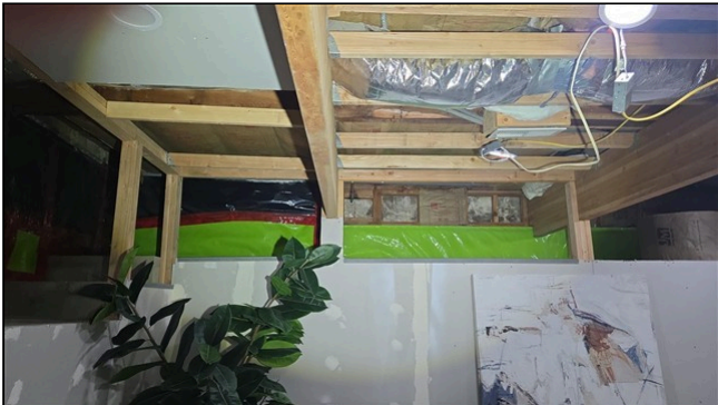
9.0 Item 2 (Picture) Foundation wall, west
