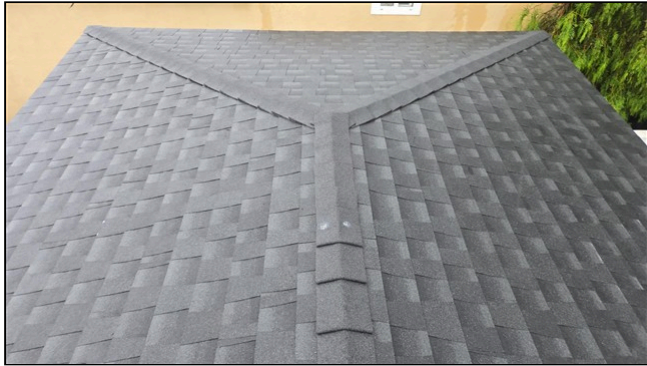
2.0 Item 4 (Picture) Roof covering
