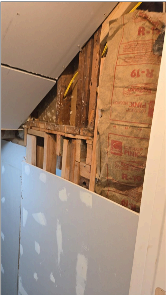
3.1 Item 2 (Picture) Basement walls, unfinished
