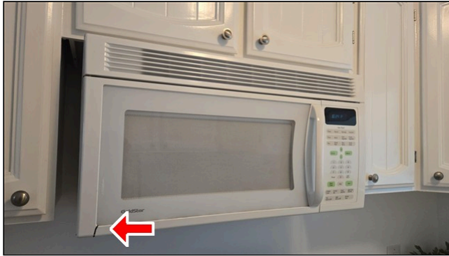
6.5 Item 1 (Picture) Built in microwave
