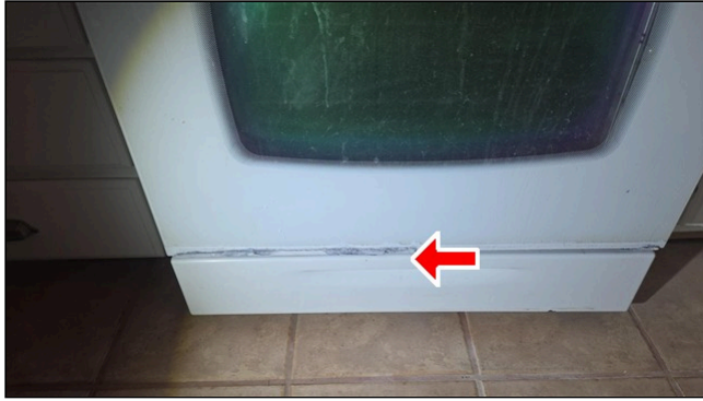
6.1 Item 1 (Picture) Oven door, rust and deterioration
