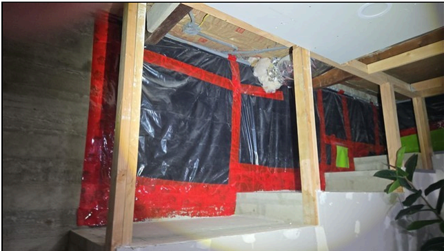
9.0 Item 1 (Picture) Foundation wall, south
