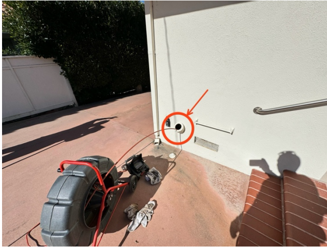
Location of 4" cleanout used for inspection.
