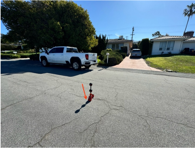
Connection to city sewer under tool 8.5' deep.
