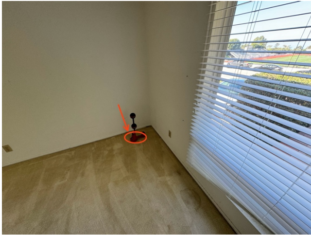
Transition from a plastic pipe to a cast iron pipe underneath the home.
