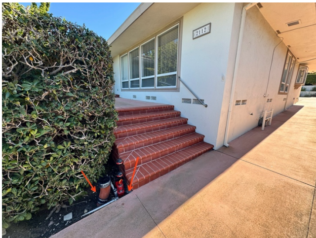
Transition from a cast iron pipe to a clay pipe 2.5' deep under tool. Location of additional sewer cleanout.
