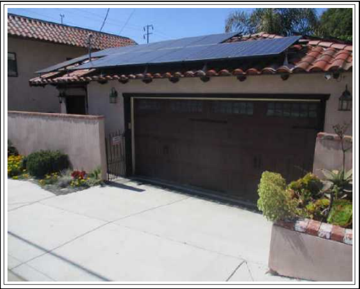
DETACHED GARAGE WITH SOLAR PANELS
