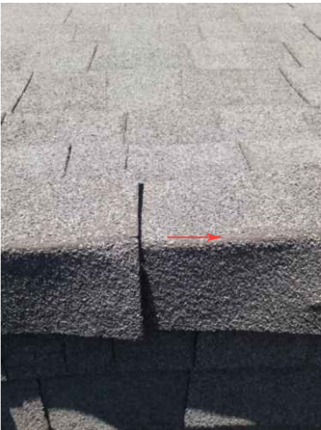
ROOF INSTALLATION Satisfactory
