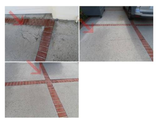
DEFECTIVE: Large crack(s). Moderate to severe cracking of pavement indicating past or present soil movement or settlement viewed. We recommend further evaluation by a licensed geotechnical engineer.
