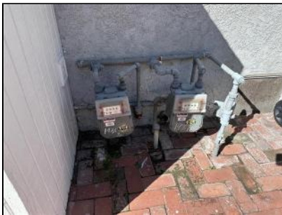
5.5 Item 2(Picture) Plumbing System
