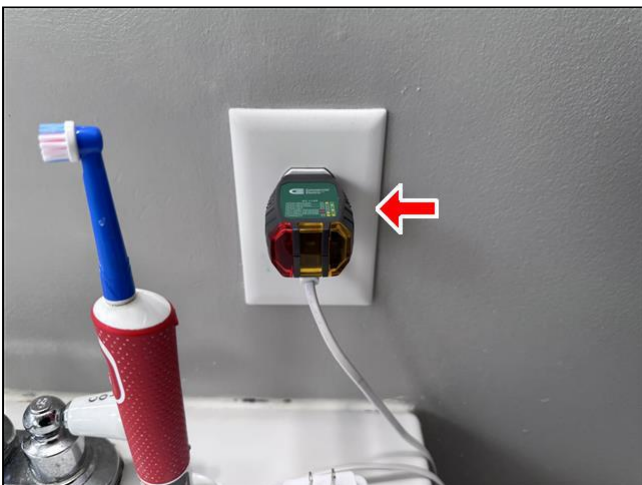
Item 60 - Item 1(Picture) Electrical System
