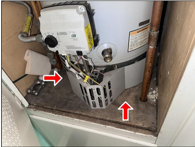
5.2 Item 3(Picture) Plumbing System
