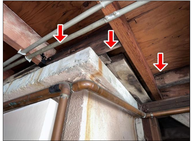
9.4 Item 2(Picture) Garage
