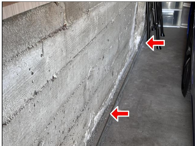
9.4 Item 15(Picture) Garage
