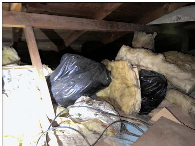
Item 63 - Item 2(Picture) Insulation & Ventilation
