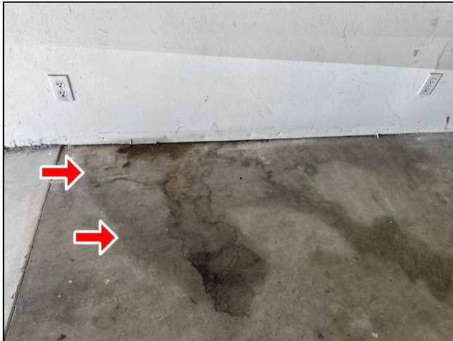
9.4 Item 5(Picture) Garage
