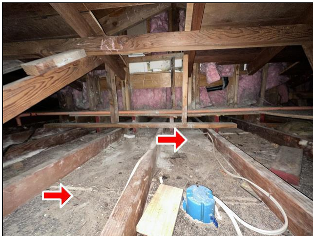
7.0 Item 1(Picture) Insulation & Ventilation
