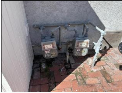
5.5 Item 1(Picture) Plumbing System
