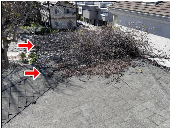
Item 2 - Item 1(Picture) Roofing
