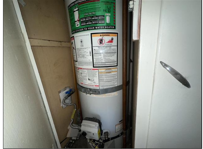
5.2 Item 6(Picture) Plumbing System
