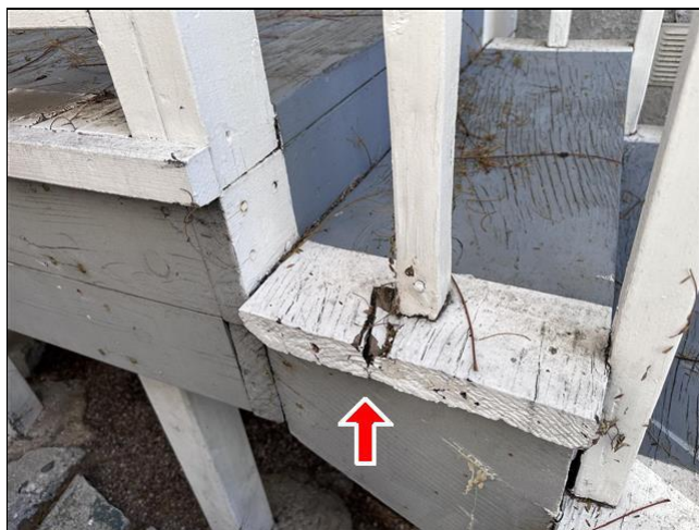
2.0 Item 4(Picture) Exterior
