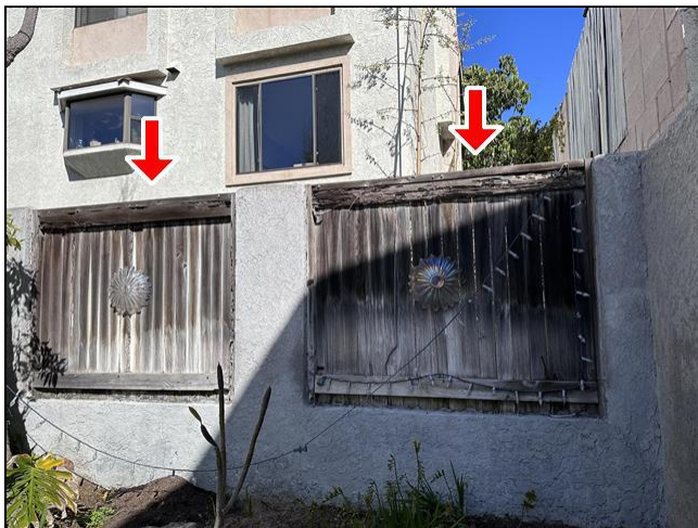
2.6 Item 1(Picture) Exterior
