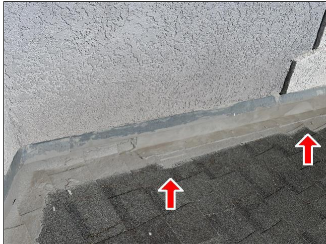
Item 1 - Item 4(Picture) Roofing
