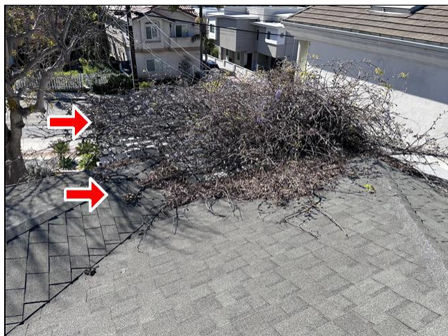
1.0 Item 10(Picture) Roofing
