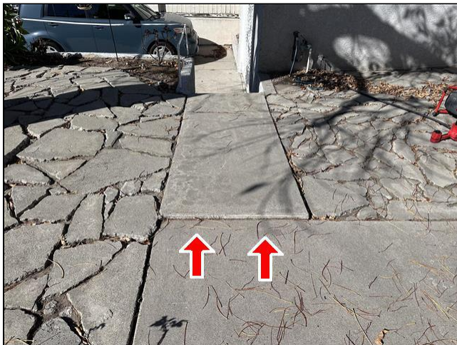
2.4 Item 1(Picture) Exterior
