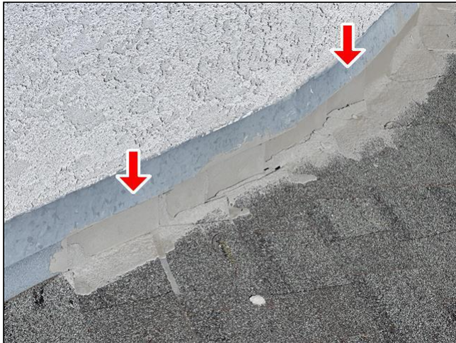
Item 1 - Item 3(Picture) Roofing
