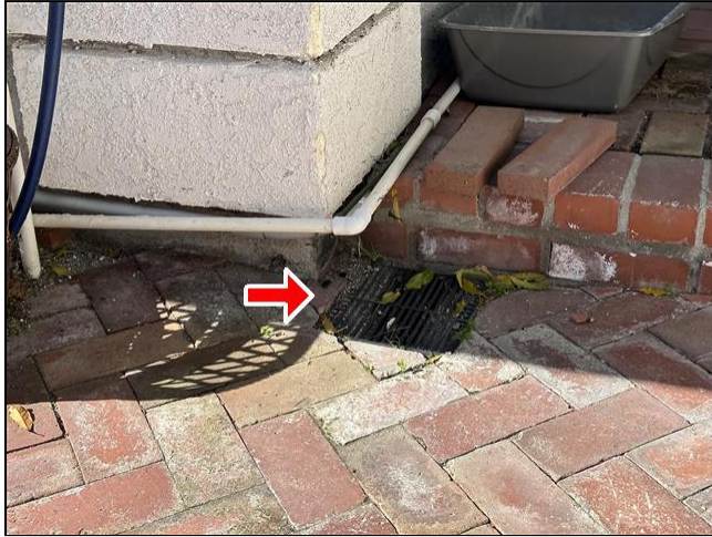
2.4 Item 10(Picture) Exterior
