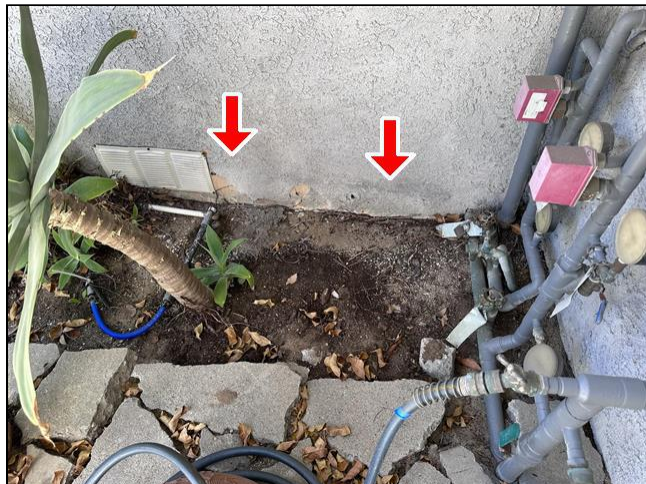
2.0 Item 8(Picture) Exterior
