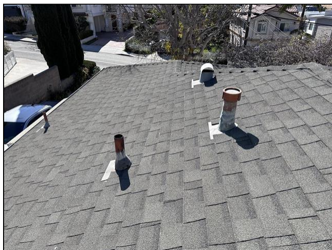
1.0 Item 9(Picture) Roofing
