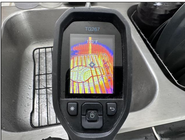
Item 49 - Item 1(Picture) Plumbing System
