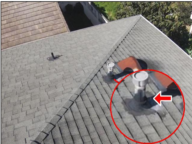
Item 6 - Item 1(Picture) Roofing
