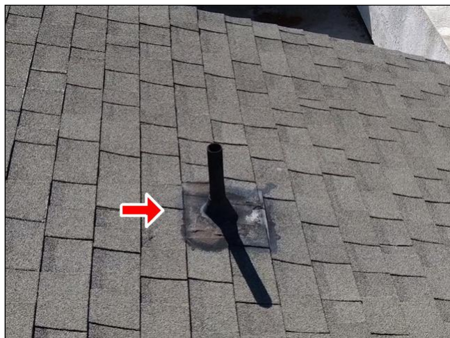
Item 3 - Item 2(Picture) Roofing
