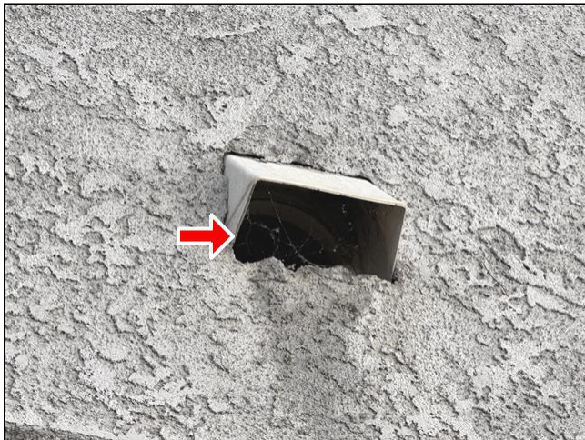
7.4 Item 2(Picture) Insulation & Ventilation
