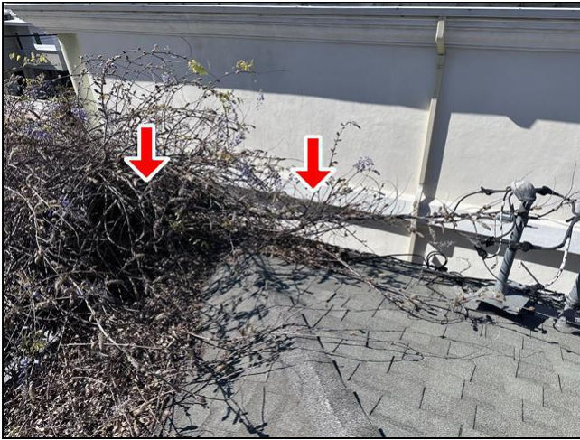
Item 53 - Item 1(Picture) Electrical System
