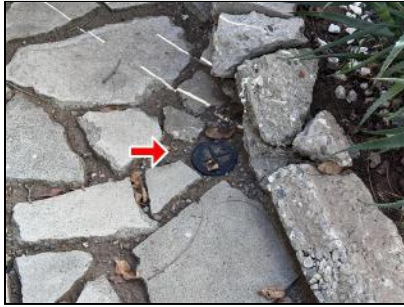
5.7 Item 1(Picture) Plumbing System
