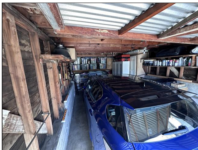
9.4 Item 16(Picture) Garage
