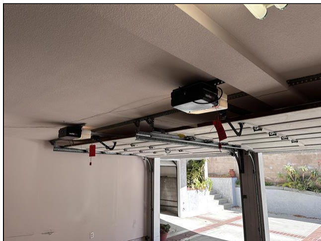
9.2 Item 1(Picture) Garage
