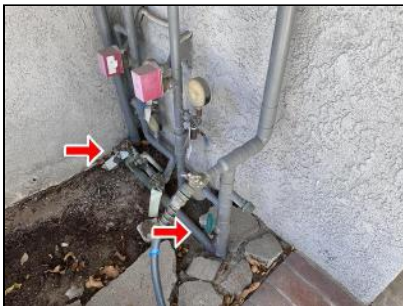
5.6 Item 1(Picture) Plumbing System
