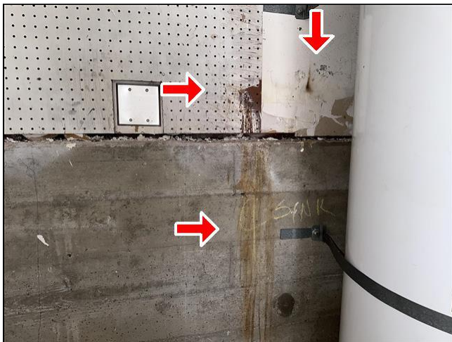
9.4 Item 9(Picture) Garage
