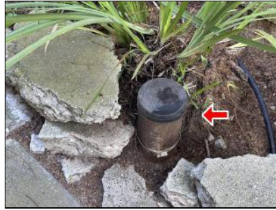
5.7 Item 2(Picture) Plumbing System
