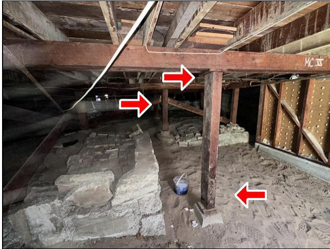
3.2 Item 3(Picture) Structural Components
