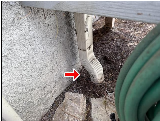
1.3 Item 2(Picture) Roofing
