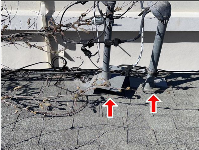
Item 4 - Item 1(Picture) Roofing
