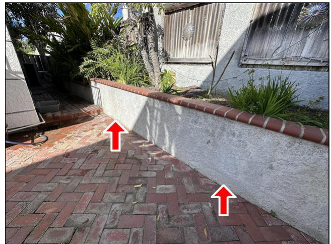
2.4 Item 9(Picture) Exterior
