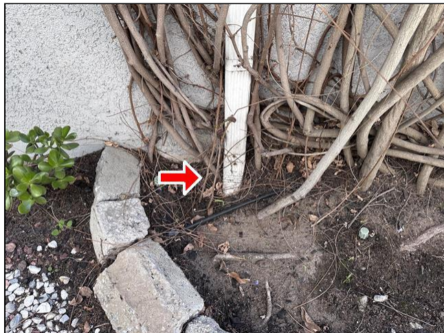
1.3 Item 1(Picture) Roofing
