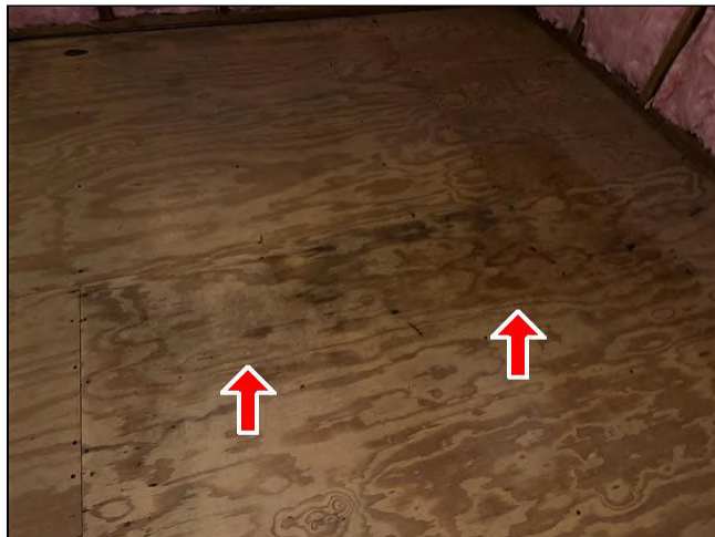
3.5 Item 5(Picture) Structural Components
