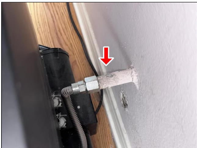
5.4 Item 2(Picture) Plumbing System
