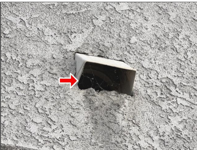
Item 65 - Item 1(Picture) Insulation & Ventilation
