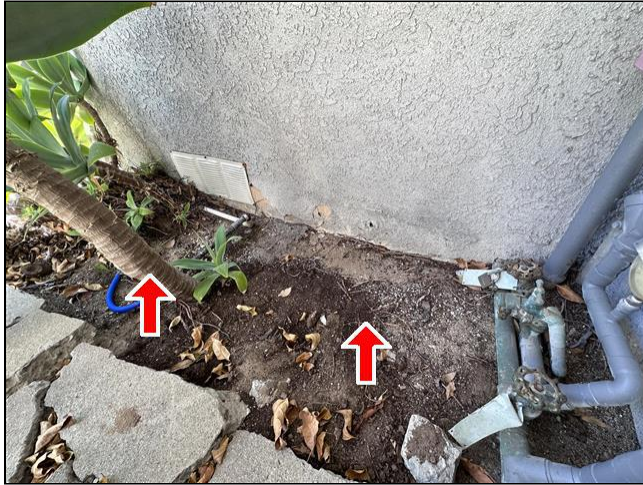
2.4 Item 7(Picture) Exterior
