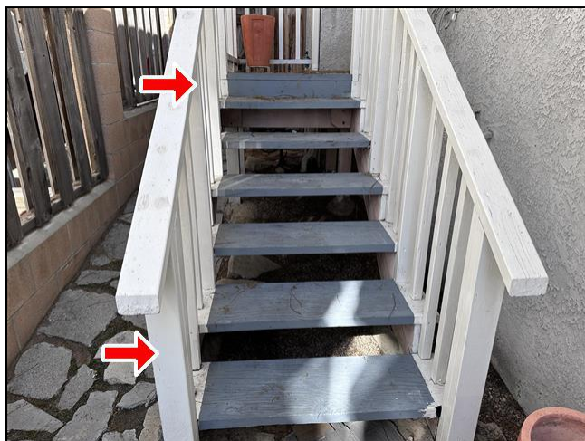
2.0 Item 3(Picture) Exterior
