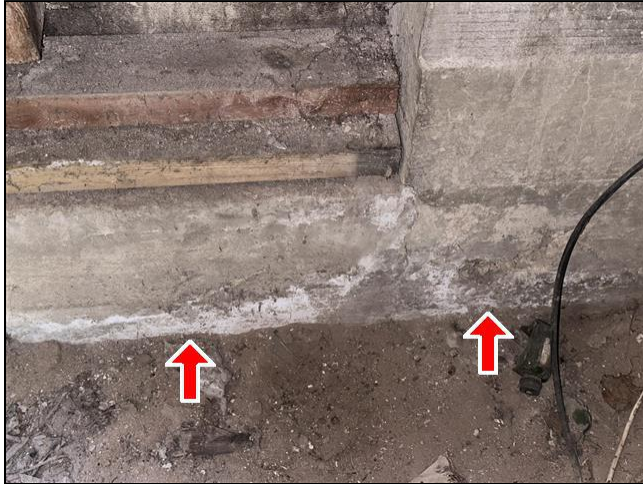
3.0 Item 2(Picture) Structural Components
