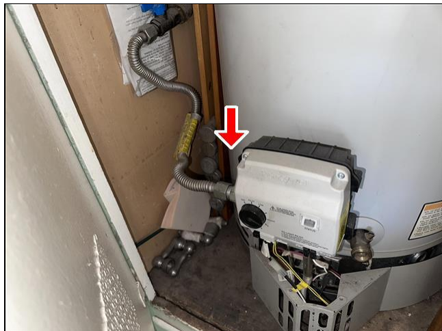
5.4 Item 3(Picture) Plumbing System
