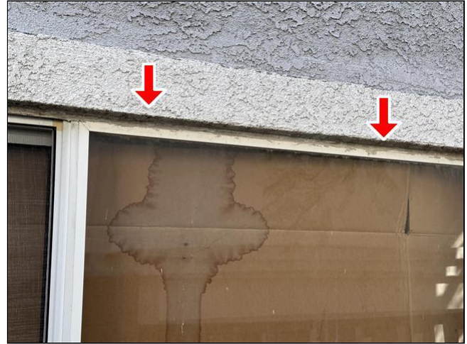
2.2 Item 2(Picture) Exterior
