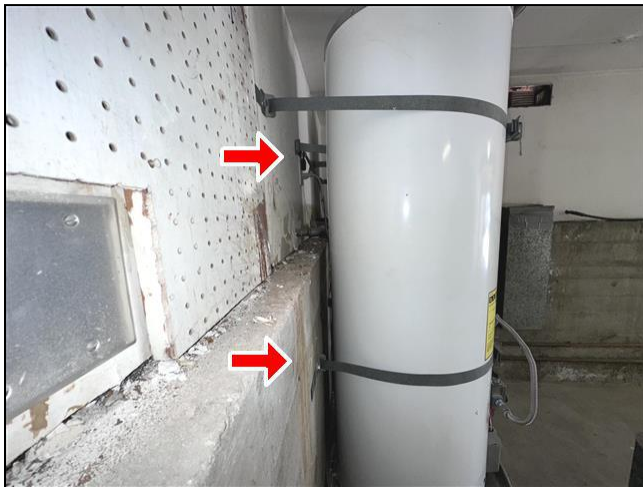
5.2 Item 4(Picture) Plumbing System
