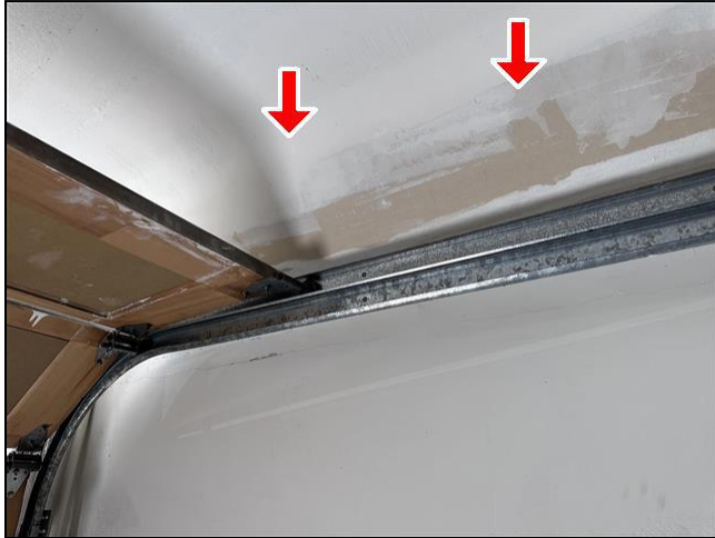
9.4 Item 3(Picture) Garage
