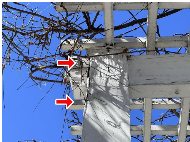
2.0 Item 6(Picture) Exterior
