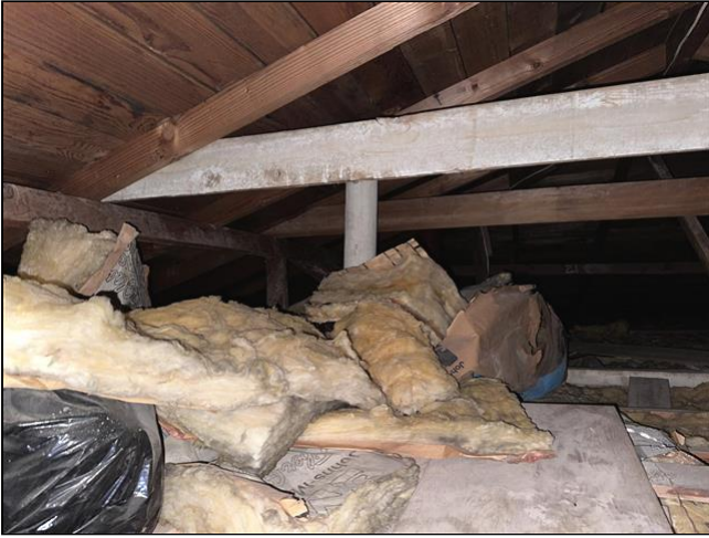
Item 63 - Item 3(Picture) Insulation & Ventilation
