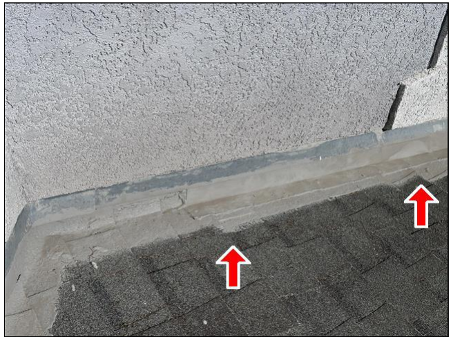
1.0 Item 4(Picture) Roofing
