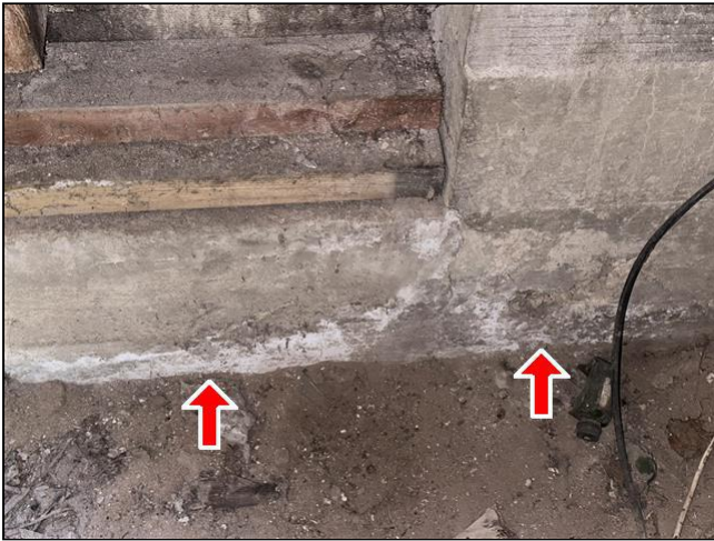
Item 25 - Item 1(Picture) Structural Components Floors/Columns/Piers
