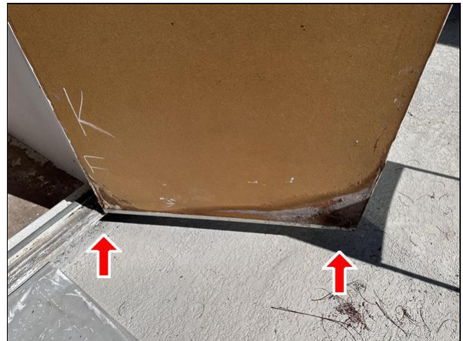
2.1 Item 2(Picture) Exterior
