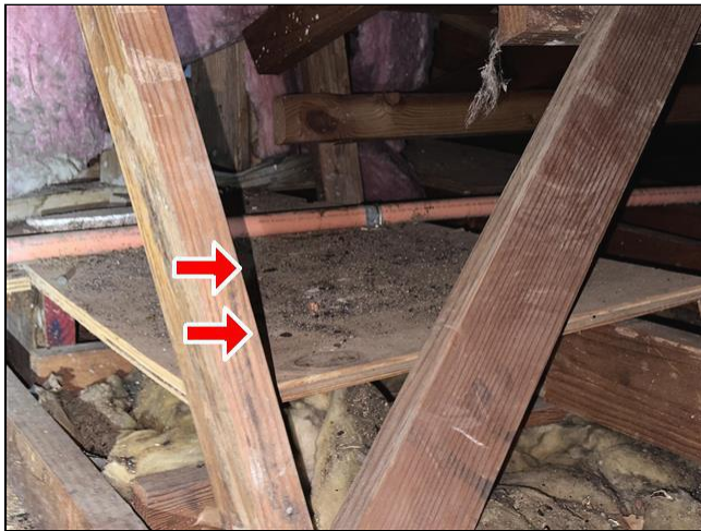
3.5 Item 1(Picture) Structural Components
