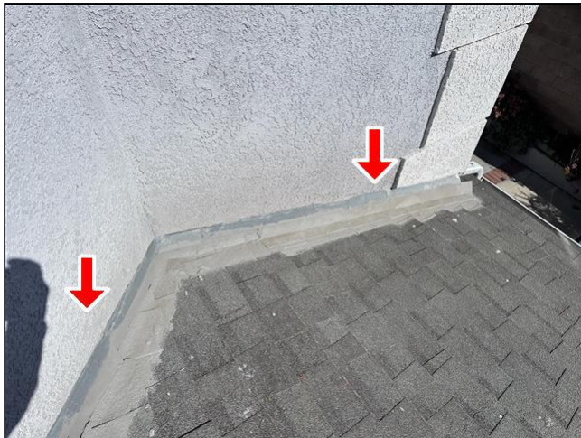
Item 1 - Item 1(Picture) Roofing
