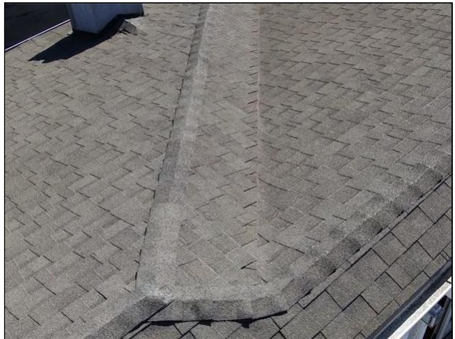
1.0 Item 6(Picture) Roofing
