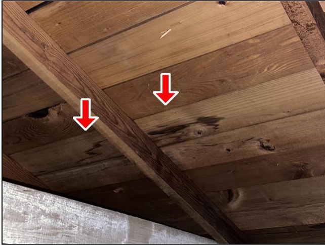
3.5 Item 2(Picture) Structural Components
