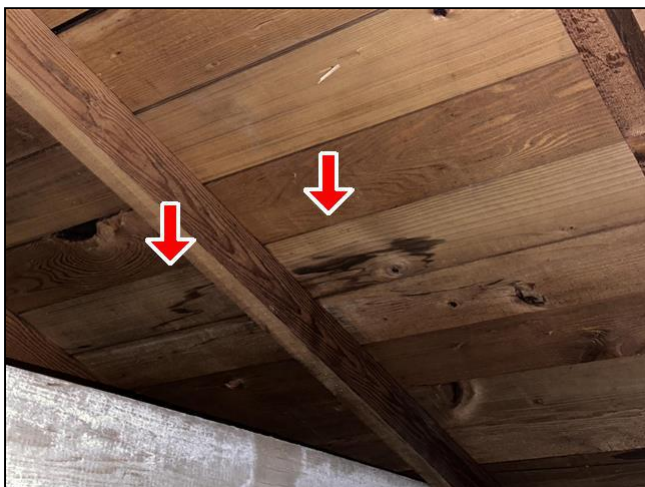
Item 29 - Item 1(Picture) Structural Components
