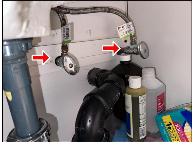
5.1 Item 4(Picture) Plumbing System
