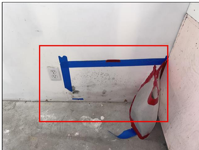
9.4 Item 14(Picture) Garage
