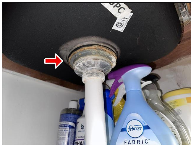
5.0 Item 1(Picture) Plumbing System
