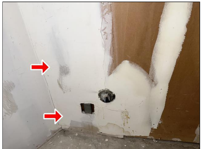
9.4 Item 10(Picture) Garage
