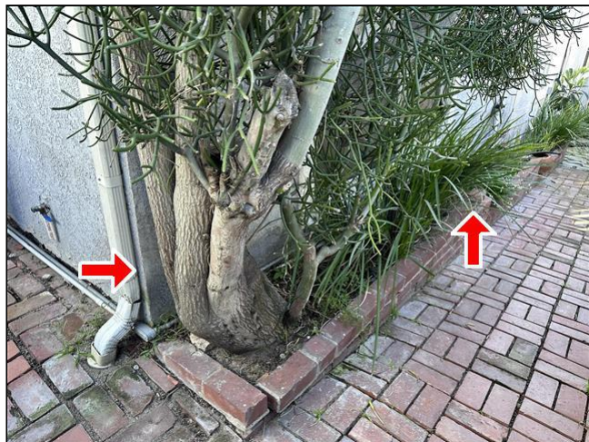
Item 13 - Item 2(Picture) Exterior
