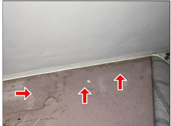
9.4 Item 13(Picture) Garage
