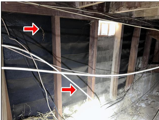
3.0 Item 1(Picture) Structural Components
