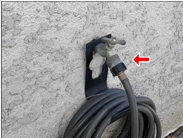
5.1 Item 5(Picture) Plumbing System
