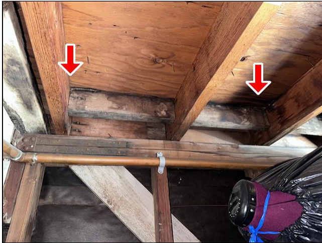
9.4 Item 1(Picture) Garage
