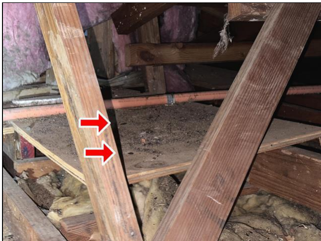
Item 28 - Item 1(Picture) Structural Components
