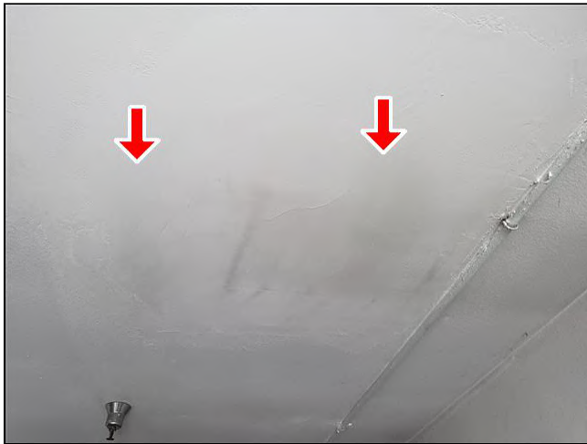
9.4 Item 7(Picture) Garage
