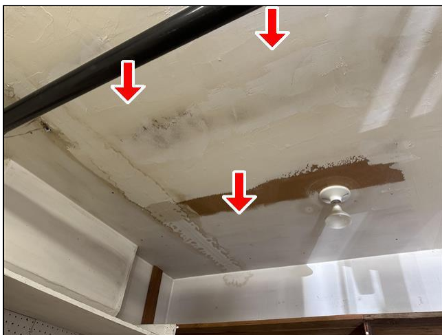
9.4 Item 11(Picture) Garage
