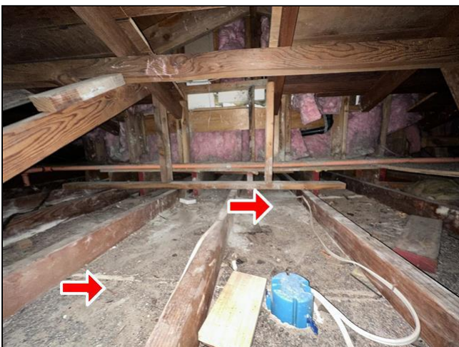
Item 63 - Item 1(Picture) Insulation & Ventilation
