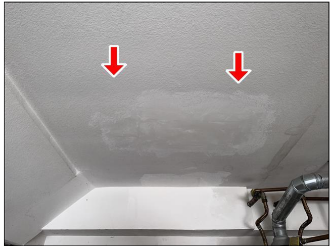
9.4 Item 8(Picture) Garage
