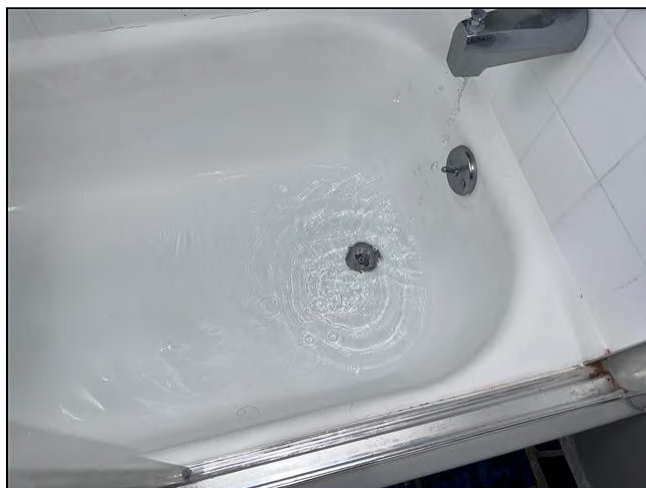
5.0 Item 2(Picture) Plumbing System
