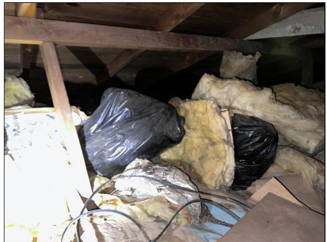
7.0 Item 2(Picture) Insulation & Ventilation
