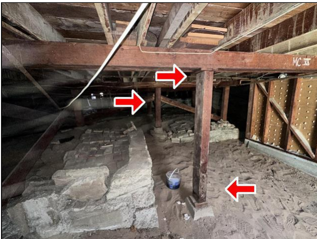
Item 27 - Item 1(Picture) Structural Components
