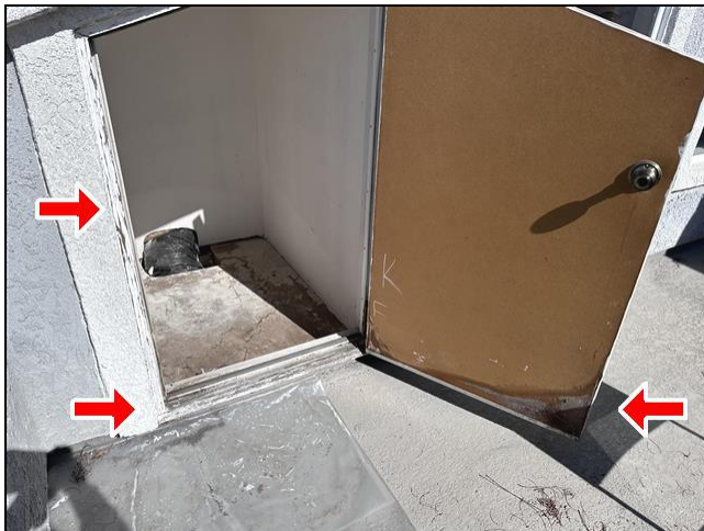
2.1 Item 1(Picture) Exterior
