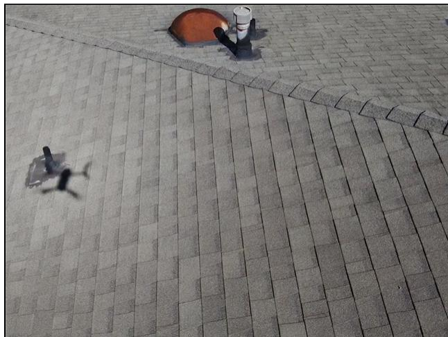
1.0 Item 7(Picture) Roofing
