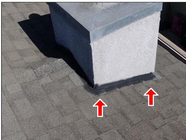
Item 3 - Item 1(Picture) Roofing Flashings/Vents
