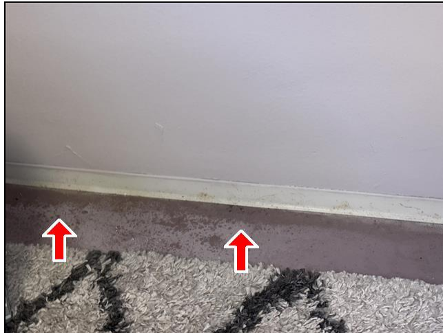
9.4 Item 12(Picture) Garage
