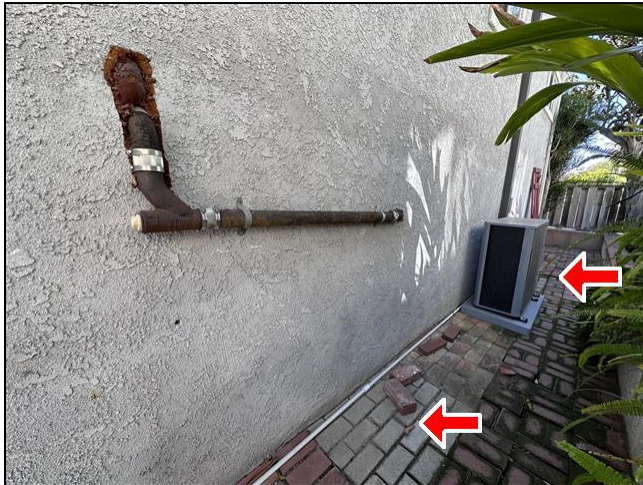
2.4 Item 3(Picture) Exterior
