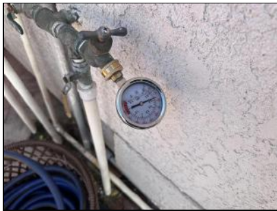
5.8 Item 1(Picture) Plumbing System
