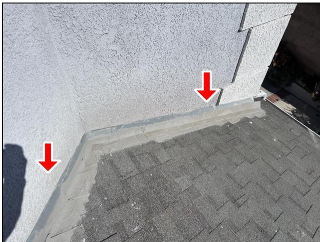
1.0 Item 1(Picture) Roofing
