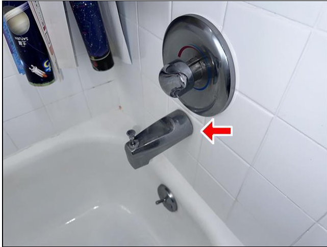
5.1 Item 3(Picture) Plumbing System
