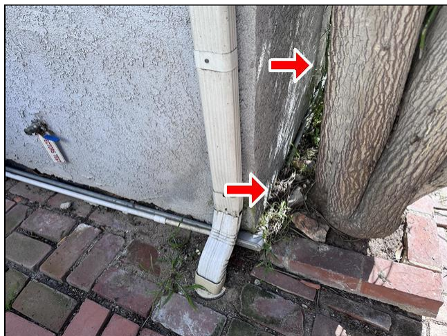
2.4 Item 6(Picture) Exterior
