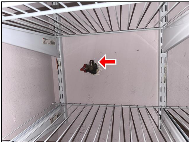
5.4 Item 1(Picture) Plumbing System
