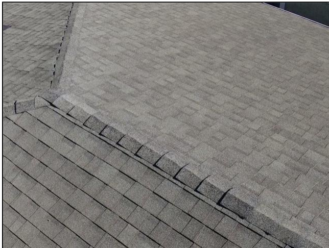
1.0 Item 5(Picture) Roofing
