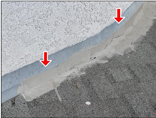
1.0 Item 3(Picture) Roofing
