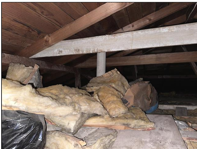
7.0 Item 3(Picture) Insulation & Ventilation
