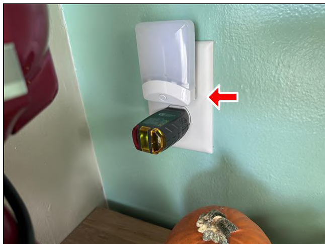
6.2 Item 2(Picture) Electrical System
