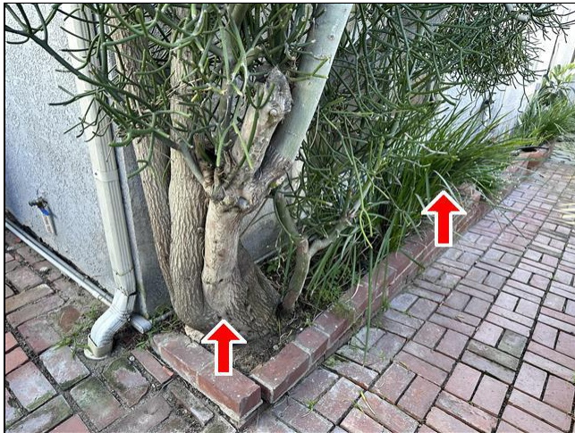
2.0 Item 12(Picture) Exterior
