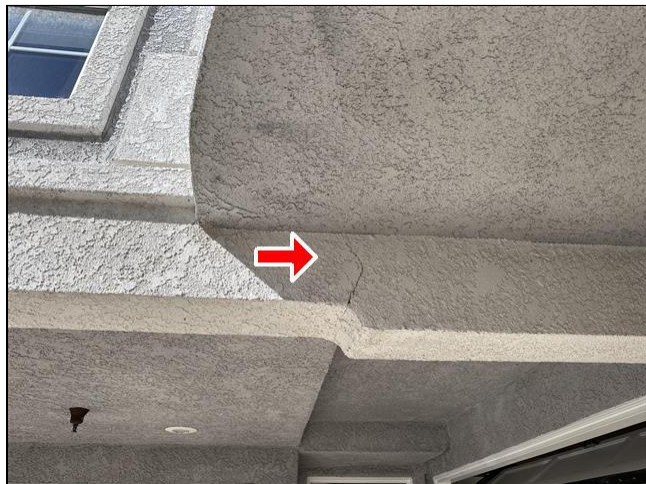
2.0 Item 1(Picture) Exterior
