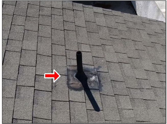
1.0 Item 12(Picture) Roofing
