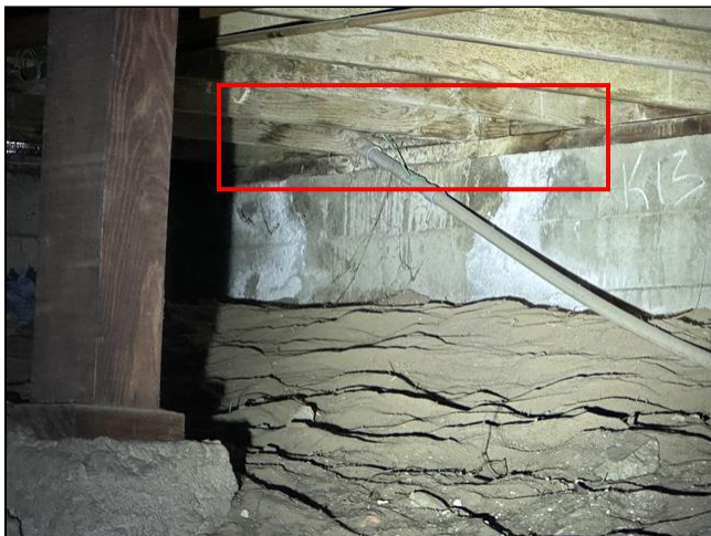
3.2 Item 1(Picture) Structural Components
