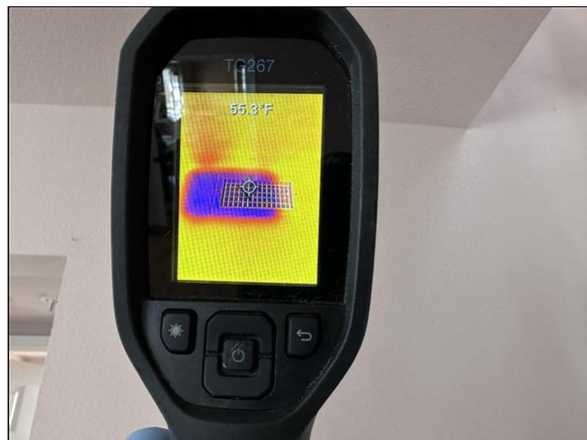
Item 36 - Item 4(Picture) Heating/Central Air
