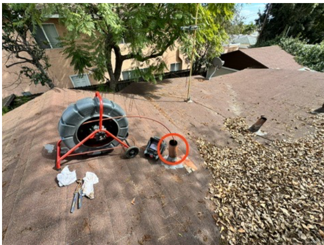
4" roof vent used for inspection.
