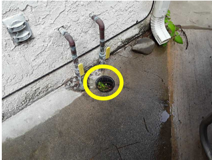
A clean-out is located at the rear.
