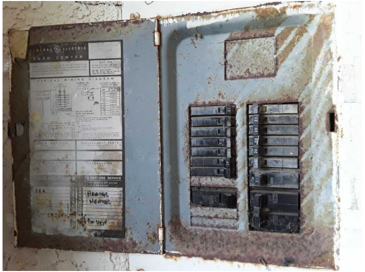
Various circuits within the sub-panel are not labeled, and should be serviced by an electrician so that the appropriate load calculations and breaker sizes could be determined.
